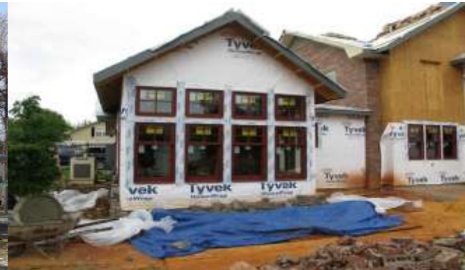
an addition to an existing dwelling
