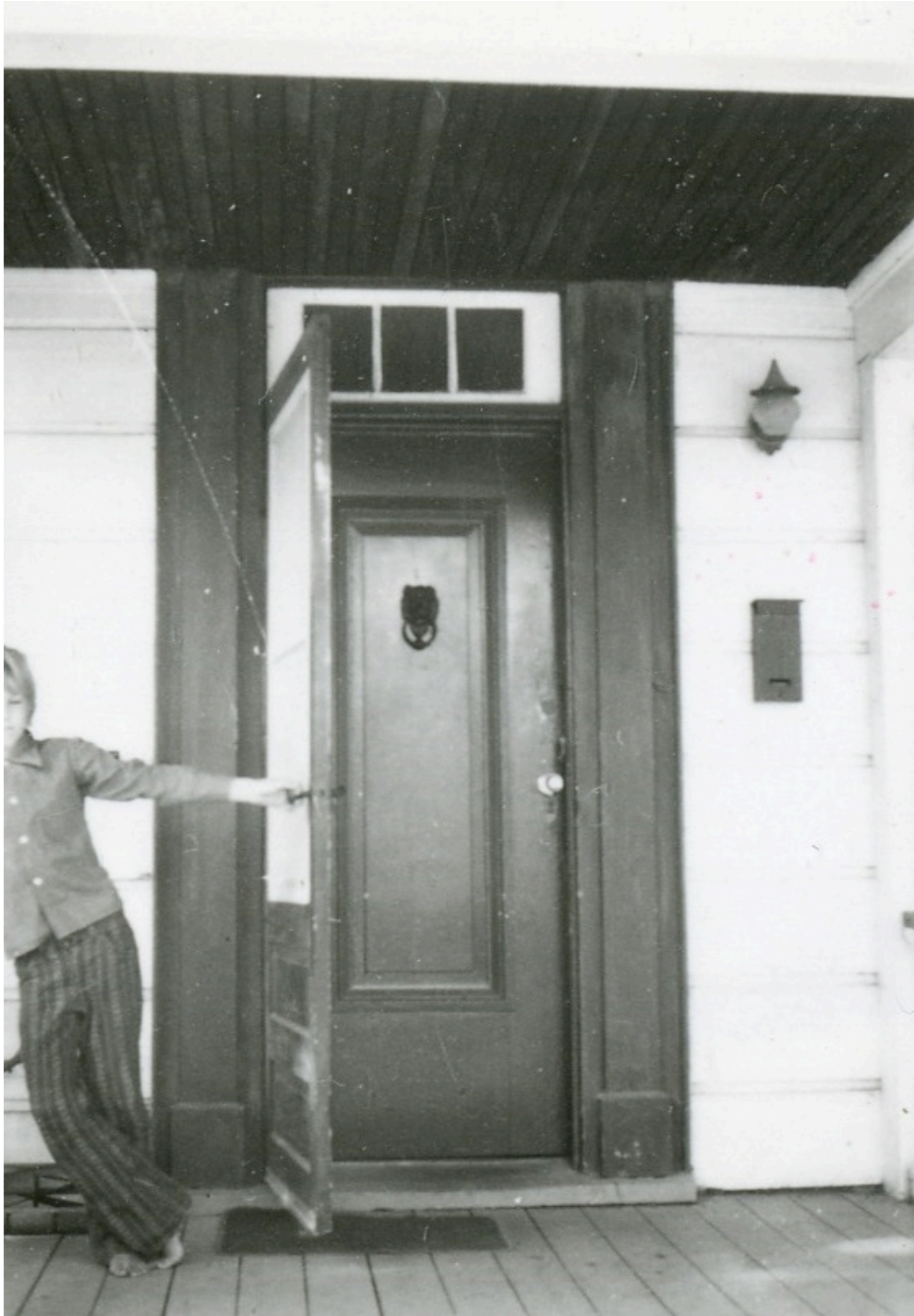
Front entrance facing Thomas Street
