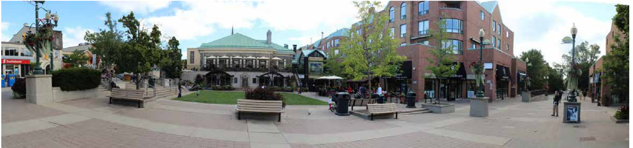
Towne Square in 2014. The fixtures, finishes and furnishings are dated and in a poor state of repair
