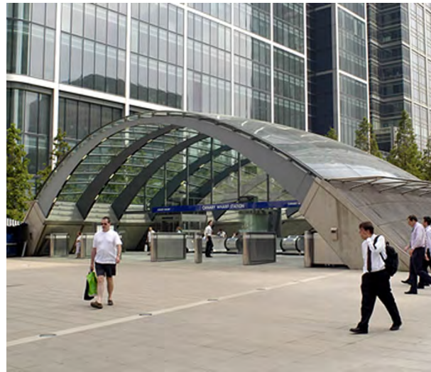
Tunnel entrance, Canary Wharf, London, UK
