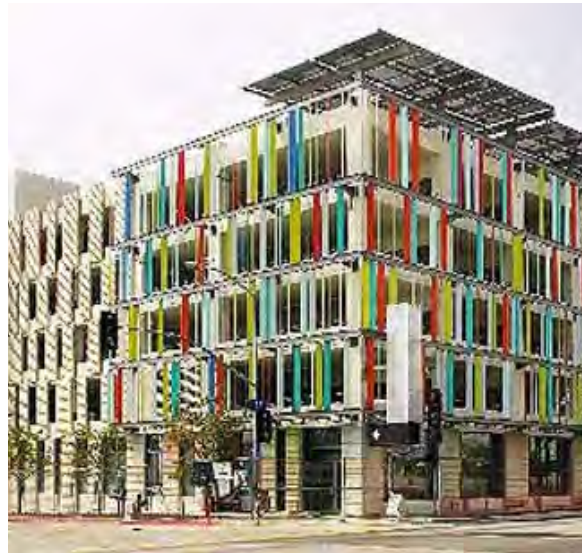
Civic Center Parking Structure, Santa Monica
