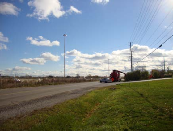
Plate 25: View south of North Service Road East ROW. ROW is disturbed. No potential.
