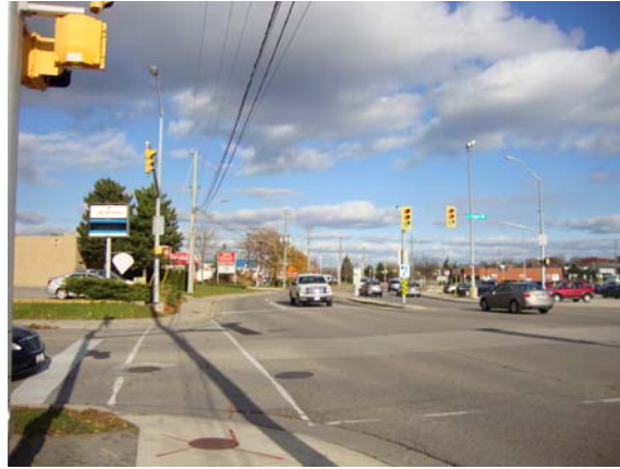
Plate 2: View northeast of Cross Avenue ROW. ROW and adjacent lands are disturbed. No potential.
