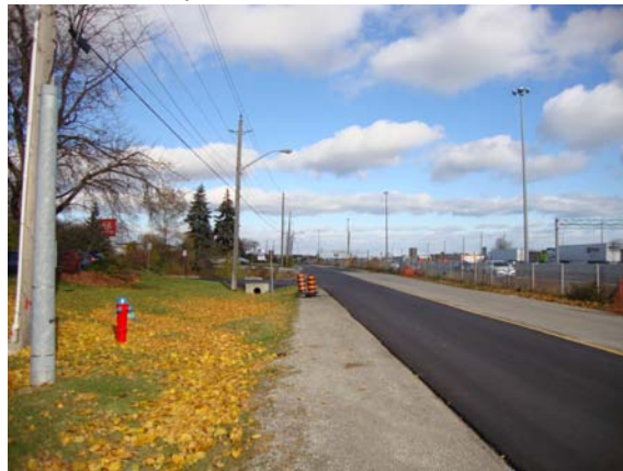
Plate 18: View northeast of North Service Road East ROW. ROW and lands beyond ROW are disturbed. No potential.
