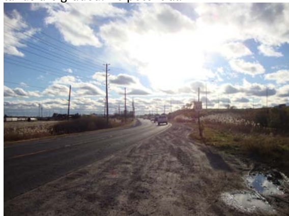
Plate 24: View SSW of South Service Road East ROW. ROW is disturbed. No potential.
