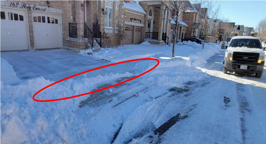
Leftover windrow from clearing
