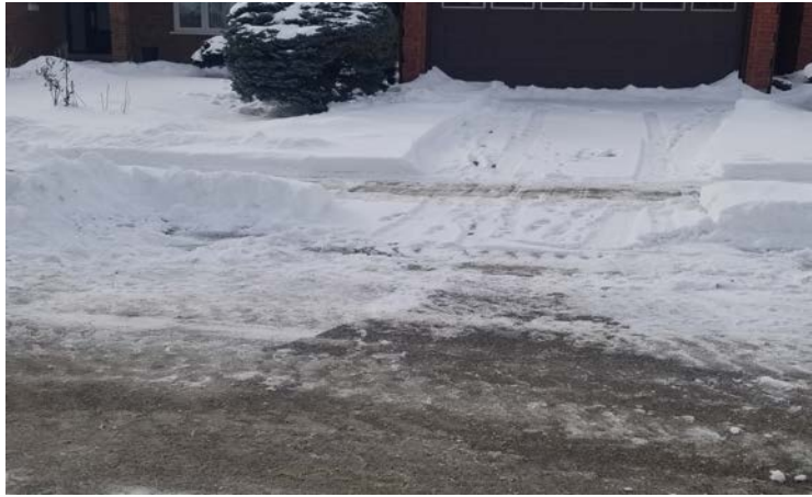
Not bare pavement
