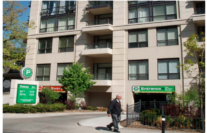
Image 34. Public parking garage in a private condominium, Toronto, Canada
