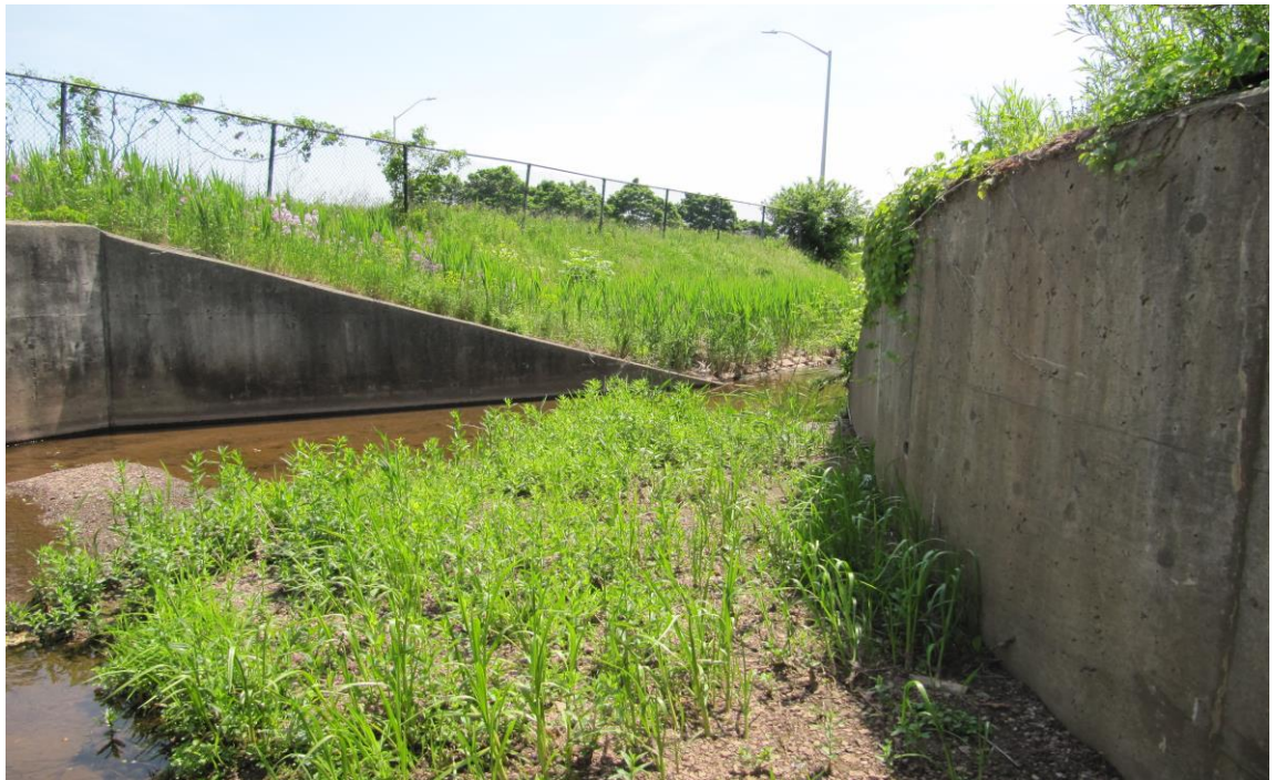
South-West Retaining Wall
