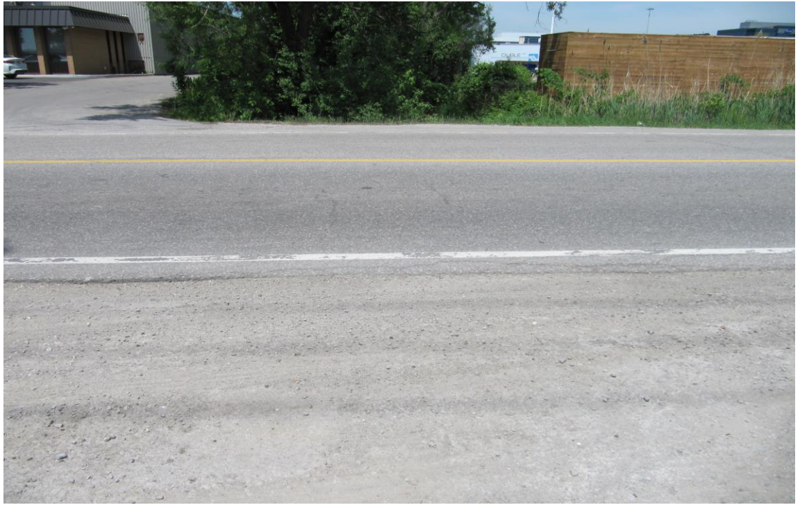
Existing Condition of Wearing Surface
