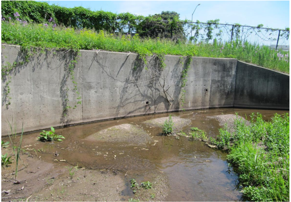
South-East Retaining Wall
