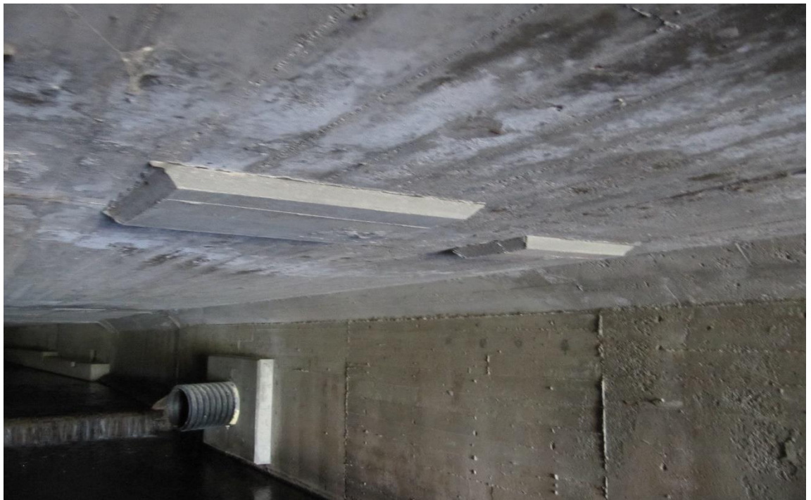
Patched Concrete Repairs for the South Extension Section of the Culvert
