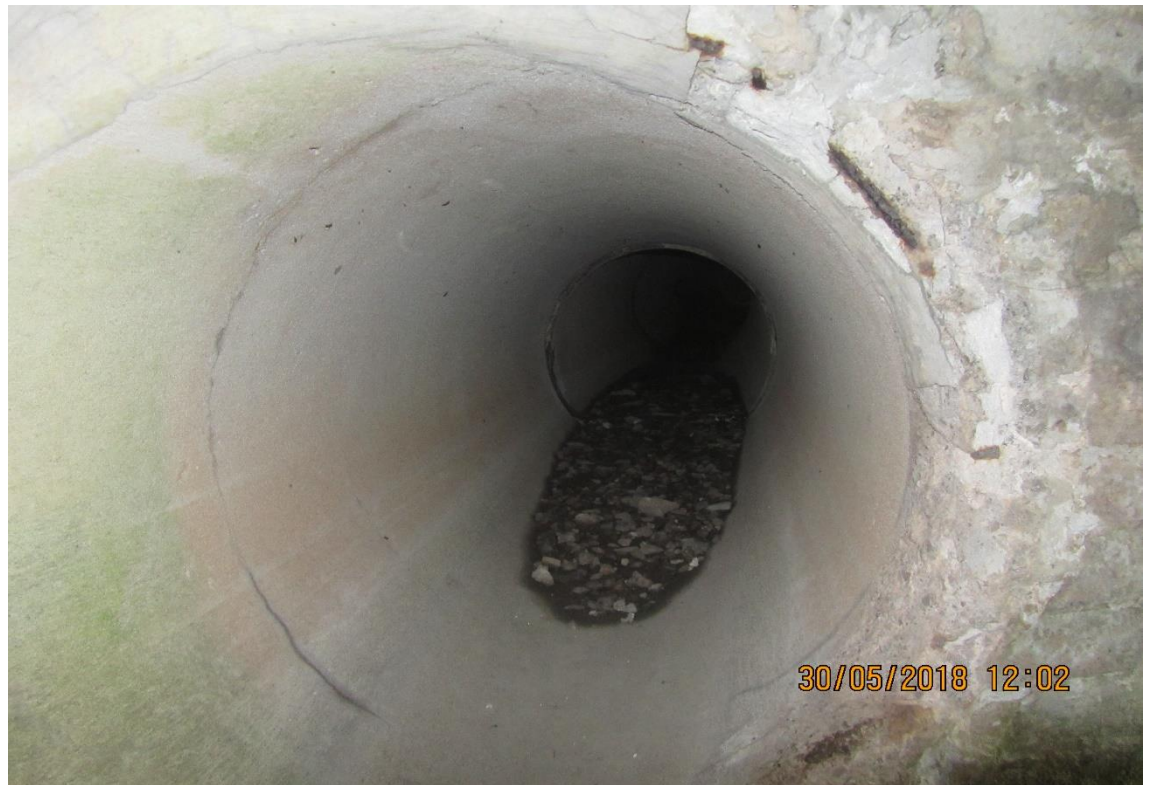
Condition of Existing Stormwater Sewer
