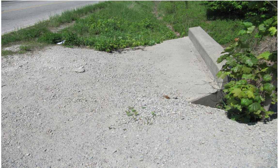
Existing Surface Condition of the Top Slab
