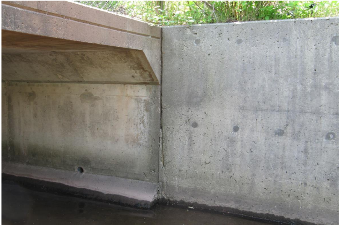
North-West Retaining Wall
