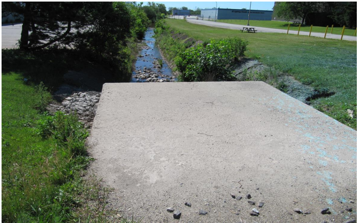
Existing Surface Condition of the Top Slab
