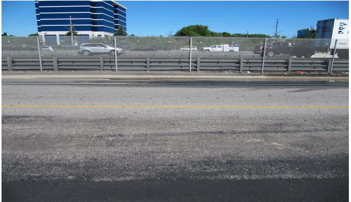
Existing Condition of Wearing Surface
