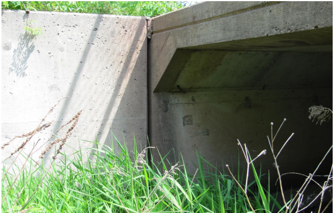
North-East Retaining Wall
