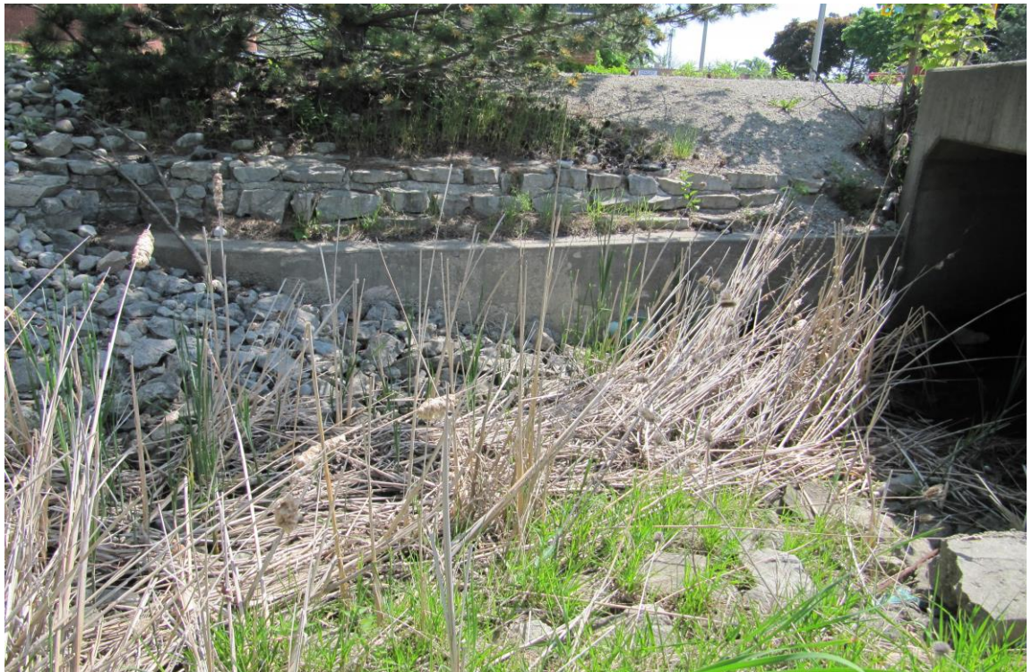
North-East Retaining Wall
