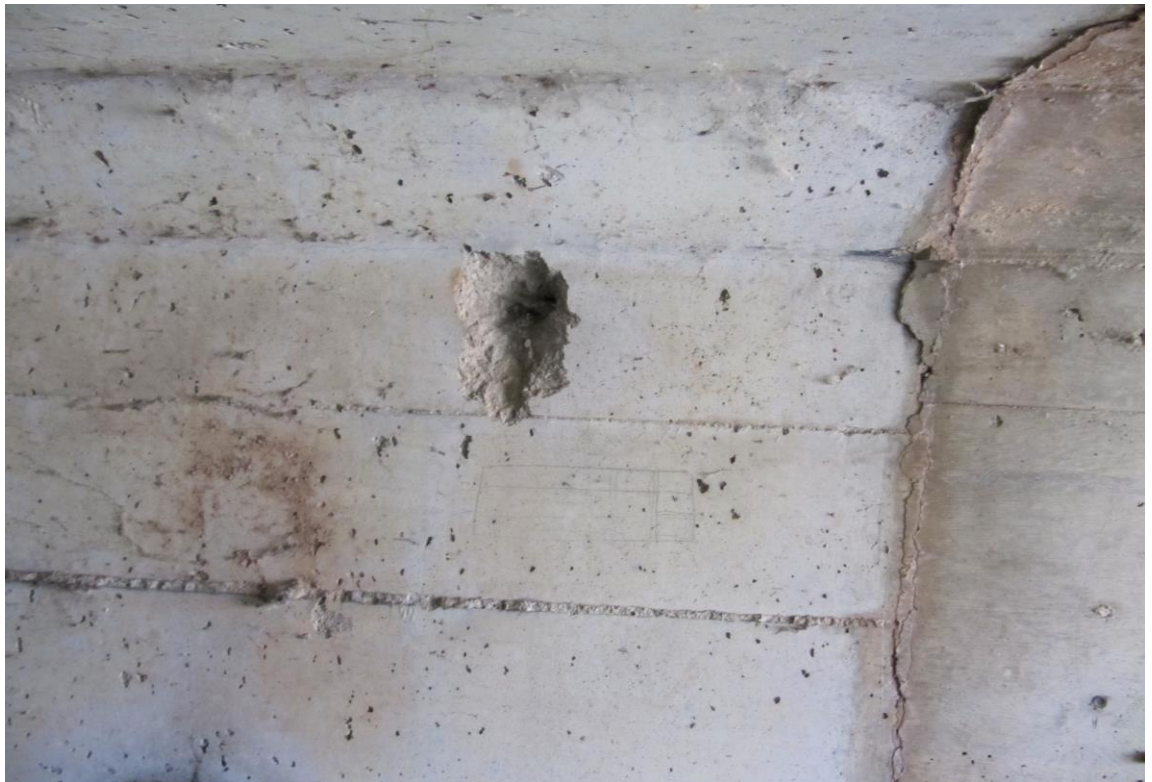
Spalled Concrete
