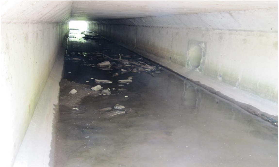
East Cell Looking South
