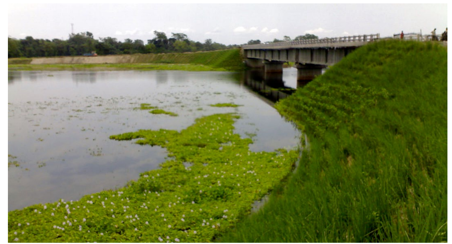
Bank stabilization planting
