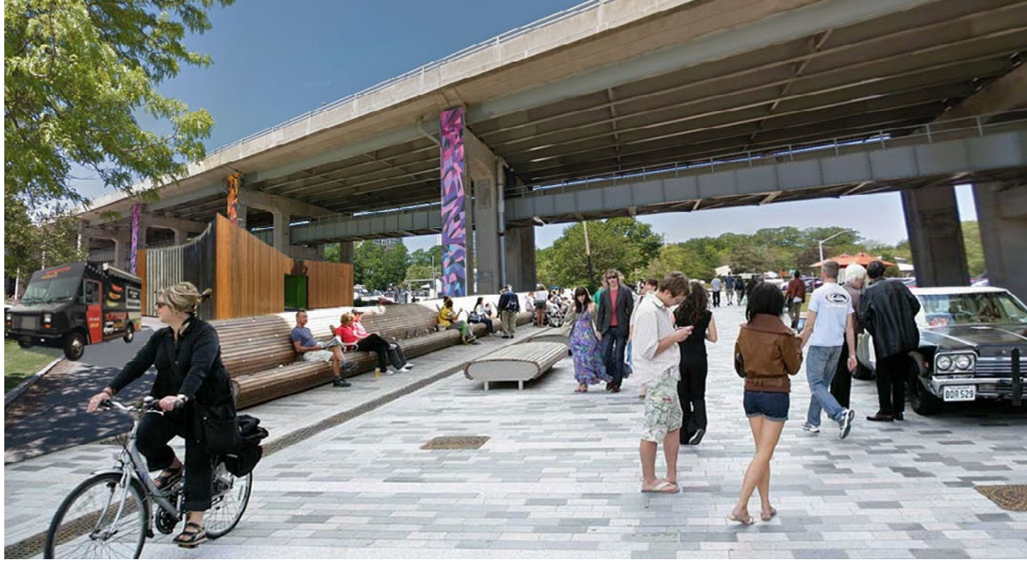
Potential improvements under the Rebecca Street bridge
