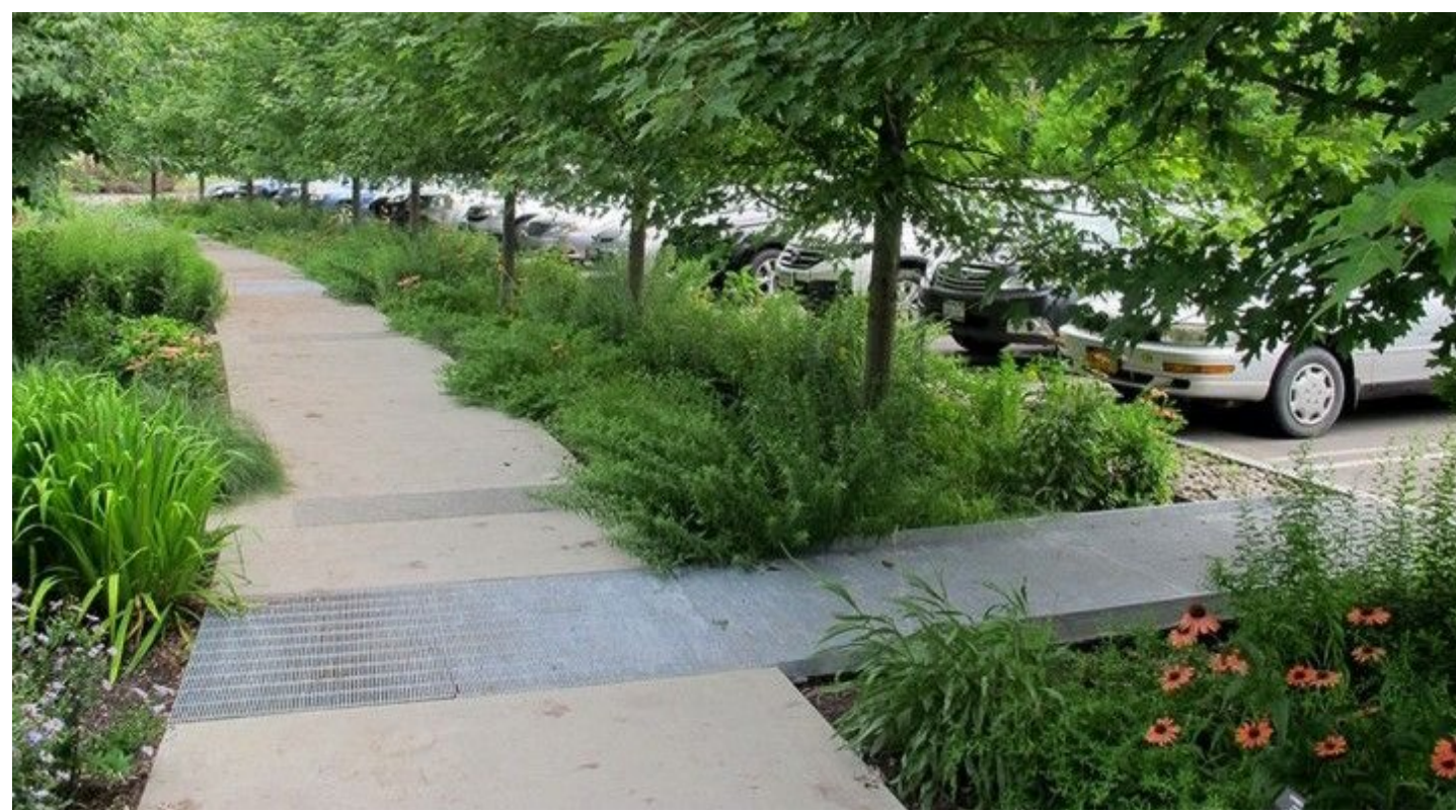
Parking lot with bio-swale
