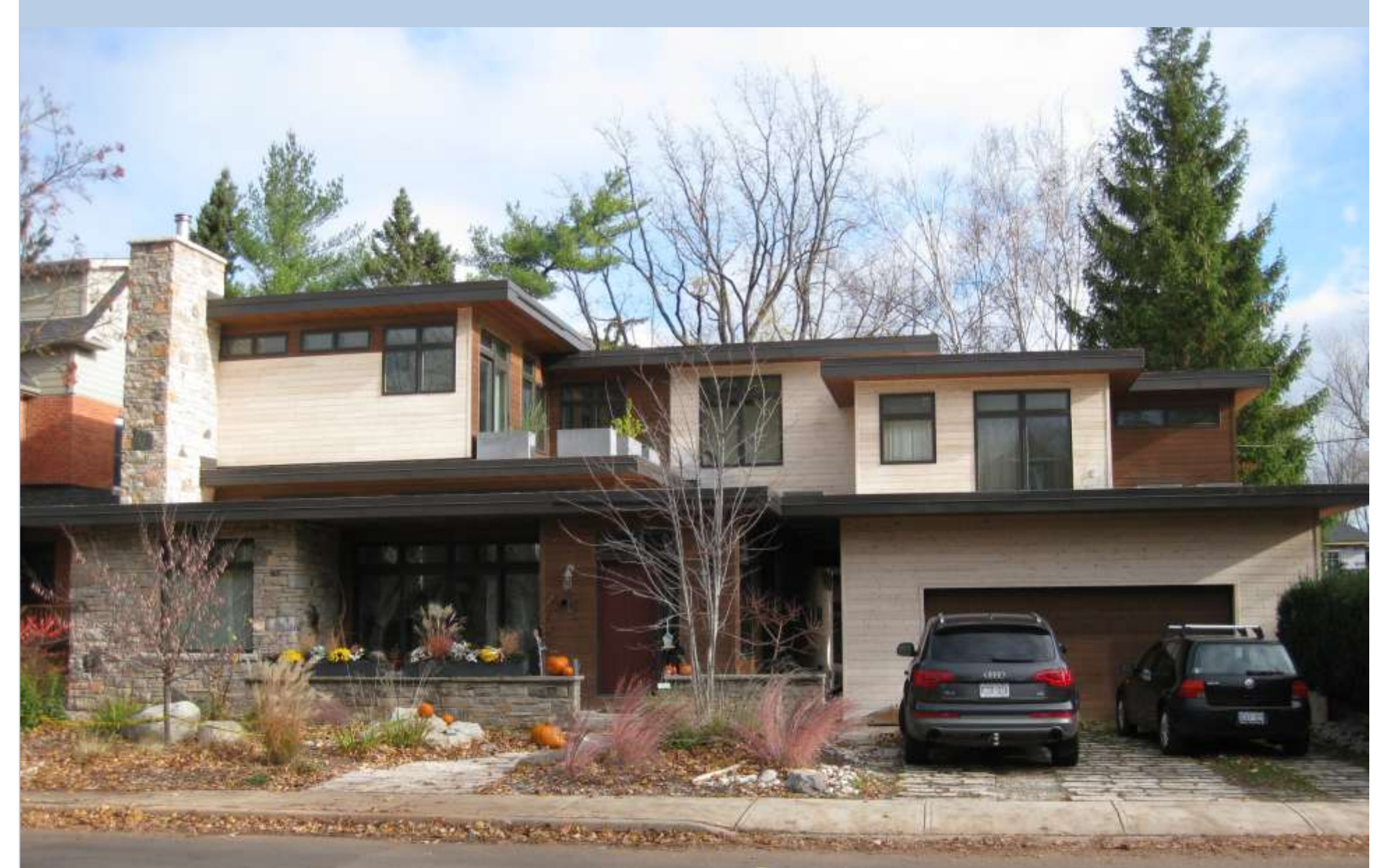
This house fits well into the neighbourhood as the massing is broken into smaller elements, including wall projections, a porch and balcony, and change in materials.
