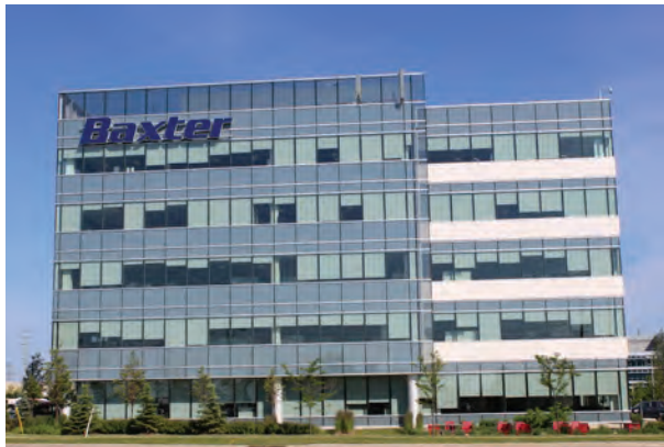
Roof top mechanical screening is incorporated into the overall building design
