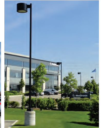
Light standards positioned to provide uniform light distribution and off-set from plantings (4.4.5)
