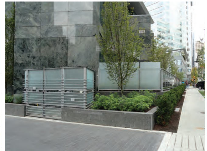
Well integrated and screened utility meters
