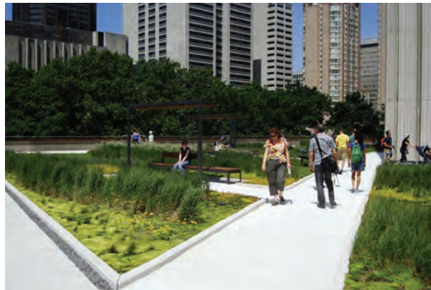
A green roof provides additional amenity space
