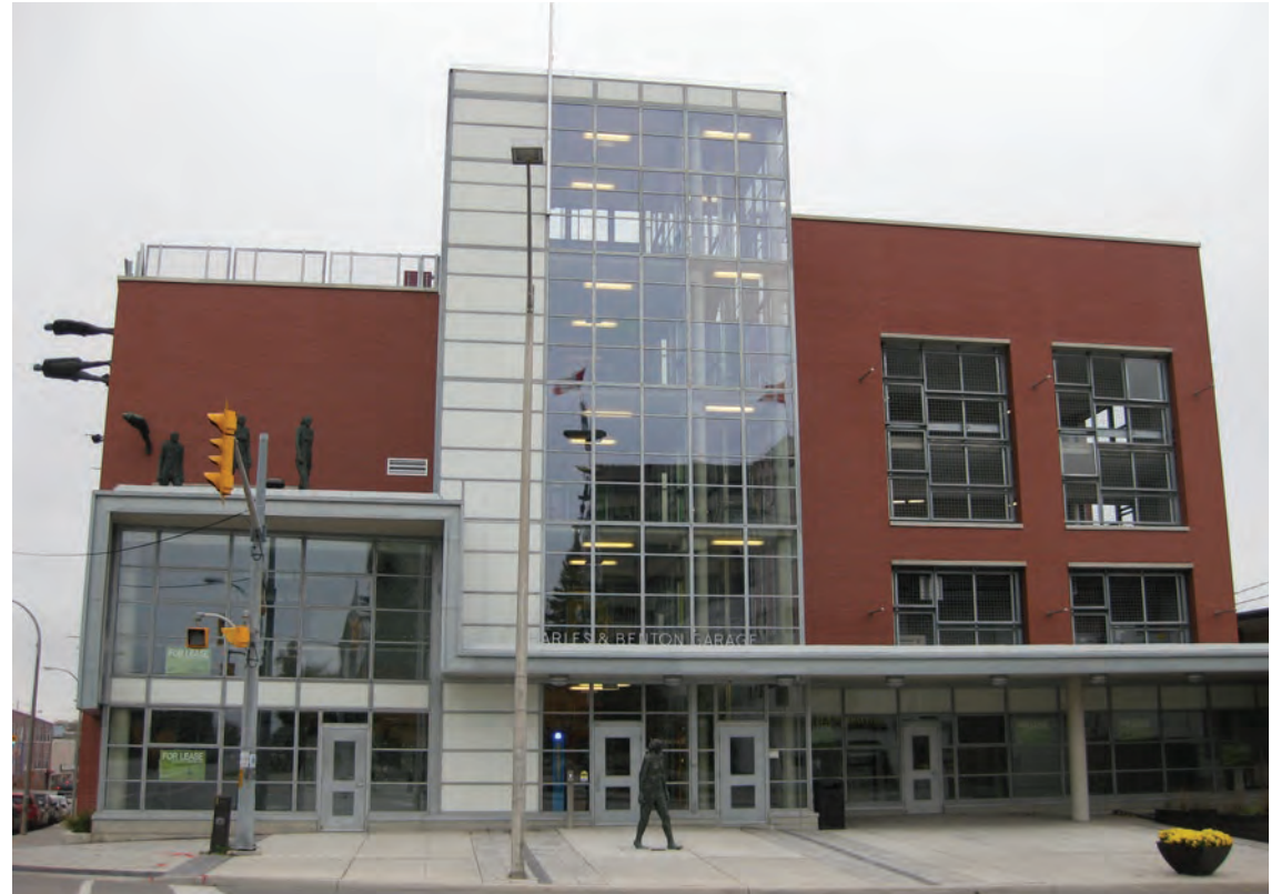
A well designed, visually interesting above-ground parking facility
