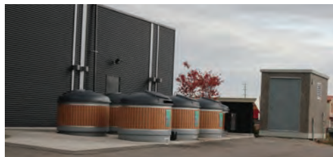
Facilities positioned in an orderly manner behind the building to screen from view (4.6.3)
