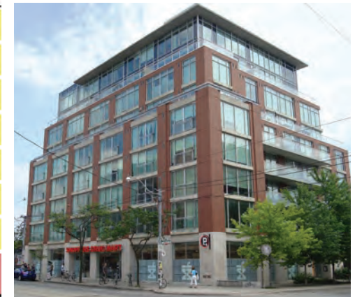
Building base frames the street with a stepback above 12m from grade
