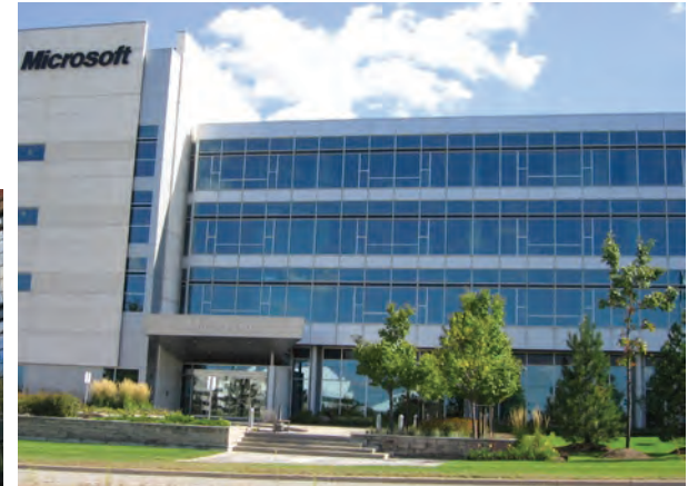
Principal building entrance accessed directly from the public realm
