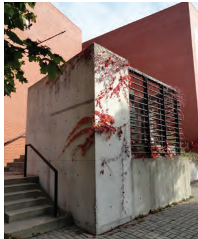
A wall, louvers and plantings screen the facilities (4.6.6)
