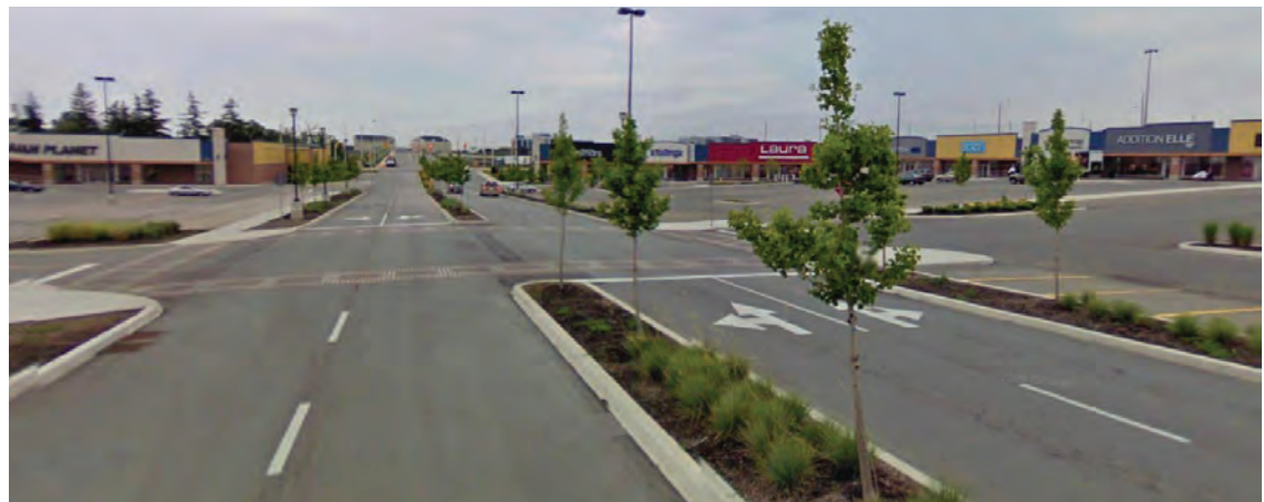
Consolidated access leading to the parking area aisles designed as an extension to the public street
