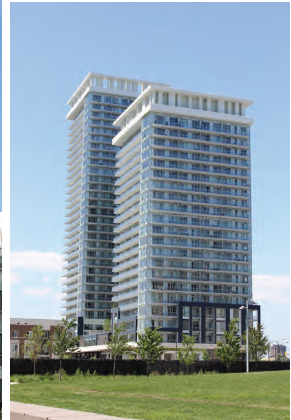
Mechanical penthouse is architecturally integrated into the building design
