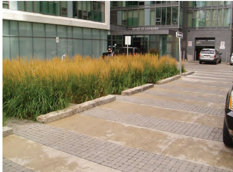
Stormwater management enhanced with permeable paving and sheet flow drainage to a bio-swale (4.1.13 to 4.1.15)
