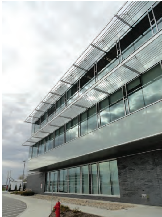
Louvers assist to regulate sun exposure
