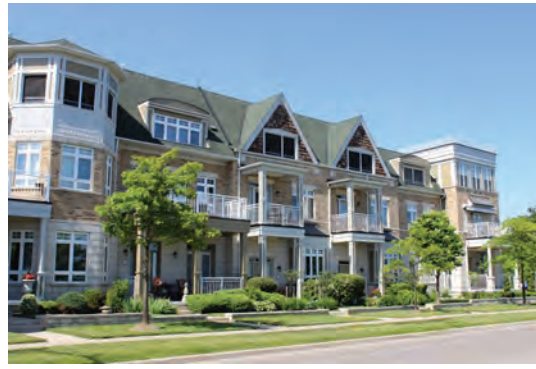
Built form positioned close to the street (without driveway interruptions) supports pedestrian environment
