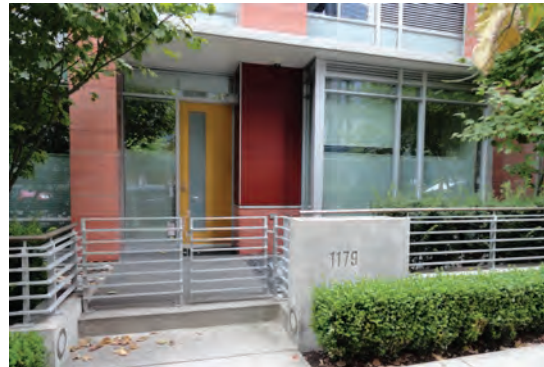
Weather-protected main entrance oriented towards the street
