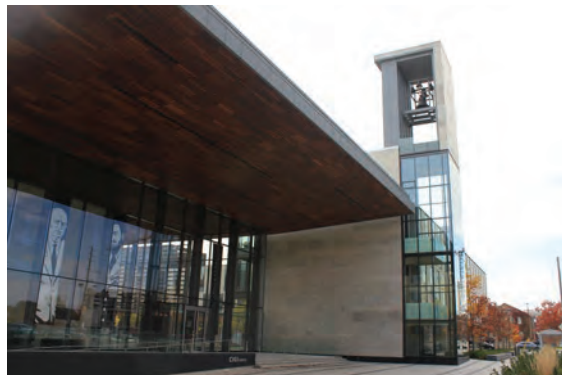
Vertical component breaks the long façade and accentuates the main entrance
