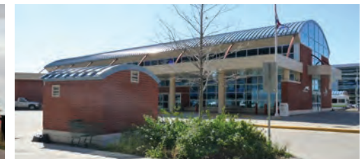
Separate storage building that complements the main building design (4.6.3)
