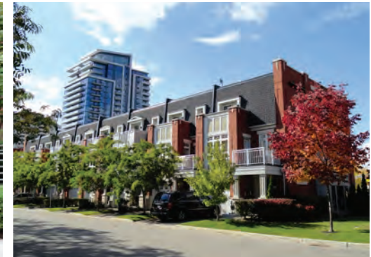
Garage entrances are flush with the main façade
