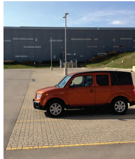
Parking lot incorporates permeable pavers
