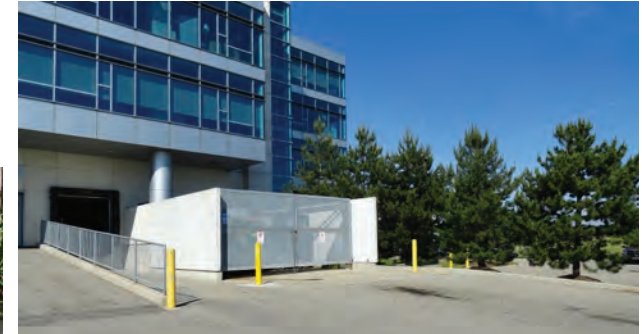
Service area screened with dense landscaping and walls (4.6.5)
