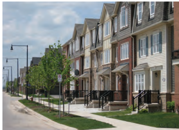
Varied roof lines create visual interest
