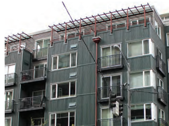
Articulated upper floors and unique roof design creates an attractive skyline
