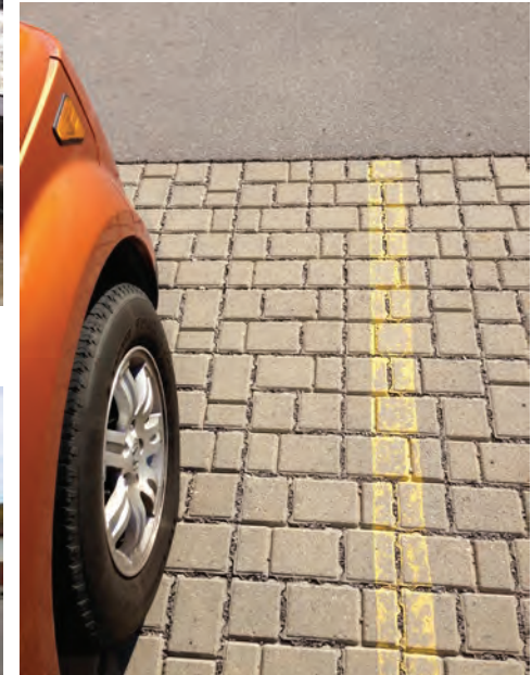
Permeable paving in a parking area (4.1.14)
