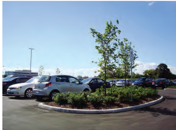
Major drive aisle unobstructed by parking spaces
