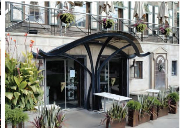
Entrance clearly identified with artistic canopy feature
