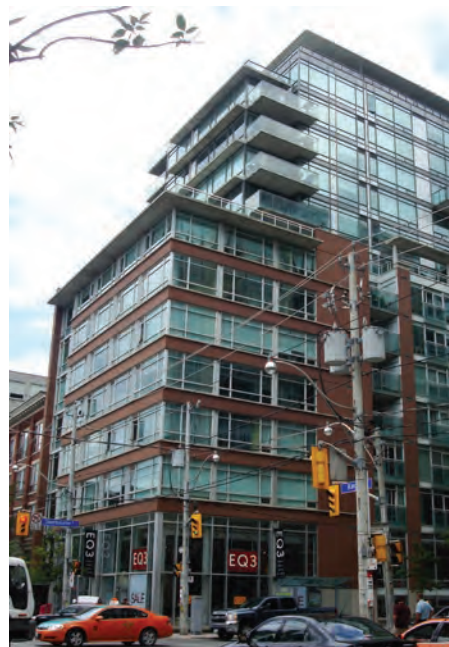
Building middle steps back from the main wall of the base
