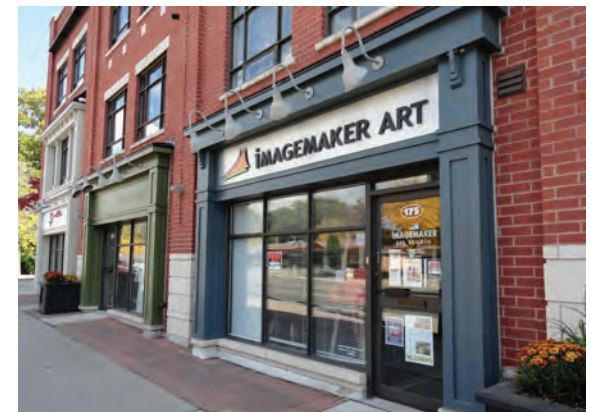
Transparent openings enhance the pedestrian experience along the street
