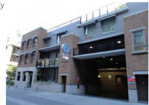
Underground parking incorporated into a residential building
