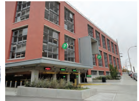
Vehicular entrance designed to complement the structure
