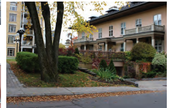
Successfully screened underground parking features exposed walls of the same material as the adjacent built form
