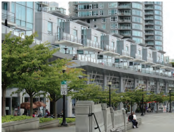
Balconies and terraces enhance of the façade and provide additional amenity spaces
