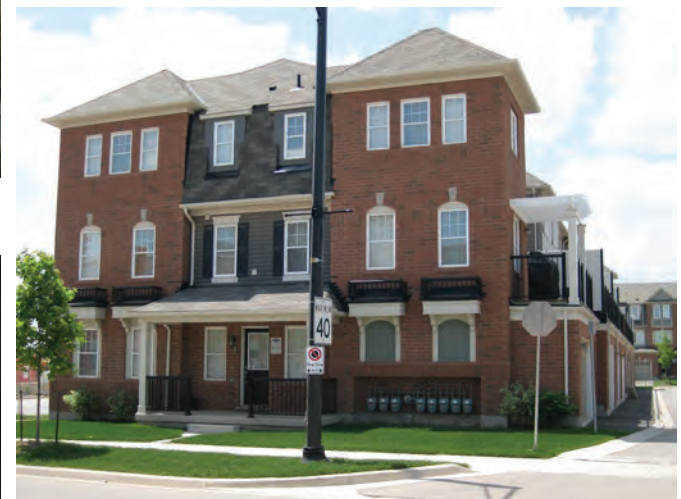
Meters located on the side of the building
