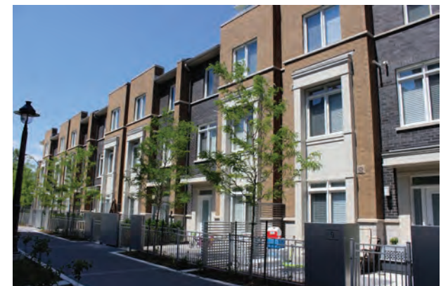
Projections and recesses divide the massing of a long façade
