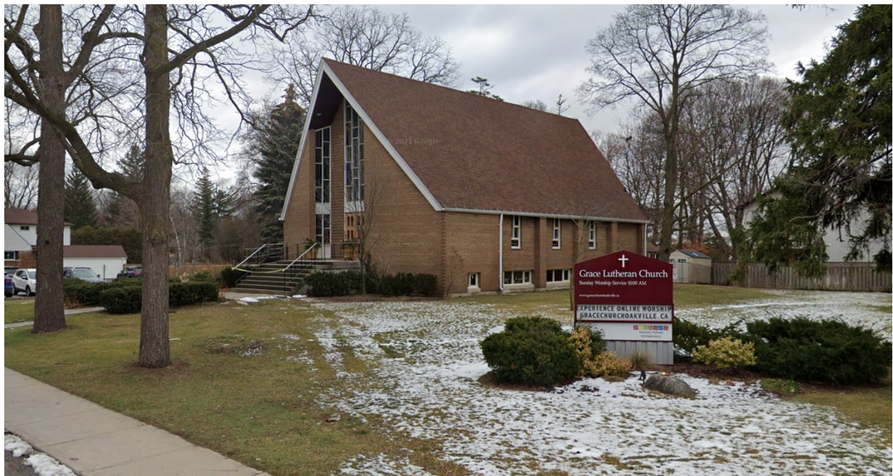
Photo 1: Subject Lands (Grace Lutheran Church of Oakville – 304 Spruce Street) looking south from Spruce Street
