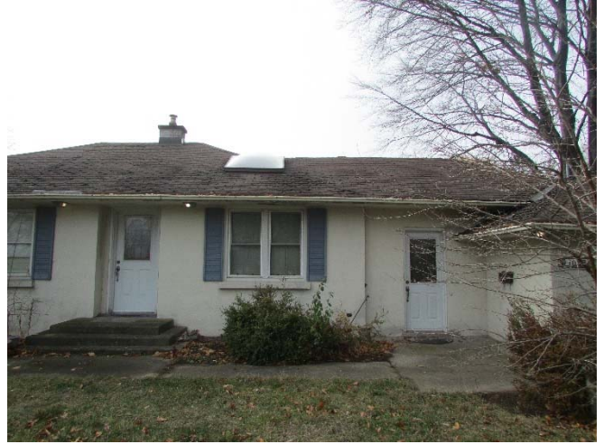
Photo 2: View of a portion of the east elevation of Building B, looking west.
