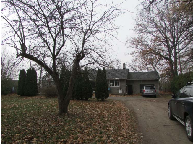
Photo 1: View of a portion of the east elevation of Building A, looking west.
