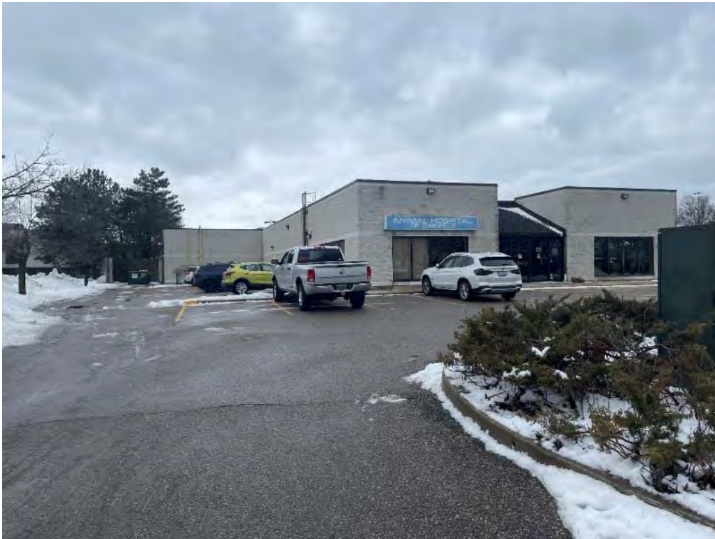
Photo 15: Property located east adjacent at 234 South Service Rd East.
