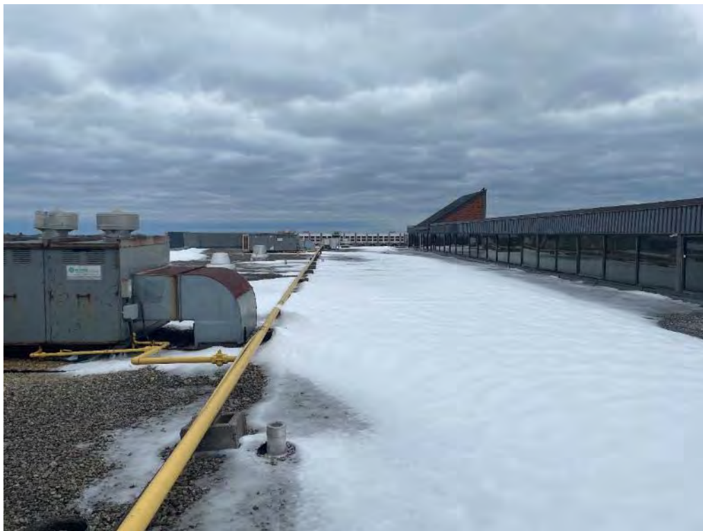
Photo 4: Roof of Site building, facing east.
