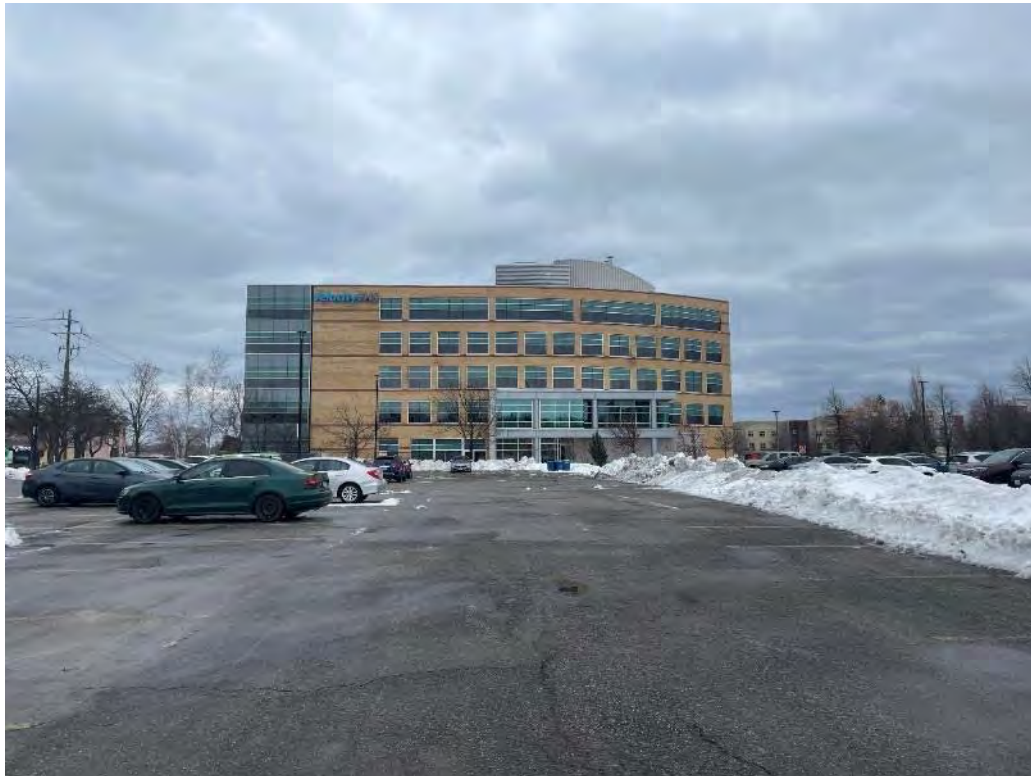
Photo 14: Parking lot in the western portion of the Site, facing south.
