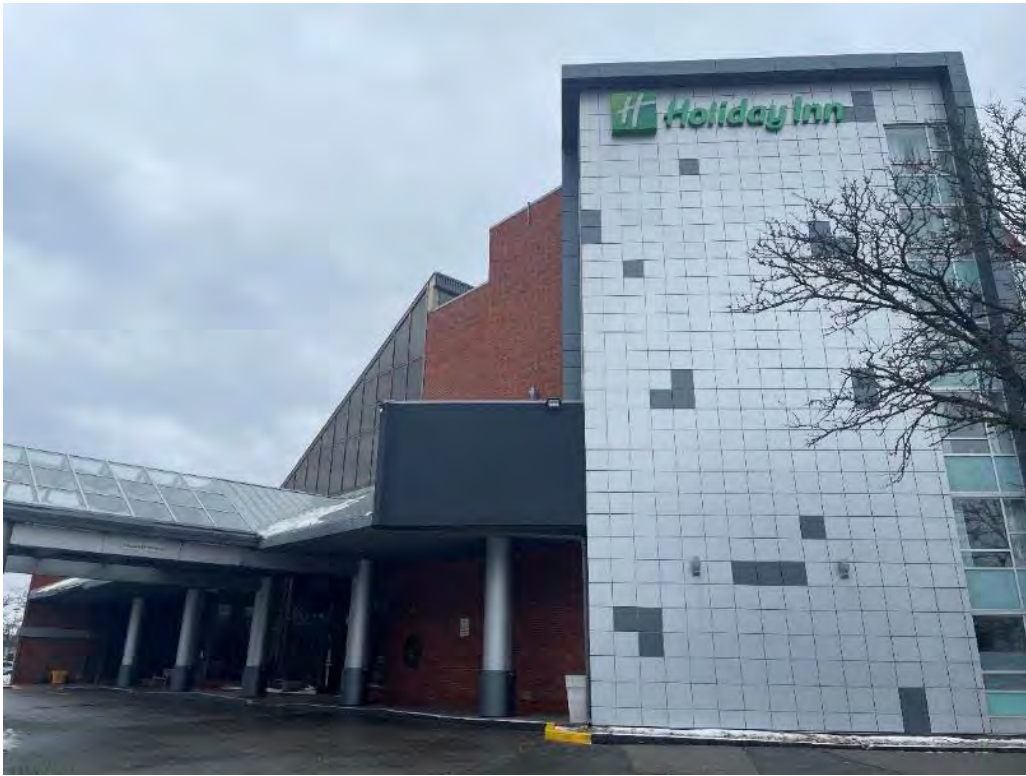
Photo 1: Frontage of Site building facing northwest.
