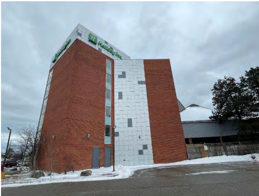
Photo 2: Rear of the Site Building facing south.
