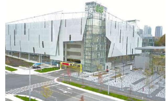
Parking structure at Cooksville GO Station with LEED features (Source: Infrastructure Ontario)
