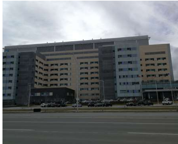
Main Hospital entrance, looking west along Third Line
