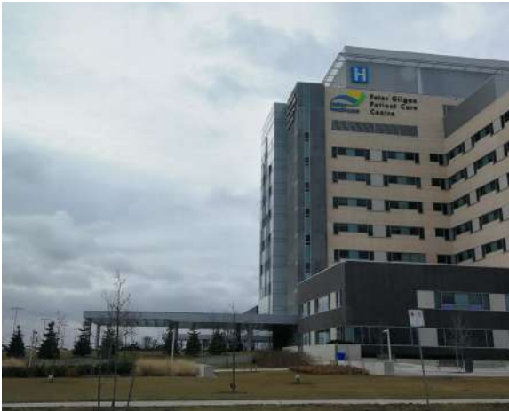
Hospital, looking west along Third Line
