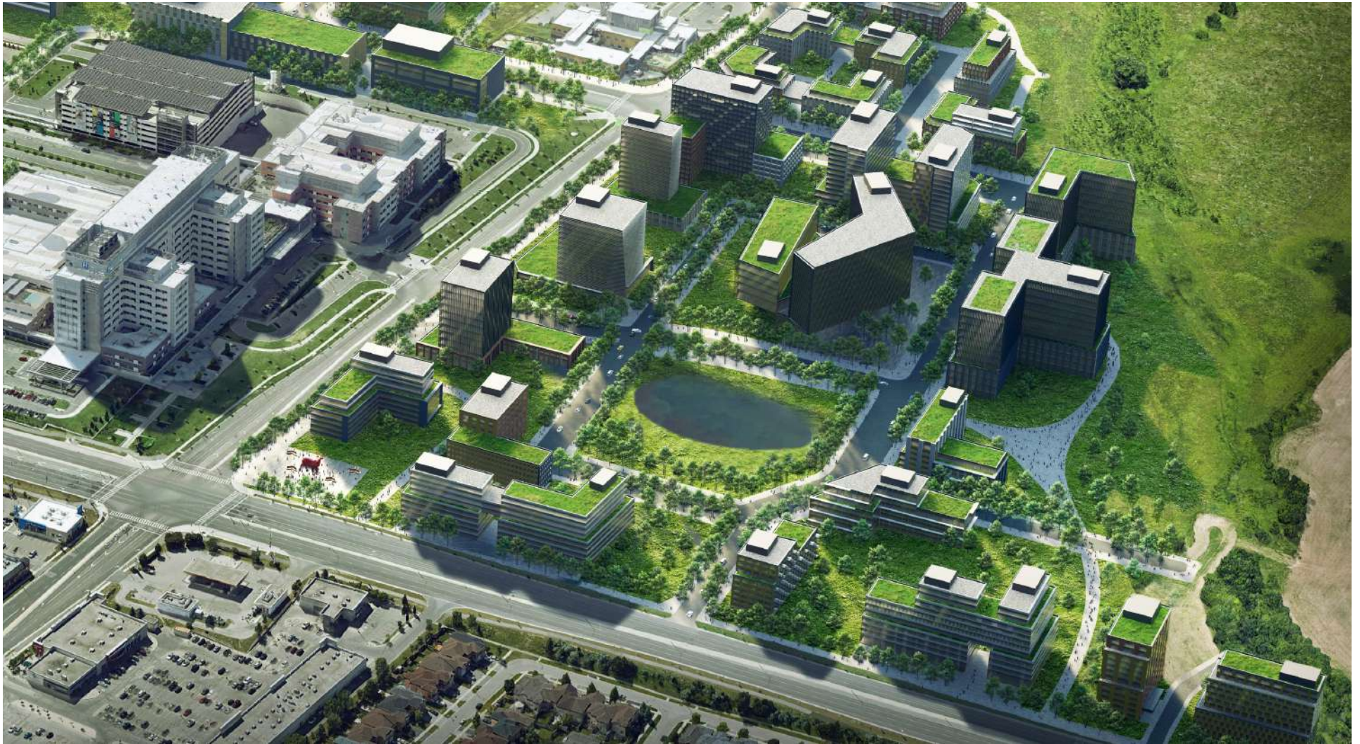
Figure 22 | Hospital District - East
