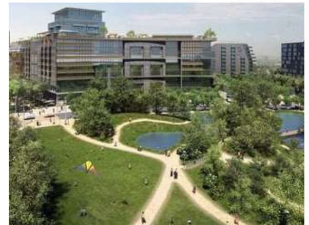
Building scale creates softened relationship with natural areas (Source: Waterfront Toronto)
