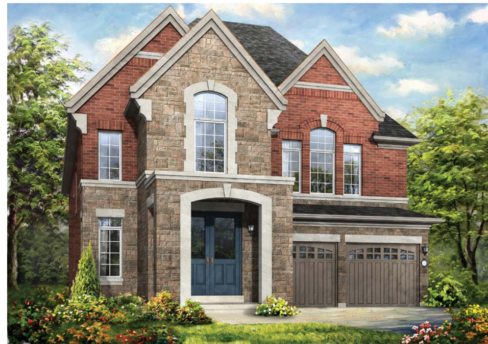
Figure 7.6: Examples of dwellings with brick as primary building material, with stone foundation and asphalt roof shingles.
