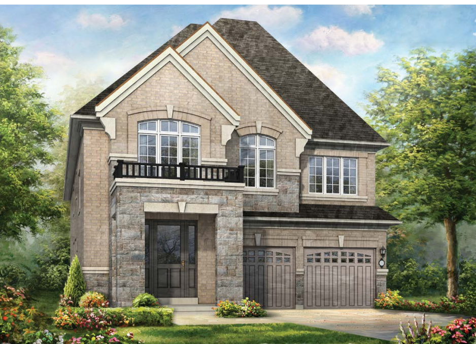
Figure 7.5: Examples of dwellings with brick as primary building material, with stone foundation and asphalt roof shingles.
