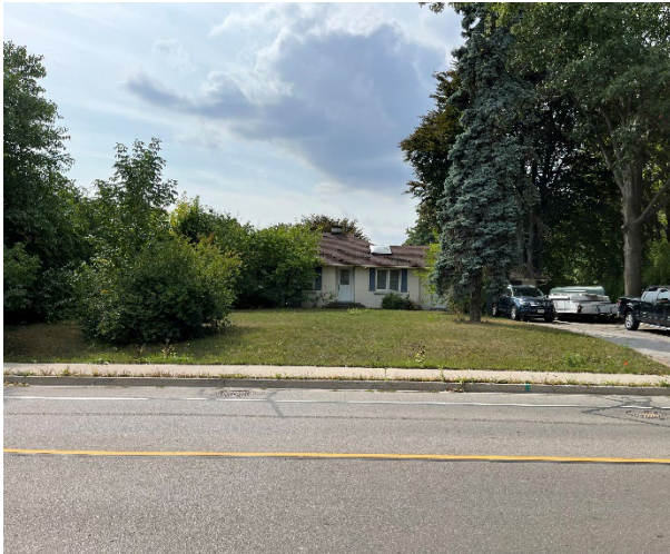
View looking west along Sixth Line toward 1020 Sixth Line
