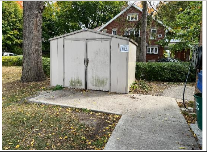
14. Wooden storage shed, located near the south-central portion of the Site.
