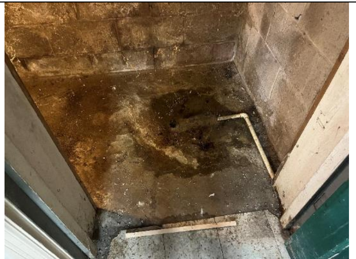
12. View of a floor drain, in a closet, in the basement of 318 Spruce Street
