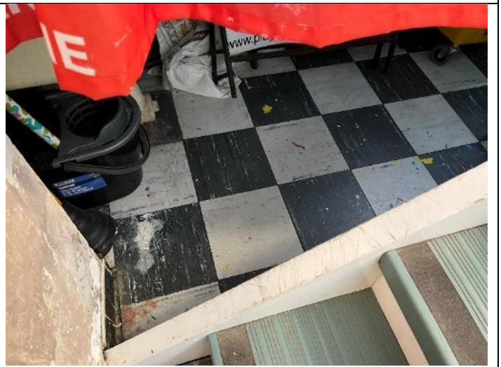
4. Original vinyl floor tile observed in the basement at 304 Spruce Street
