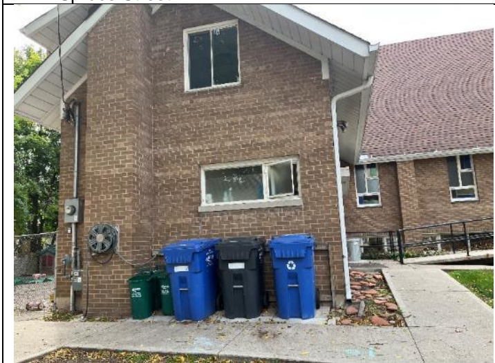
15. Non-hazardous waste bins, located on the east exterior wall of 304 Spruce Street.
