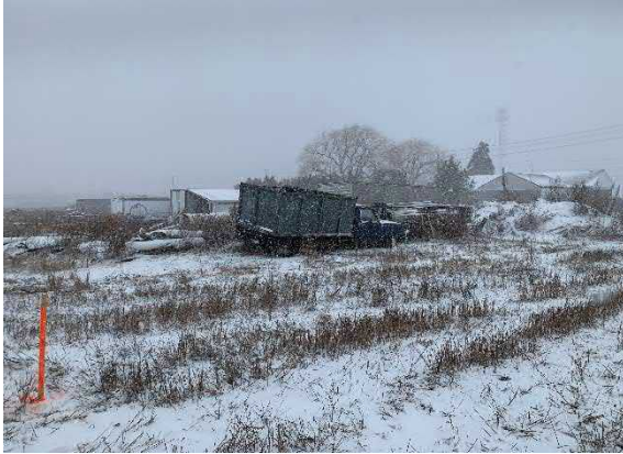
Picture 7: View of east adjacent property (3278 Regional Rd. 25) and several trucks, piping and stock piles on the Phase One Property, facing east.
