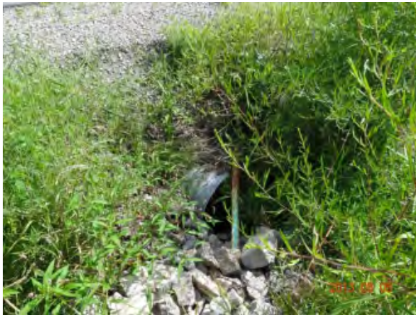
Figure 9: u/s side of Culvert ME-B1
