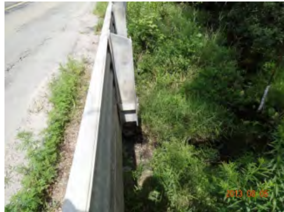
Figure 4: d/s end of Bridge JC-B4
