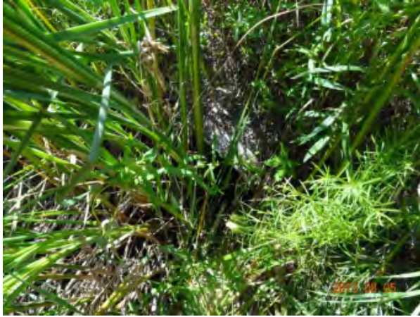
Figure 7: d/s side of Culvert JC-B9
