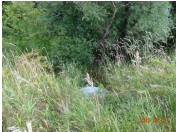
Figure 12: d/s side of Culvert ESM-B14
