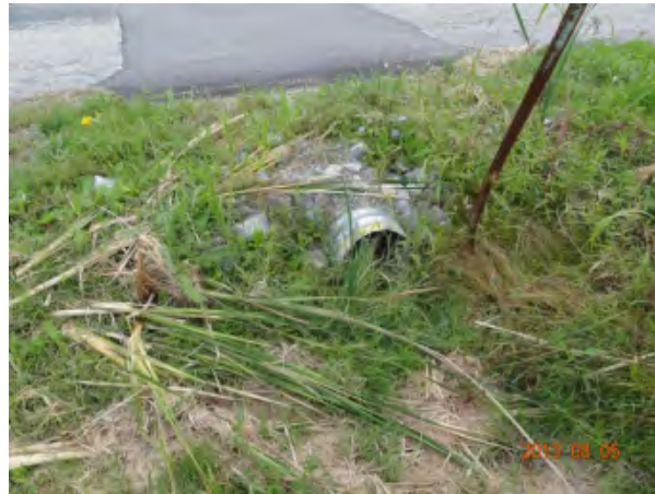
Figure 10: d/s side of Culvert ME-B1
