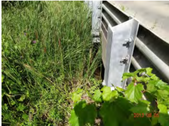
Figure 3: u/s end of Bridge JC-B4
