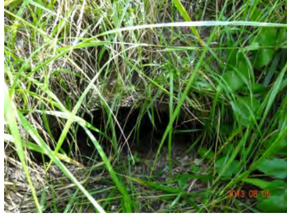
Figure 2: d/s end of Culvert JC-B2
