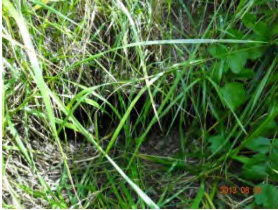
Figure 1: u/s end of Culvert JC-B2
