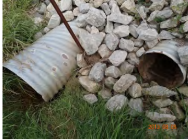
Figure 8: u/s side of Culvert JC-B10
