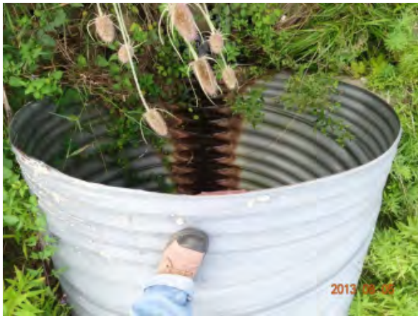
Figure 11: u/s side of Culvert ESM-B14
