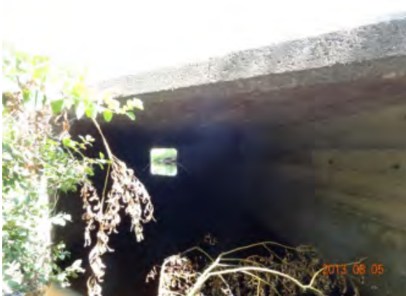
Figure 5: u/s end of Culvert JC-B7
