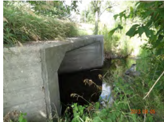
Figure 6: d/s end of Culvert JC
