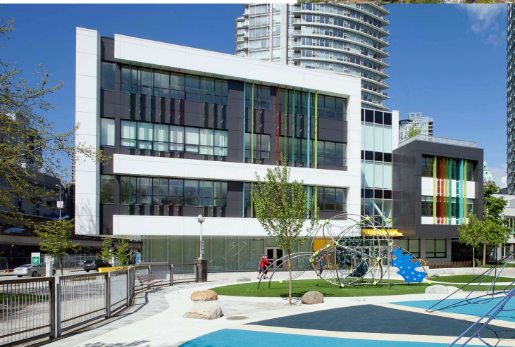
Crosstown Elementary School, Vancouver Source: Robert Stefanowicz
