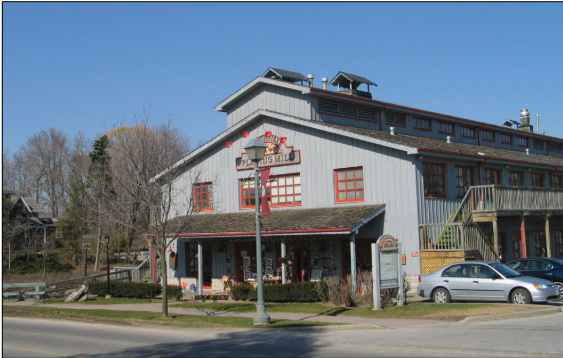
Compatible Infill Development Models inspired by former Unionville Planing Mill. Source: Town of Markham
