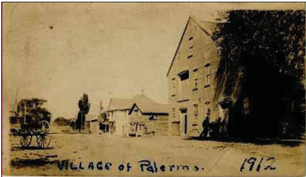
Former Palermo Agricultural Works. Source: Trafalgar Township Historical Society
