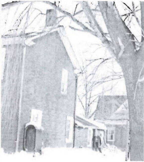
West wall of house and addition, 1962.
