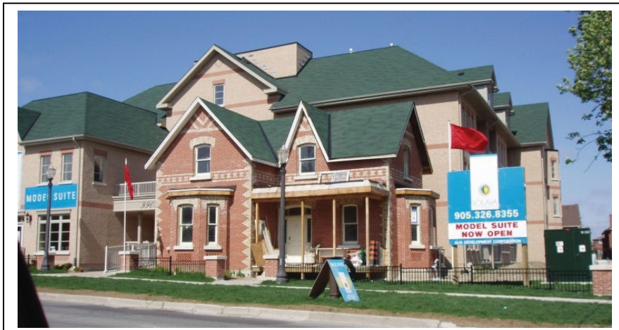
Village house preserved in a medium density development Maple Village, City of Vaughan Source: Town of Markham Planning Services Department
