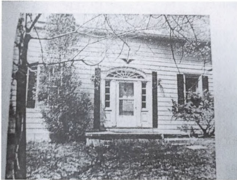
Original doorway – removed in 1992.
