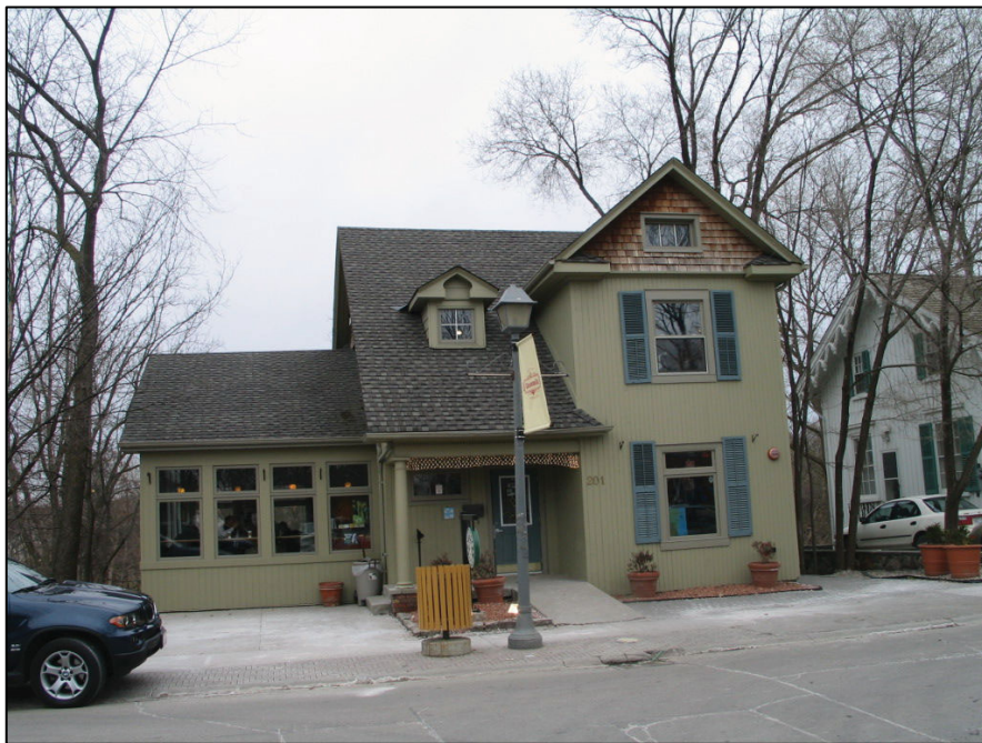
Former residential building converted to a coffee shop – Main Street Unionville. Source: Town of Markham
