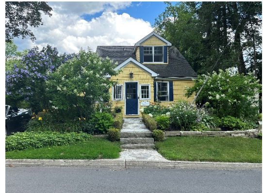
Figure 28: Flagstone pathway used at 230 King St.
