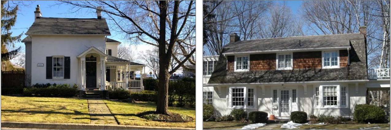
Figure 4: Black asphalt shingles, 212 King St. (left); Cedar shake roof 309 King St. (right).
