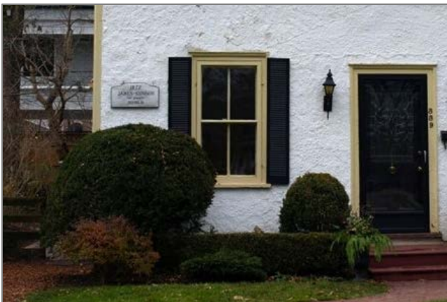
Figure 6: Two-over-two windows 339 William St. (left); Six-over-six windows 212 King St. (right).
