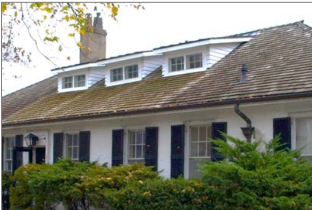
Figure 5: Shed dormers 212 Front St. (left); Wall-style gabled dormers 295 King St. (right).
