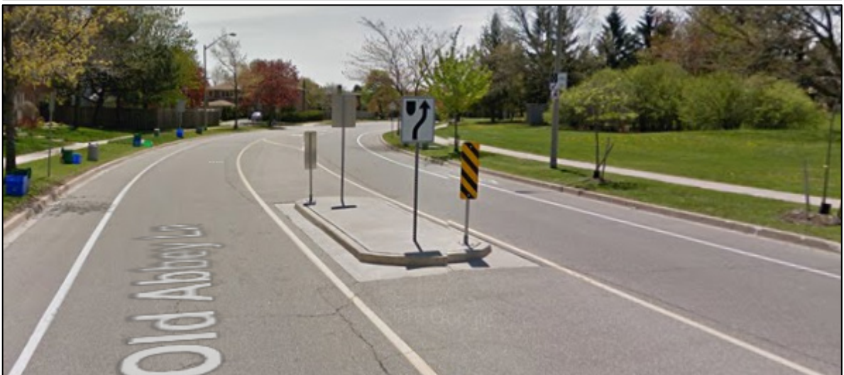
Raised centre median installed as traffic calming measure on Old Abbey Lane
