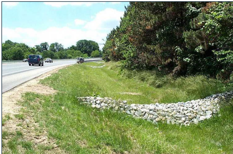
Figure 7-11: Enhanced Grass Swale (Low Impact Development Stormwater Management Planning and Design Guide, Version 1.0, CVC and TRCA, 2010)
