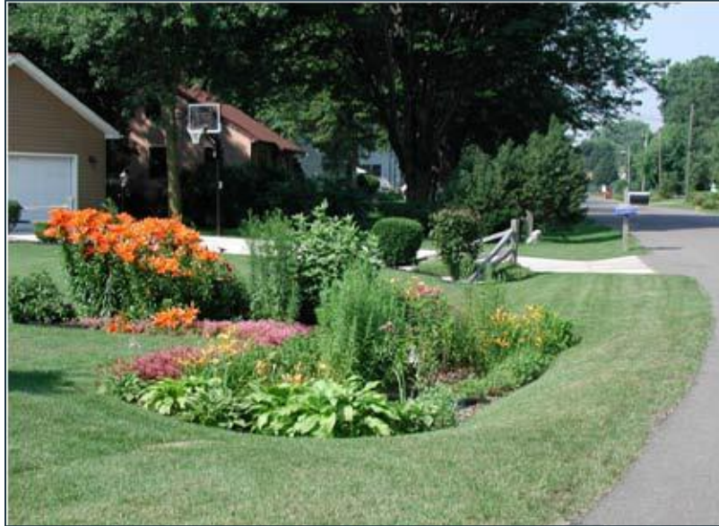
Figure 7-12: Bioretention Facility (Low Impact Development Stormwater Management Planning and Design Guide, Version 1.0, CVC and TRCA, 2010)
