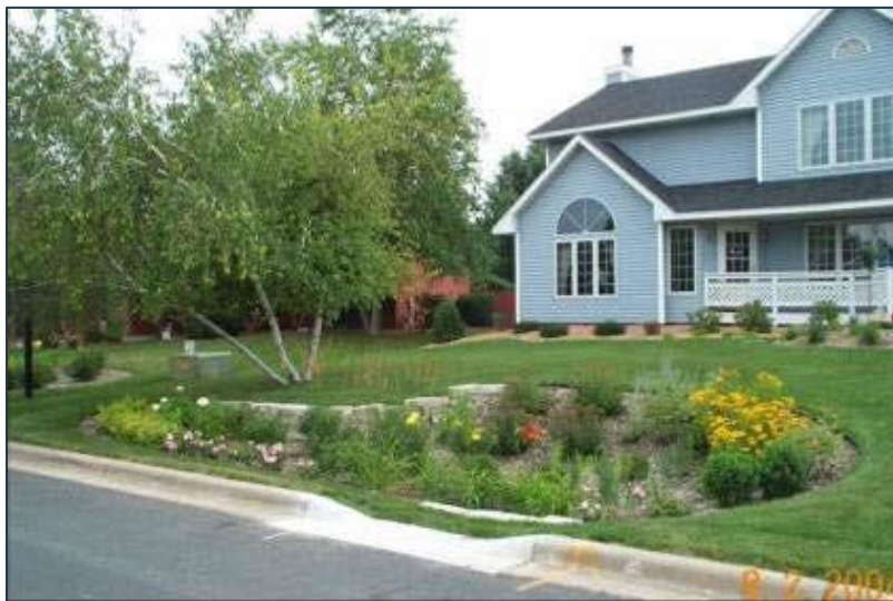
Figure 7-13: Bioretention Facility (Low Impact Development Stormwater Management Planning and Design Guide, Version 1.0, CVC and TRCA, 2010)
