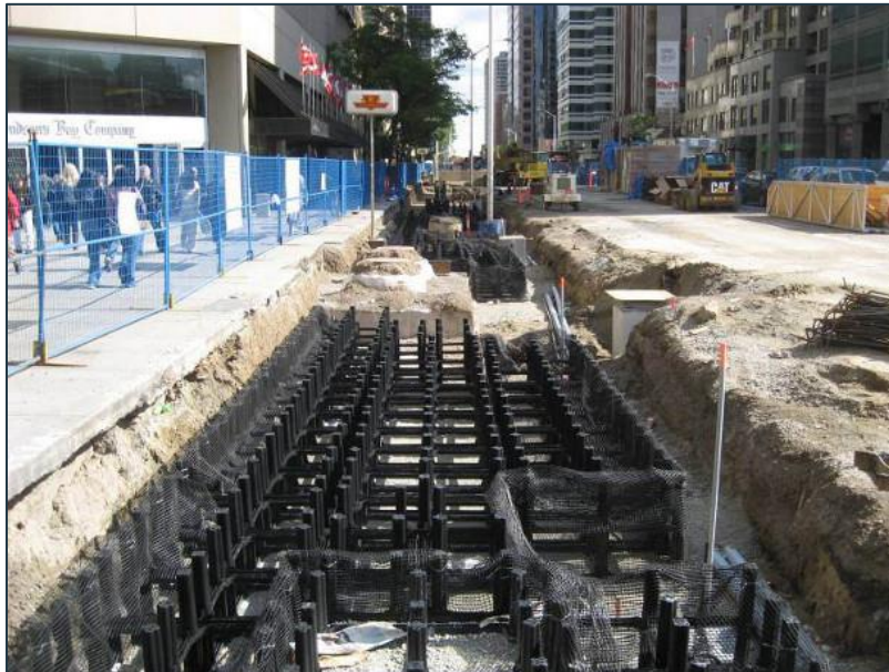
Figure 7-15: Silva Cell Construction (www.smartcitiesdive.com, 2020)
