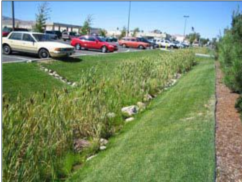
Figure 7-10: Enhanced Grass Swale (Low Impact Development Stormwater Management Planning and Design Guide, Version 1.0, CVC and TRCA, 2010)
