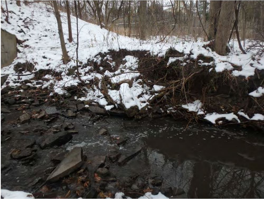
Photo 5: Erosion evident at east bank immediately downstream of Rebecca Street retaining wall. Area spans approximately 10.3 m in length. Height of erosion averages at 1 meter.
