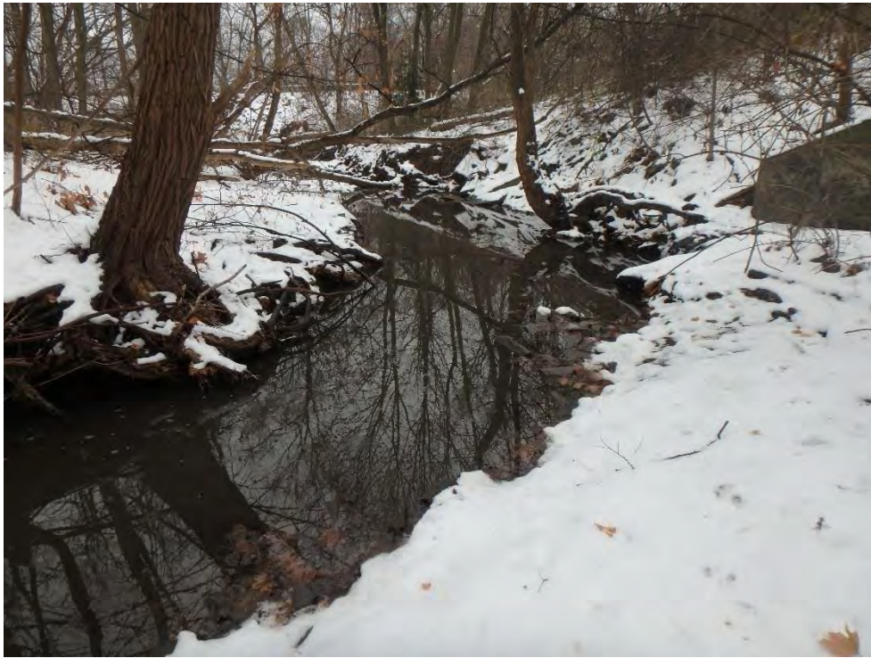
Photo 7: Downstream banks stabilize before erosion area present on west bank.
