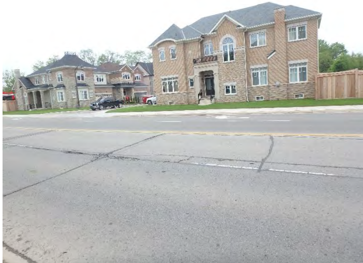
Photo 1: Crossing C1 - north of ROW.
