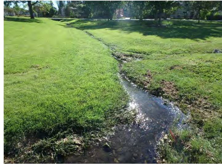
Photo 18: Downstream end of crossing C5 facing downstream culvert.
