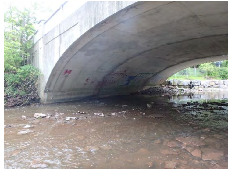
Photo 34: C11 east side of bridge.
