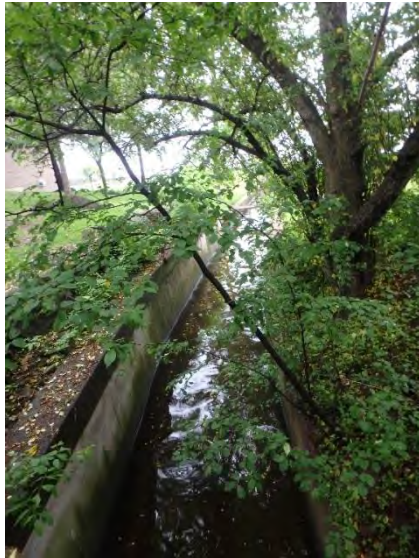
Photo 25: Crossing C8 downstream of ROW.
