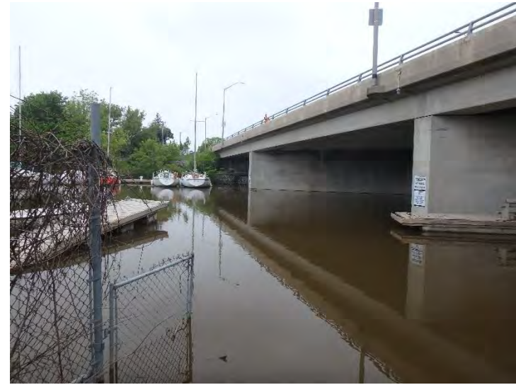
Photo 10: C2 under bridge ROW facing south.
