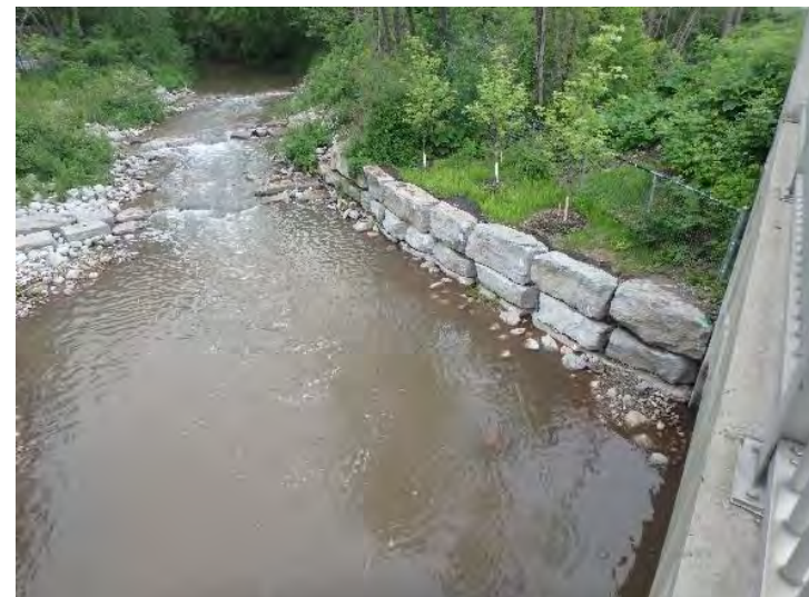
Photo 32: Crossing C11 northeast bank.
