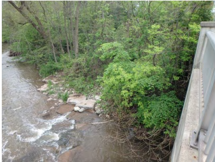
Photo 37: C11 southwest bank of bridge.
