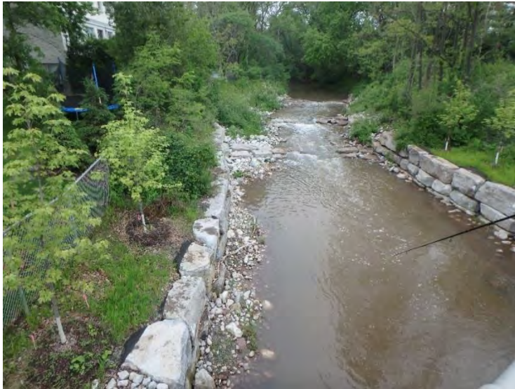
Photo 33: Crossing C11 northwest bank.
