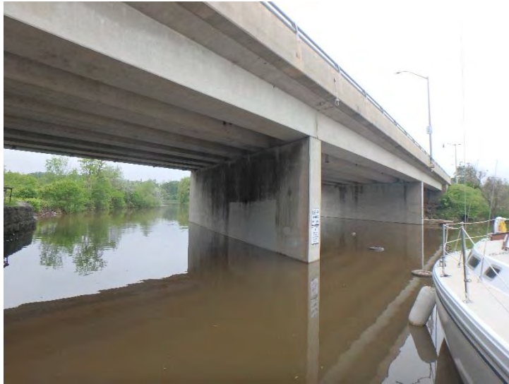
Photo 9: C2 under bridge ROW facing north.
