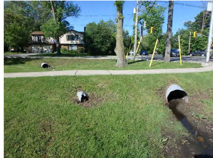
Photo 14: C4 southwest of intersection.
