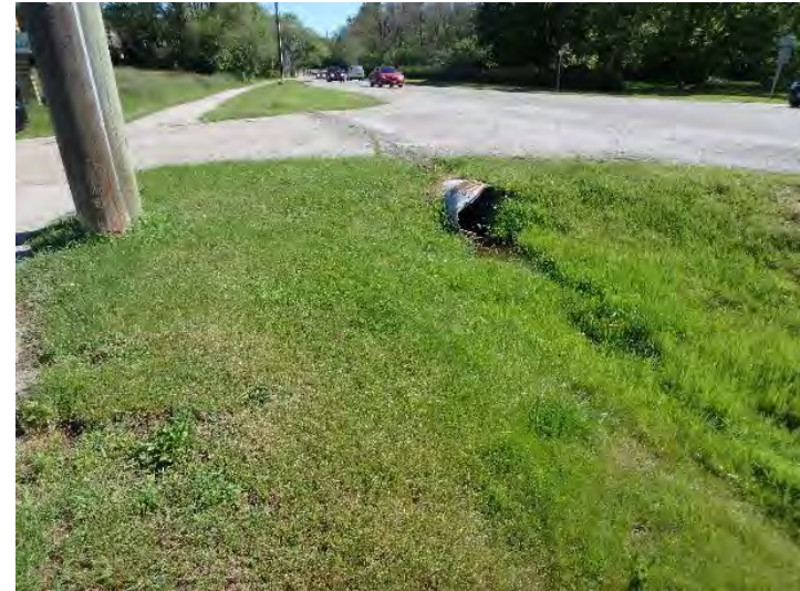
Photo 30: Crossing C10 west side.
