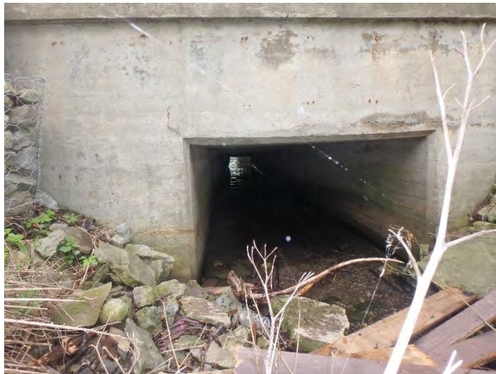
Photo 27: Bridge at C8.
