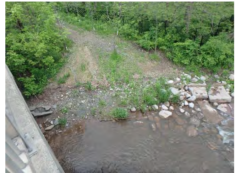
Photo 36: C11 southeast bank of bridge.
