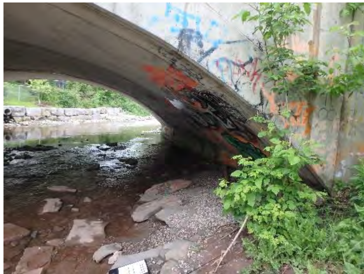
Photo 35: C11 west side of bridge.
