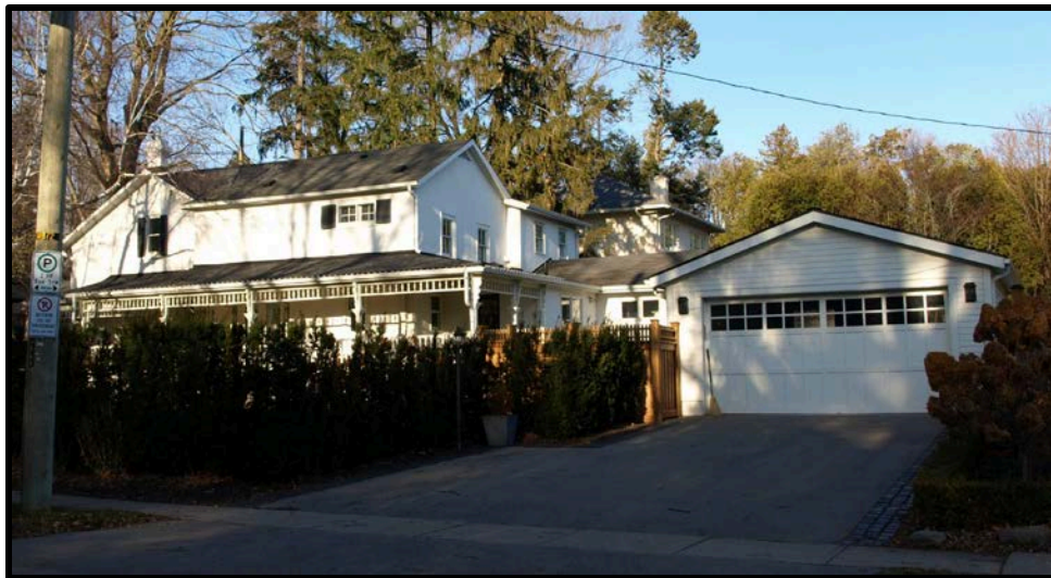
Figure 12: 212 King Street, 2017 porch addition and new garage, December 2021
