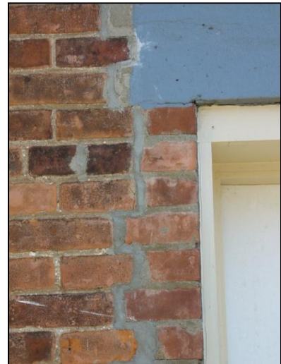
Repointing should avoid the use of Portland cement (as shown above) in favour of a lime-based mortar mix.
