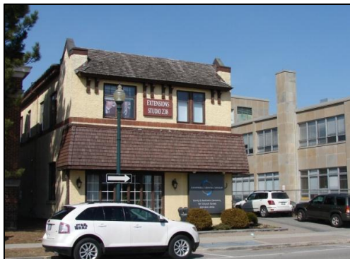
Fire Hall c. 1922.
