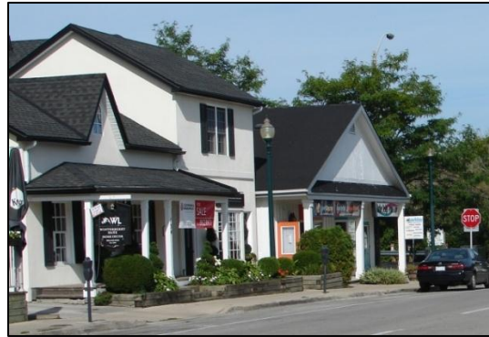
The height and scale of the new addition is larger than the original house (on left). As a result, the addition is not subordinate to the c 1845 Gothic Revival dwelling.
