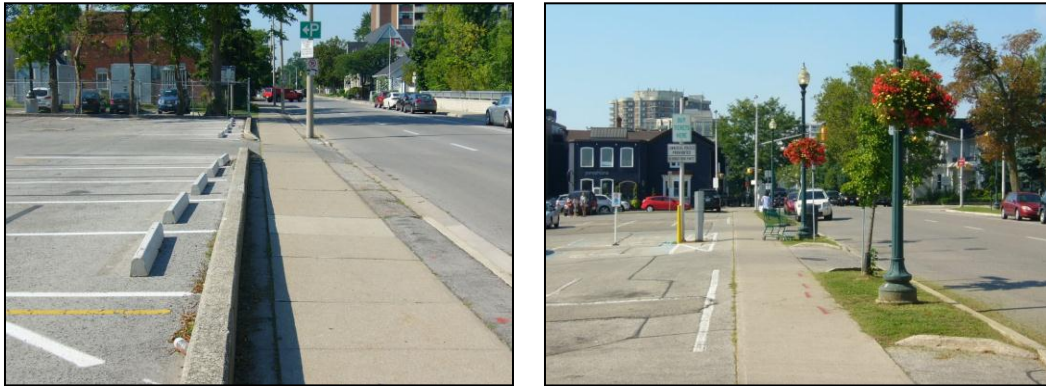
Poorly defined lot edges along the public sidewalk, as shown above, can be enhanced by adding masonry walls, street trees and hedging material.
