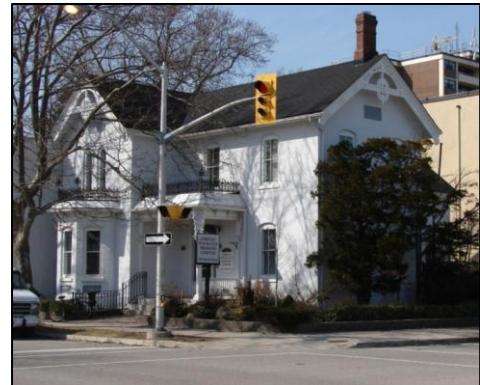
Original windows, entrances and walkways should be retained when establishing commercial uses in former residential buildings, as shown above.
