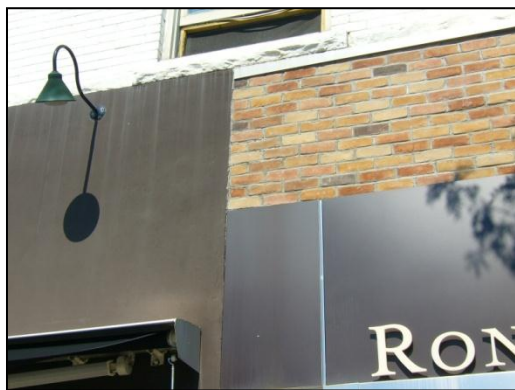
Fascia signs should be placed in their traditional locations on storefronts, and expansive areas of fascia boards (as shown here), not in scale with the storefront shall be avoided.
