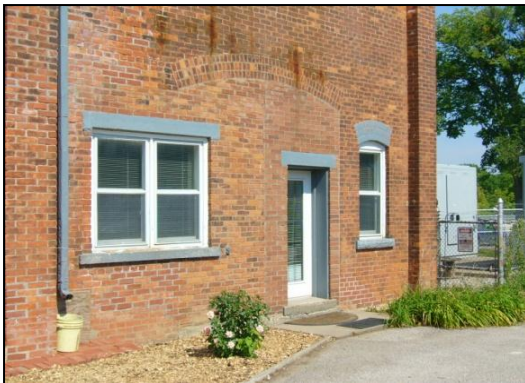
Maintain original openings, and avoid the introduction of new windows and entranceways, as was done here.
