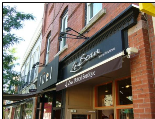
New signage should not obscure architectural detailing. This sign is a good example of sign placement that does not cover historic details.
