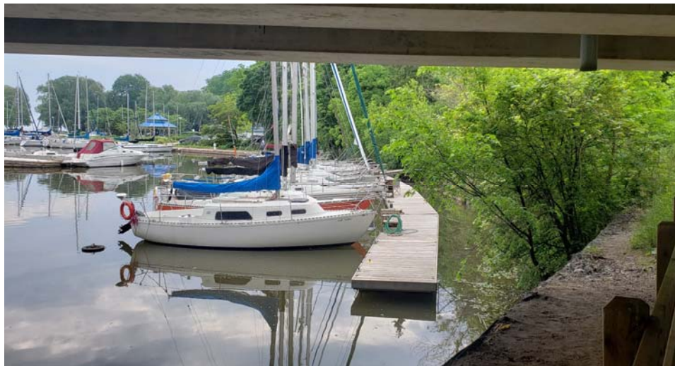
View looking south at Lakeshore Rd. W Bridge
