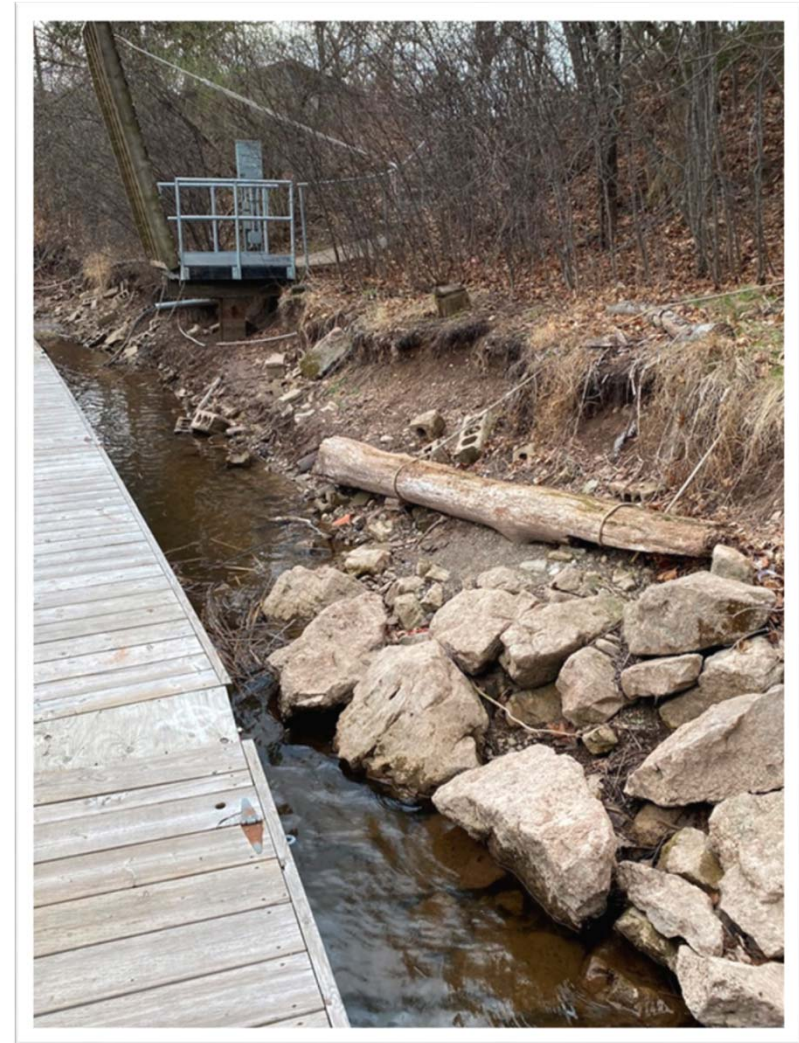
View looking south along the bank.
