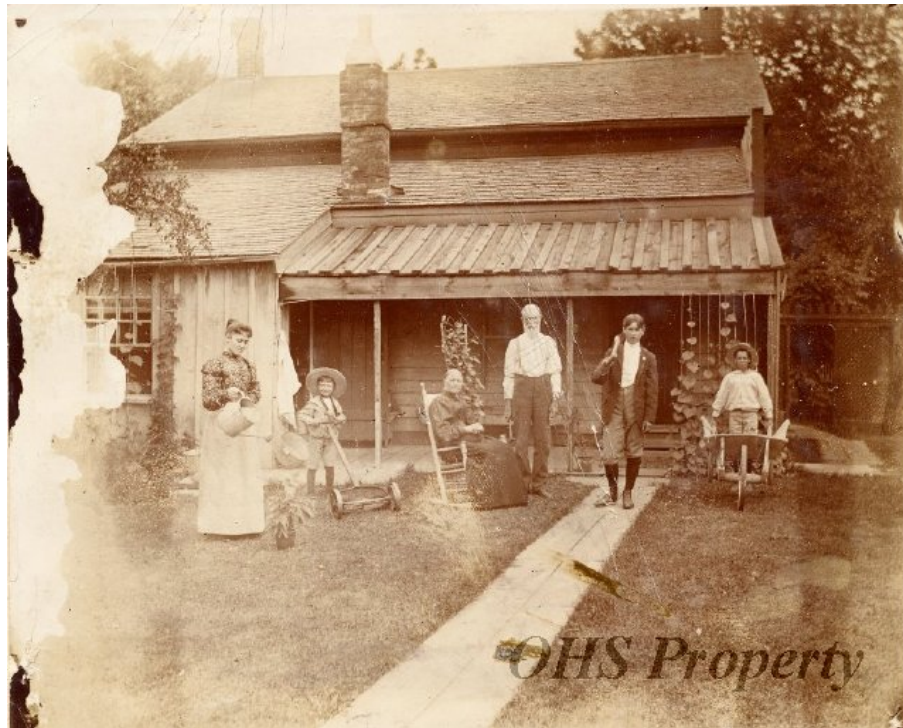
Rear of house
