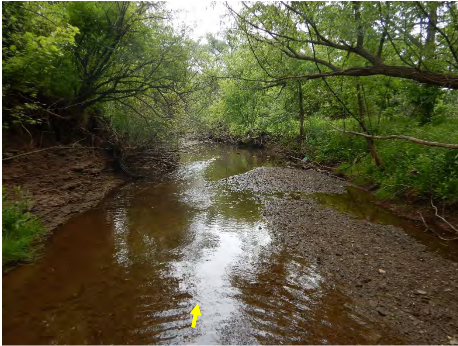
Channel conditions downstream of the South Service Road crossing were consistent with observations upstream, including valley wall contacts. In this instance, the channel laterally eroded Queenston Shale along the north side of the channel.
