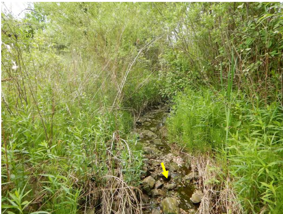
A small channel conveyed flows from a headwall located east of Third Line and discharged into Fourteen Mile Creek approximately 30 m from the South Service Road crossing. The channel was lined with cobbles and had significant algal growth.
