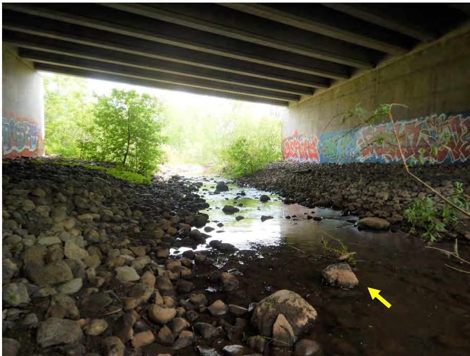
The Third Line crossing was a bridge, with the channel and banks composed of large cobble-sized riverstone.
