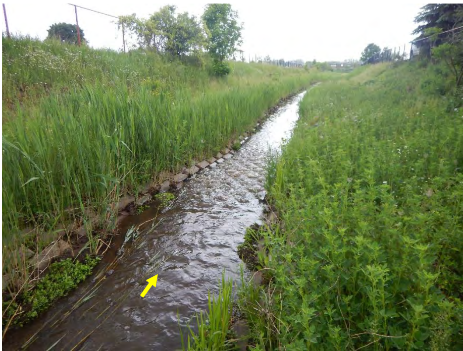
Taplow Creek downstream of South Service Road had a riparian buffer that lacked woody vegetation. The channel bed and banks were composed of articulated concrete blocks, consistent with upstream conditions.
