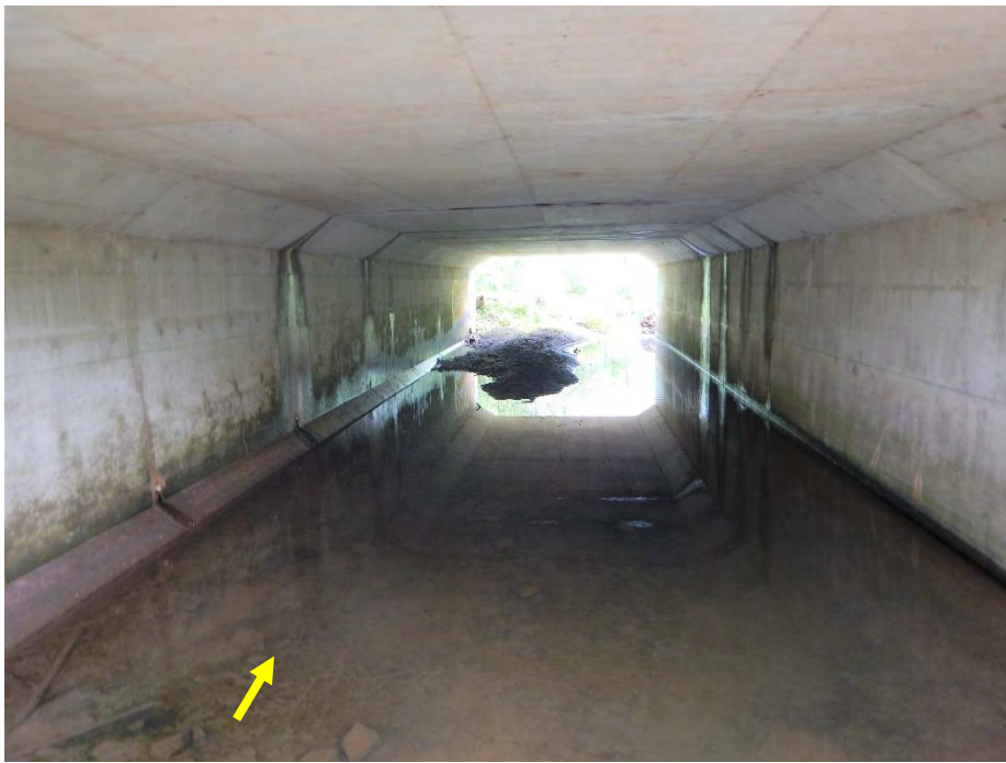
The northern culvert contained standing water.
