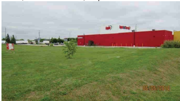
Plate 11: East view from Wycroft Rd.; Area is disturbed, no potential
