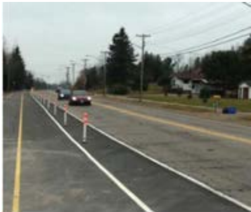
OPTION 4 – SEPARATED TWO-WAY CYCLE TRACK (ONE SIDE)
