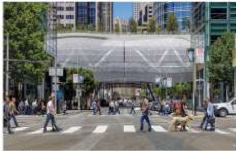
Salesforce Transit Centre and Park, San Francisco Source: Salesforce Transit Centre
