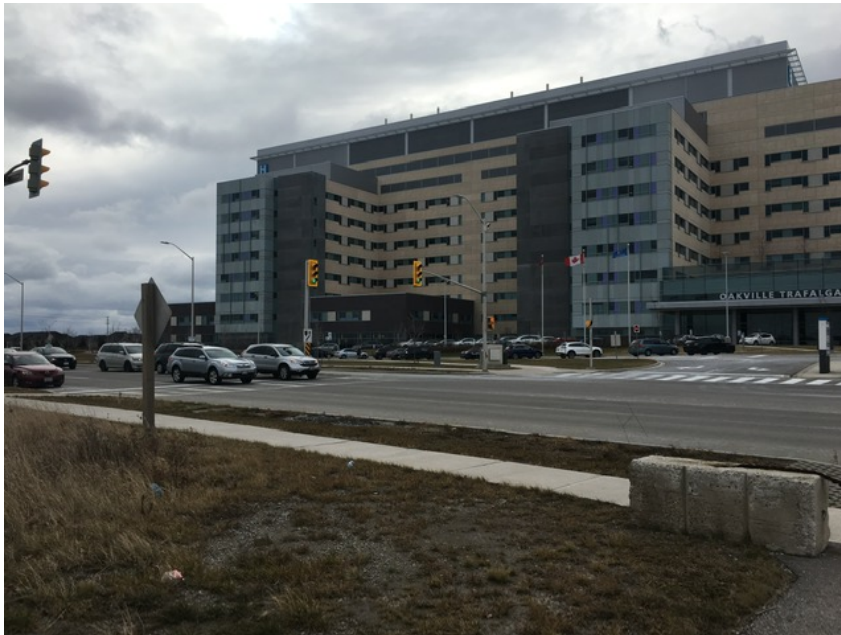
Oakville Trafalgar Memorial Hospital from Third Line Road, view facing west
