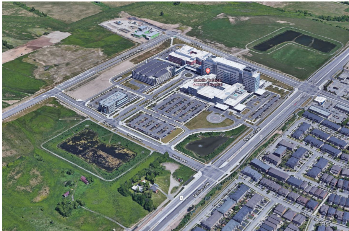
Figure 2 – Aerial of Study Area
