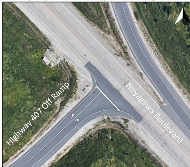
Figure 9: Highway 407 Eastbound Off Ramp at Neyagawa Boulevard
