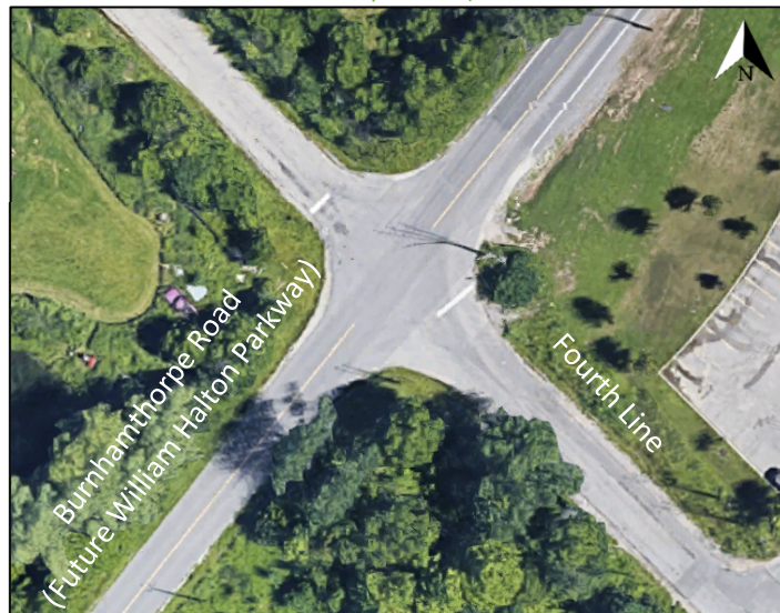
Figure 4: Fourth Line at Burnhamthorpe Road (Future William Halton Parkway)
