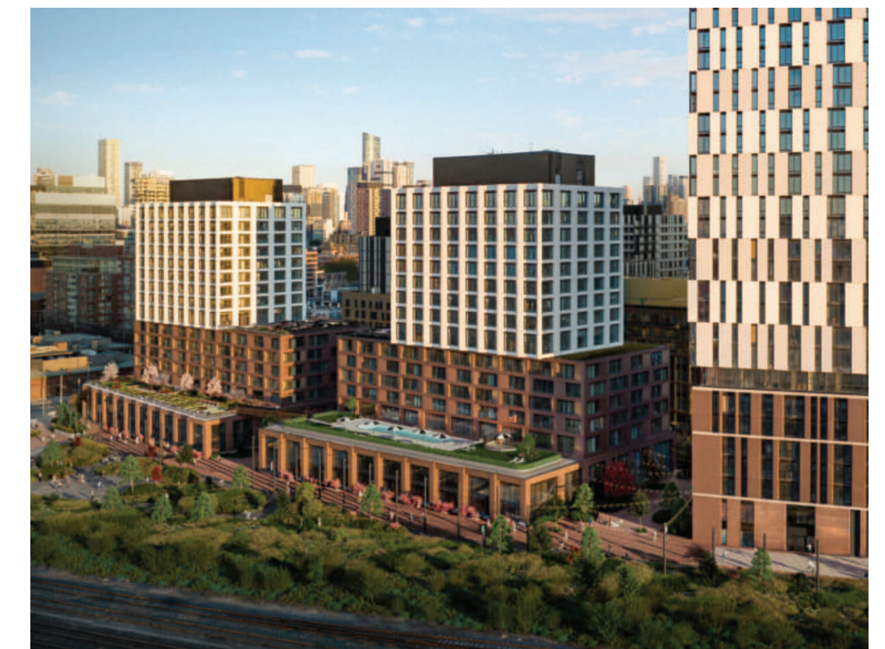
Maple House, Canary Landing, Toronto, ON
