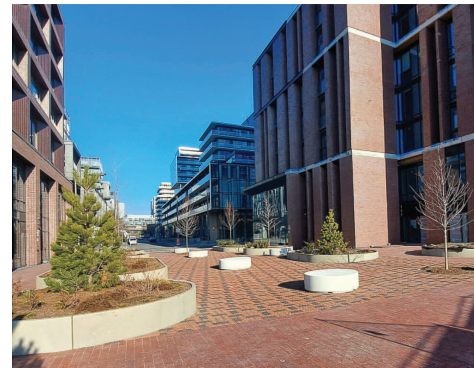
Panorama Residential Building, Ottawa, ON
