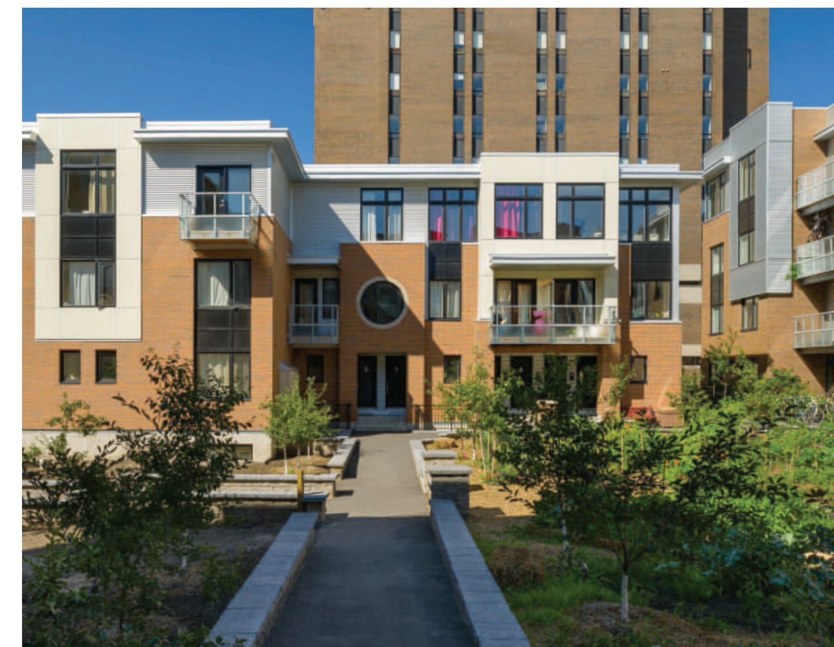
Beaver Barracks Redevelopment, Ottawa, ON
