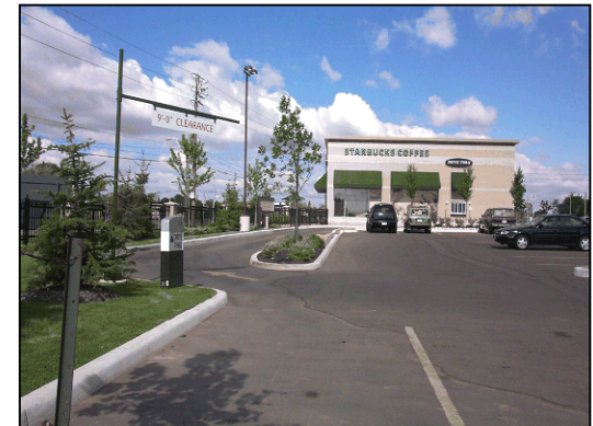
The location of the stacking lane for this Starbucks restaurant on Trafalgar Rd. in Oakville is a good example of how to avoid traffic and pedestrian conflicts, and also allow the building to establish a good street relationship.
