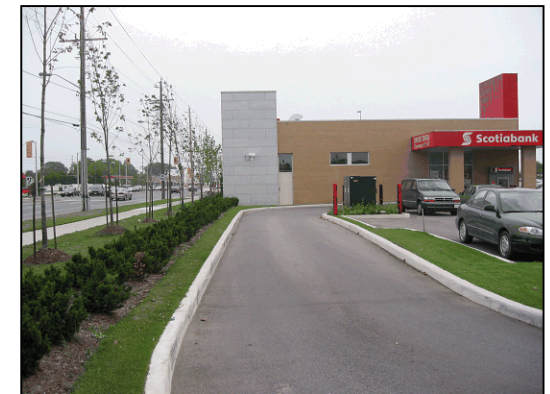
Photograph of the stacking lane leading to the pick up area for the above Scotiabank building. Note the relatively new landscape screen adjacent the driveway.
