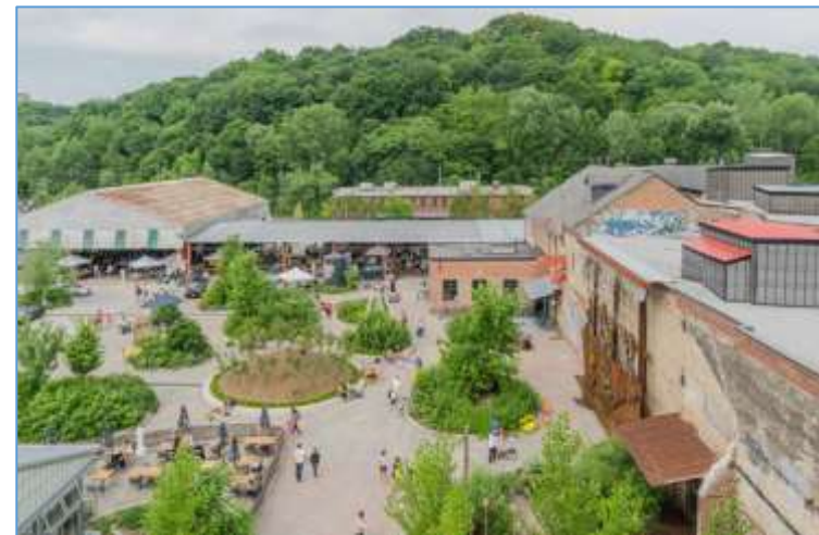
Evergreen Brickworks, Toronto, an example of naturalization within an institutional setting
