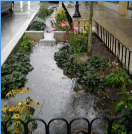
Rain garden to reduce stormwater flow
