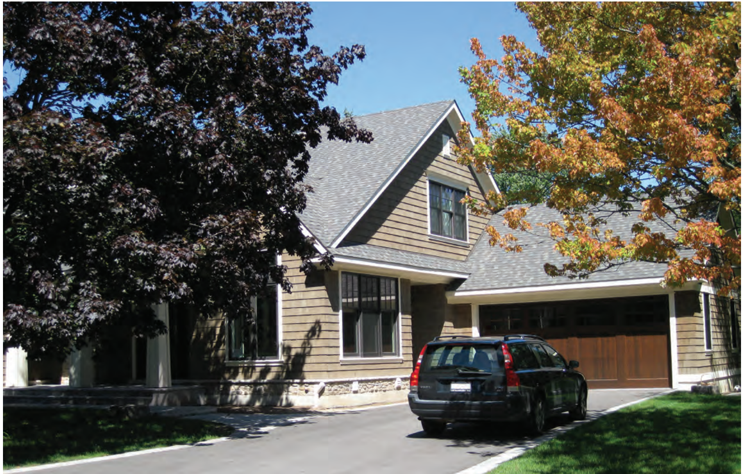
This well-detailed, single-storey attached garage is adequately recessed behind the main façade of the dwelling.
