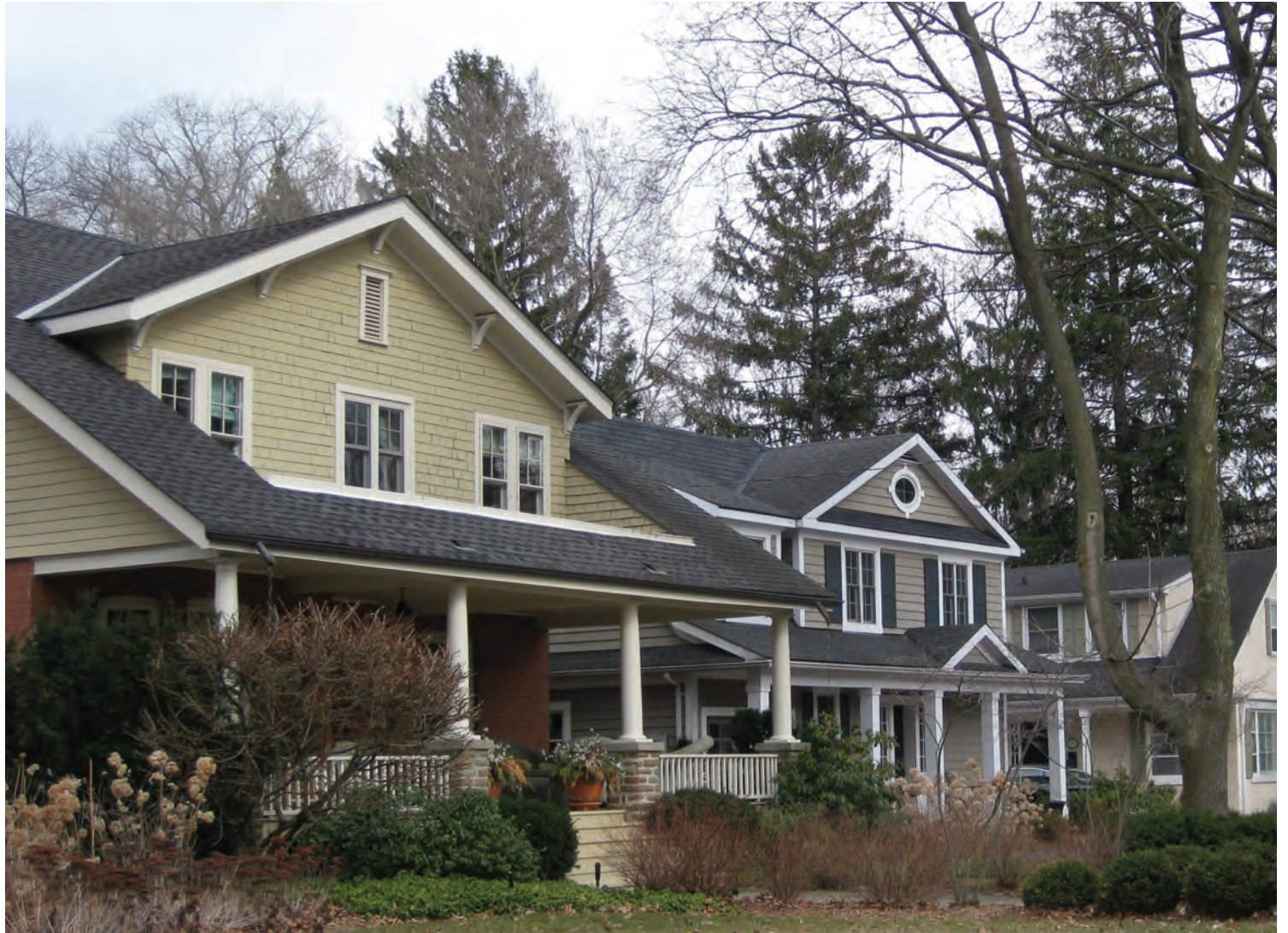
This new dwelling (centre) incorporates many of the patterns and elements of its neighbours – dwelling width, roof forms, window design, covered porch, and building materials.
