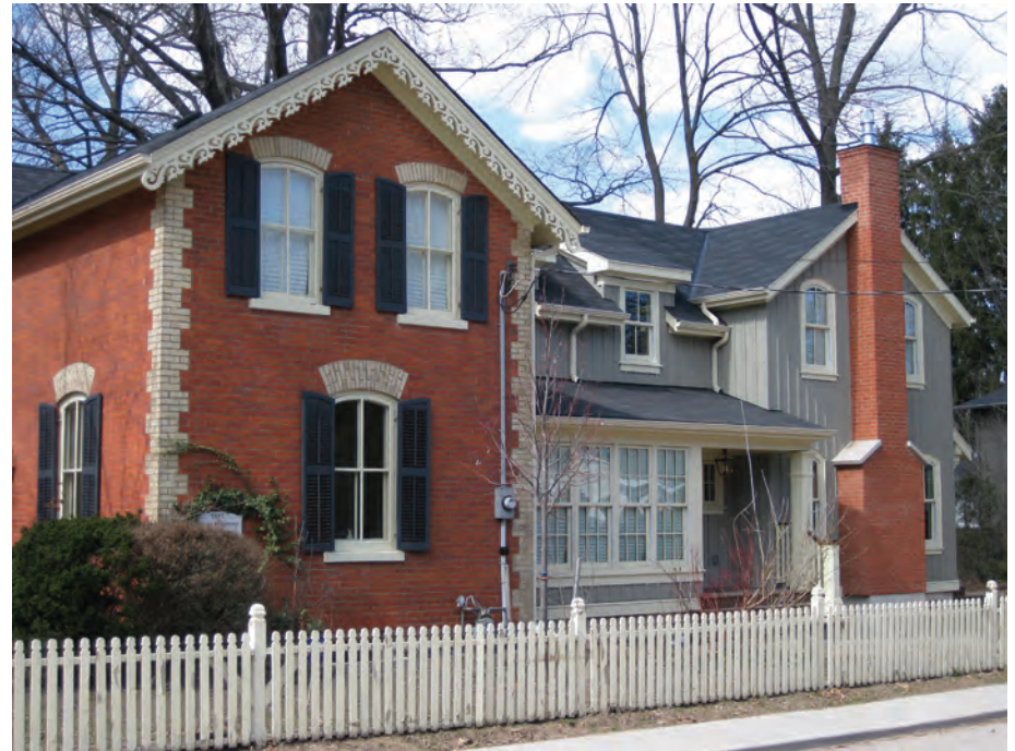
The addition to the heritage dwelling is visually distinct from the original dwelling (left) but incorporates similar architectural details, such as roof slopes and windows.
