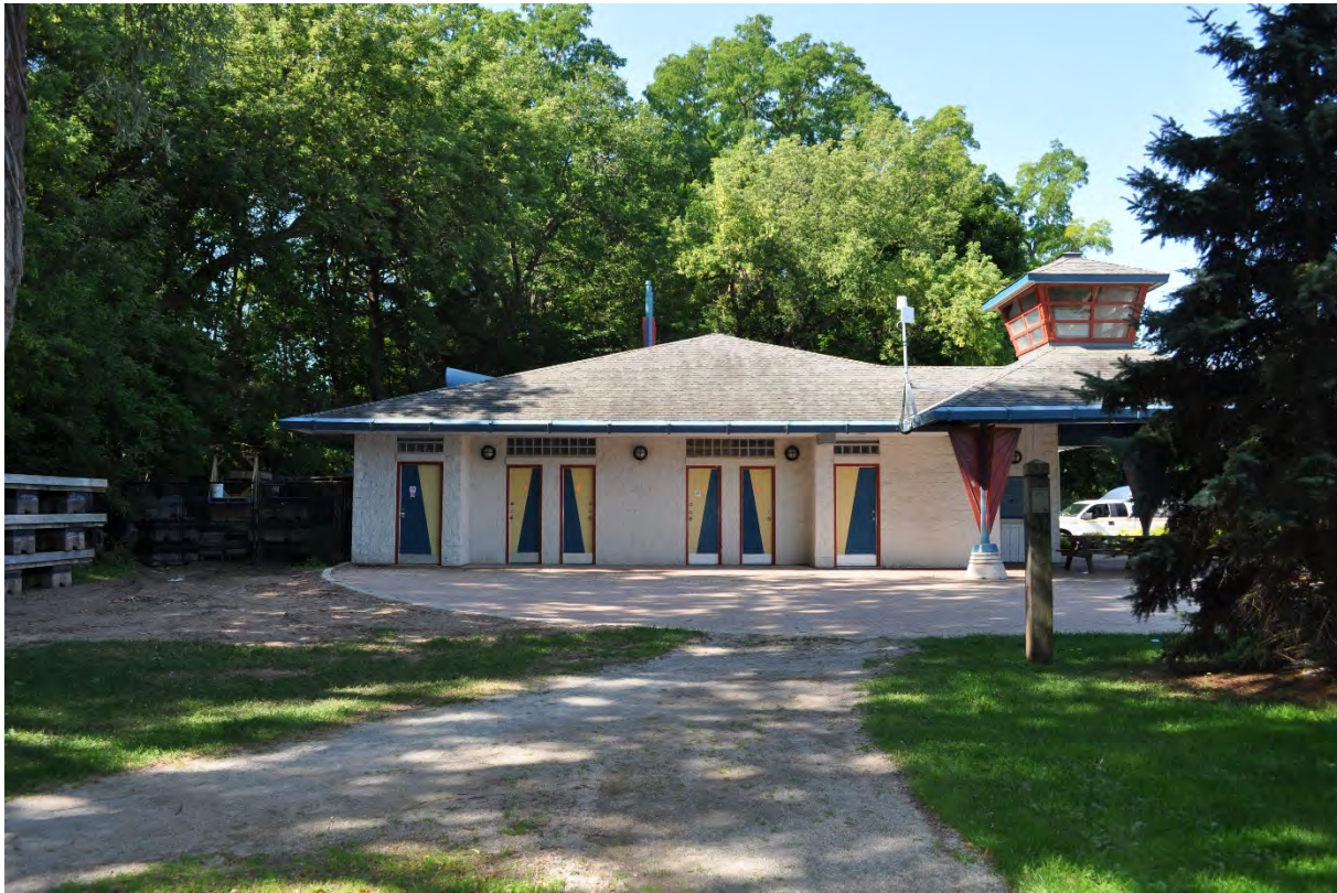
Figure 29: Washroom/Workshop building (CU 2015).
