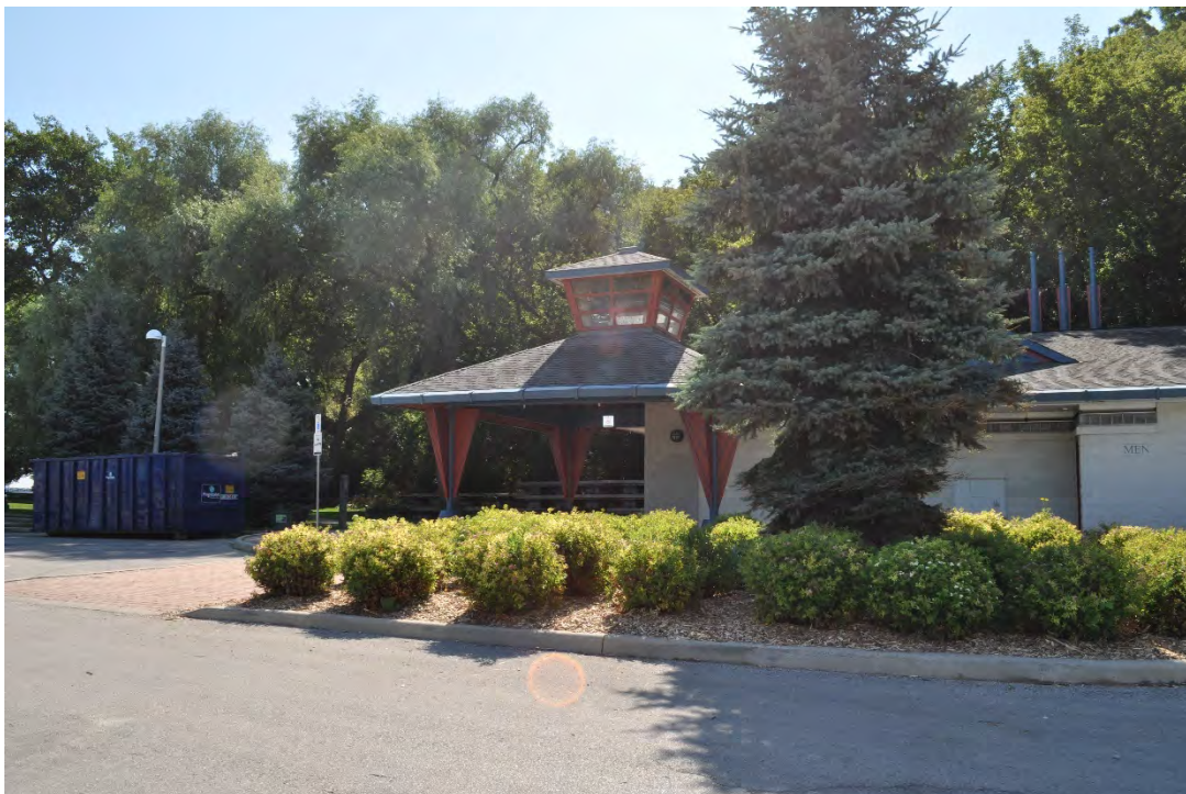
Figure 28: Area around washroom/Workshop building (CU 2015).
