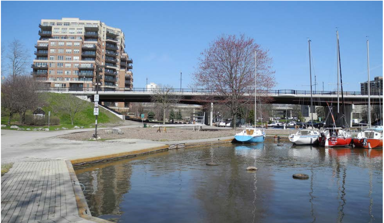
Figure 2-23: The shipyard's original marine railway path has been enlarged over the decades to house a number of moorings in Shipyard Park (CBCollective 2019).
