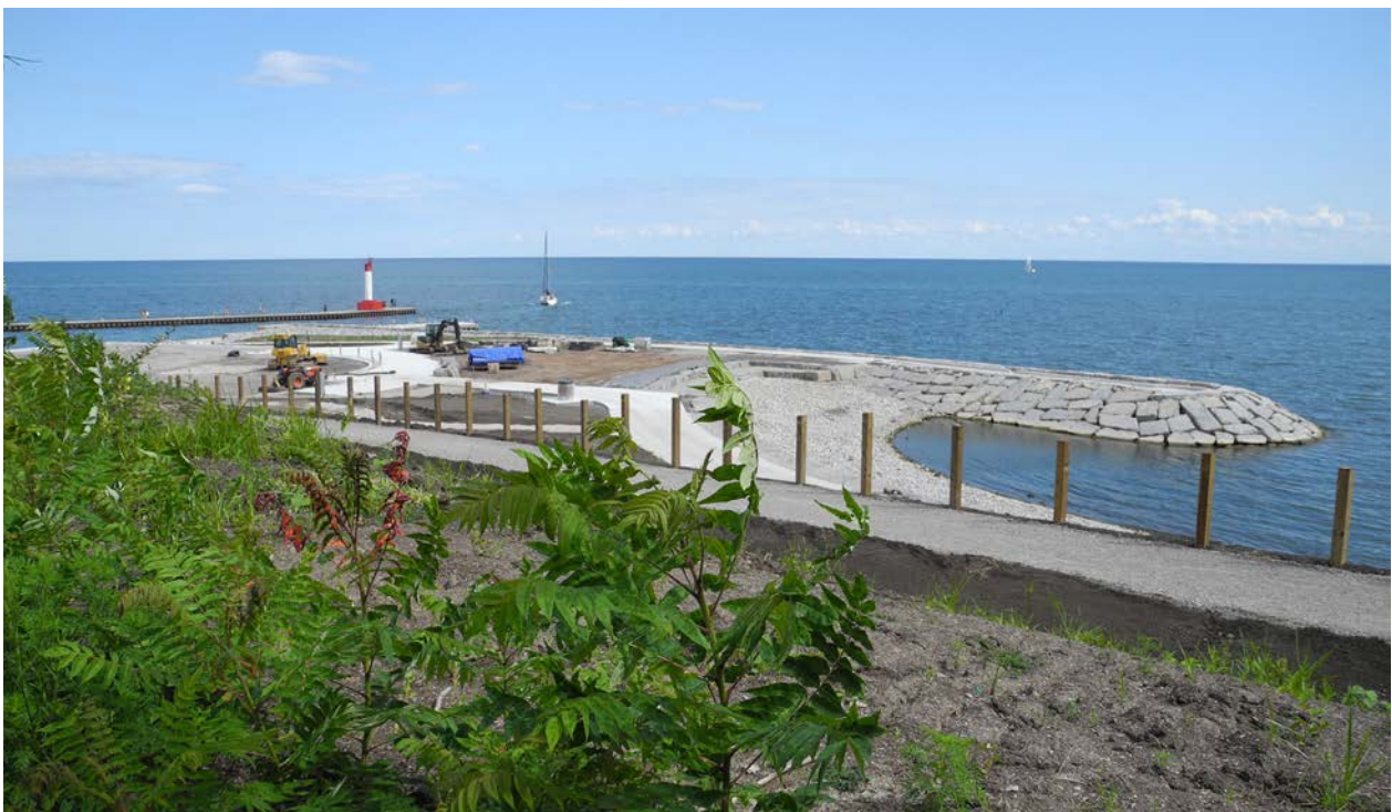
Figure 2-20: Looking south at shoreline engineering currently underway at Tannery Park (CBCollective 2019).
