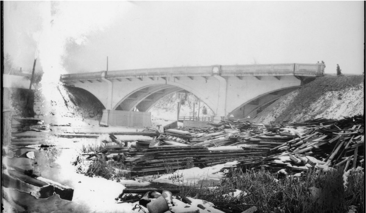
Figure 4-39: The new bridge over Colborne Street under construction in 1924 (COTA).
