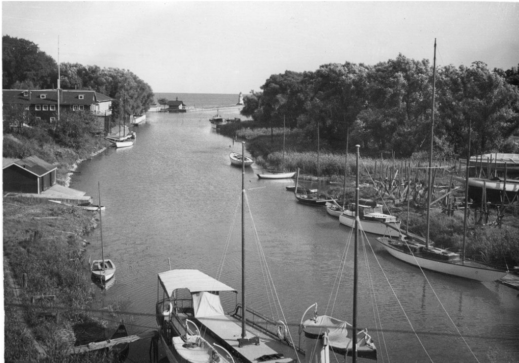
Figure 4-51: 1932 photograph showing the ecology of the peninsular form still intact (COTA).
