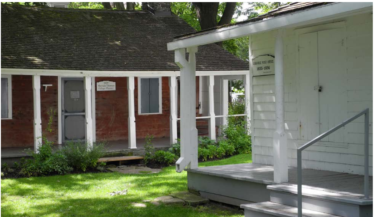
Figure 2-10: The Merrick Thomas House (left) and Post Office Museum (right) form a cluster of heritage resources relocated to Lakeside Park in the 1950s (CBCollective 2019).
