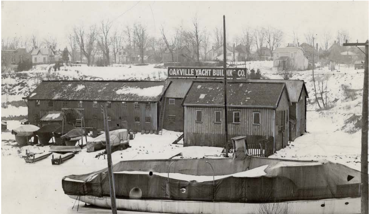
Figure 4-31: Undated photograph showing the Oakville Yacht Building Company's facilities during the winter season (TSPA).
