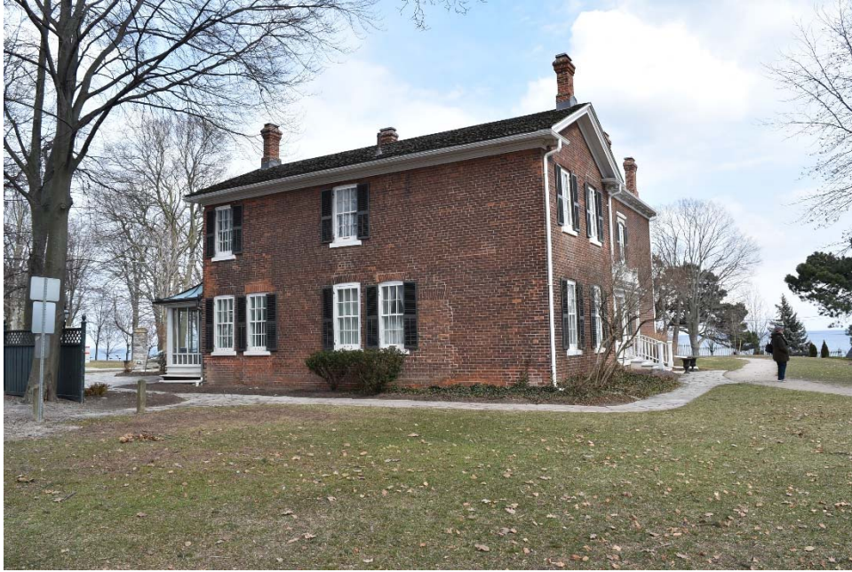
Figure 52: North façade of the c. 1828 Store , and partial west façade.
