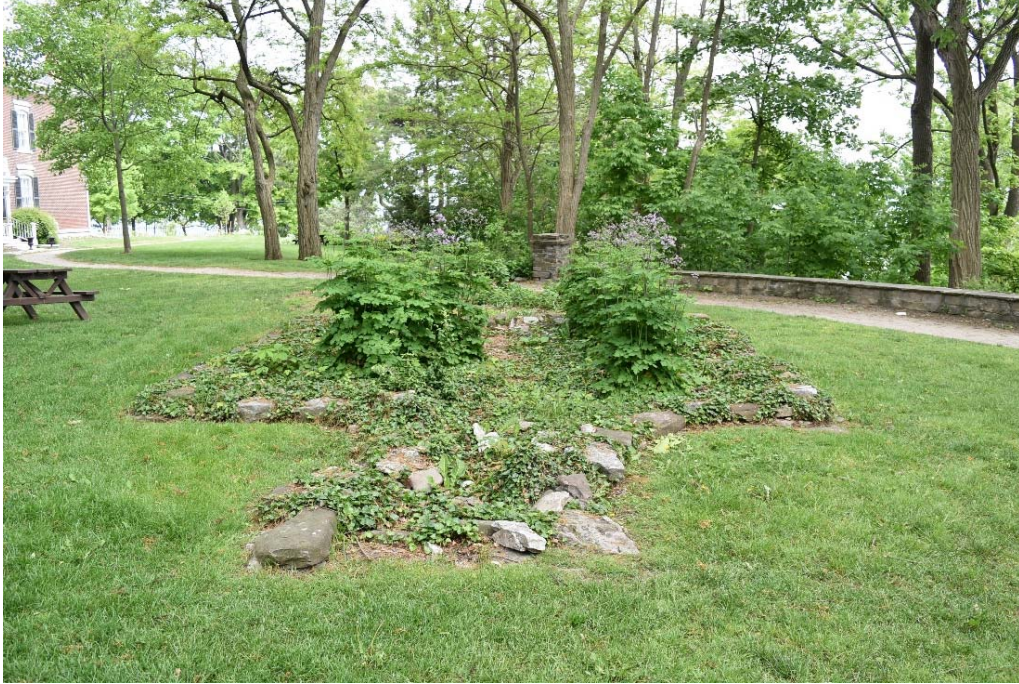
Figure 44: Remnant foundation walls, originally from Capt. Wilson's residence, later repurposed as the foundation of the late 19 th /early 20 th century water tower, June 2018
