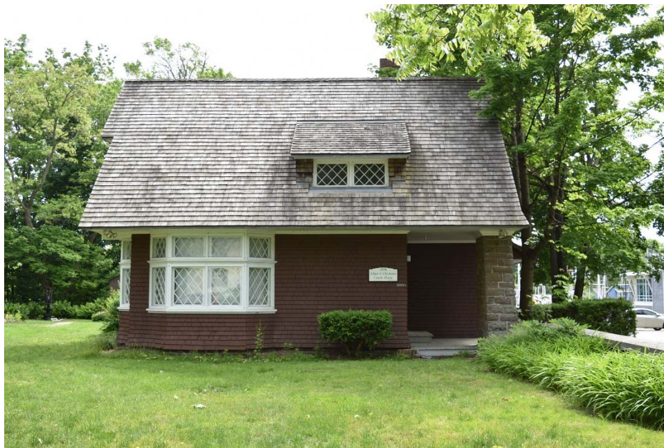
Figure 55: East façade with King Street to the right of the building.
