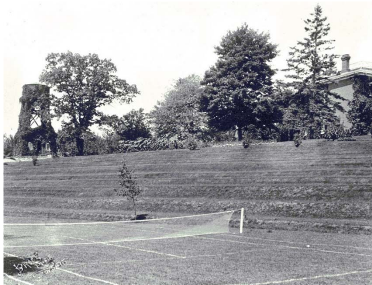
Figure 26: R.K.'s late 19 th century water tower and tennis court 117
