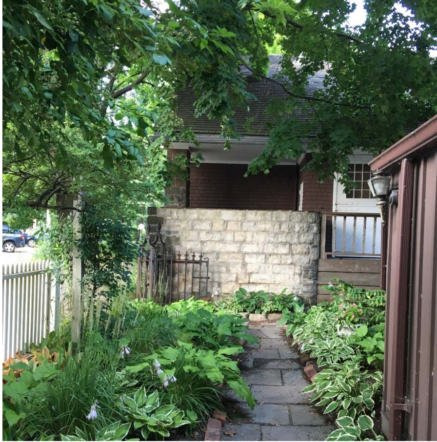
Figure 58: Partial west façade of the Coach House and Gardener's Cottage , showing the manure pit stone wall, the Dutchman door, and the board and batten Cottage walls.
