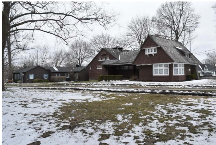
Figure 31: Southeast aspect of the Cottage and the Coach House and Gardener's Cottage
