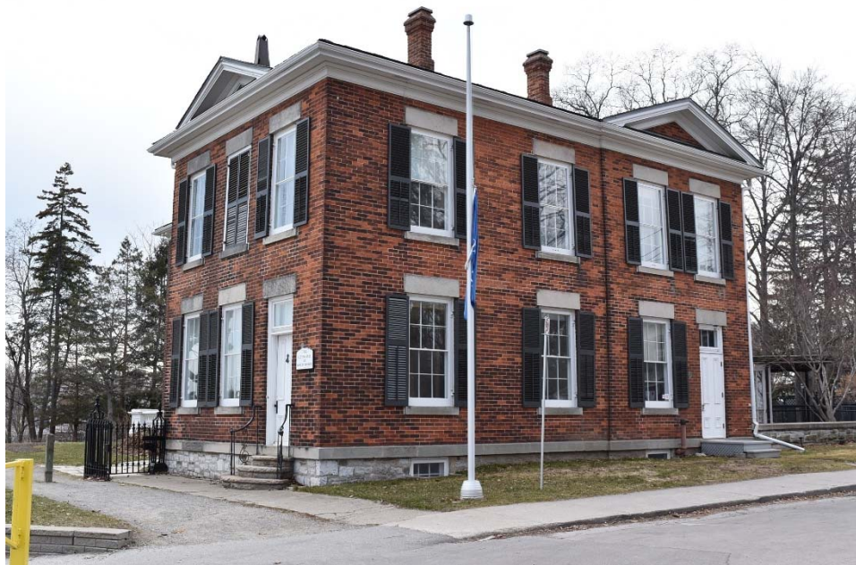
Figure 49: Southeast corner of the Custom House , from Navy Street.
