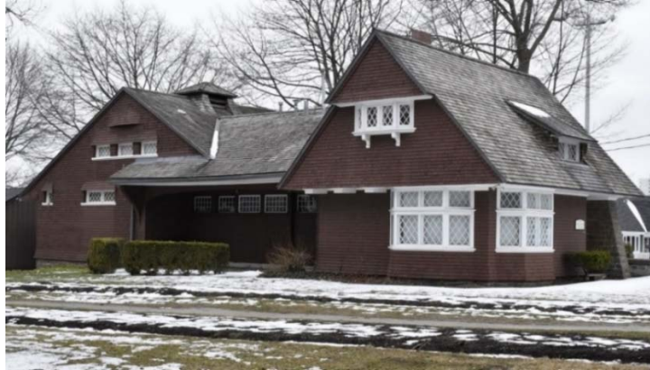
Figure 27: The Coach House and Gardener's Cottage , southeast façade
