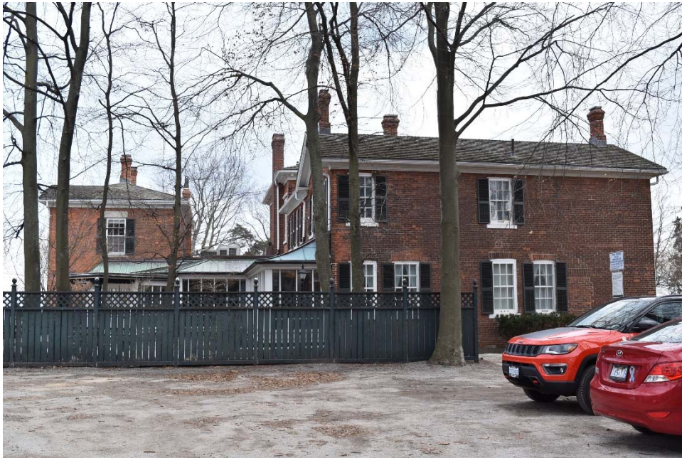
Figure 51: North façade, showing (left to right) the 1856 Custom House , 1983 Museum vestibule, and the c. 1828 Store .
