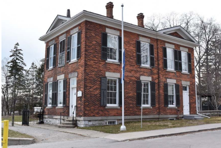
Figure 18: Southeast corner of the Custom House and Bank of Toronto building
