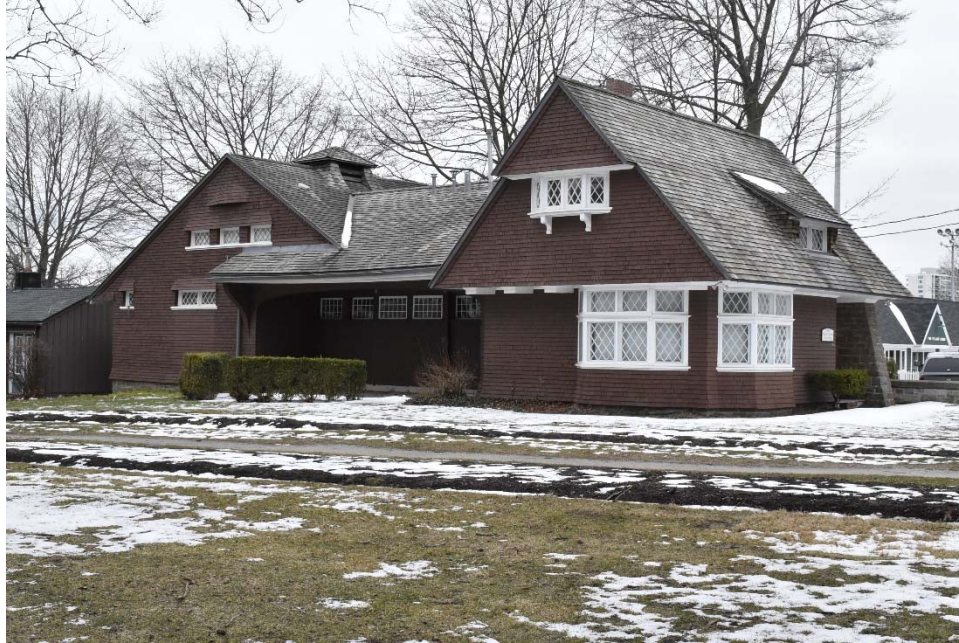
Figure 54: Southeast corner of the Coach House and Gardener's Cottage , showing the south and east elevations.
