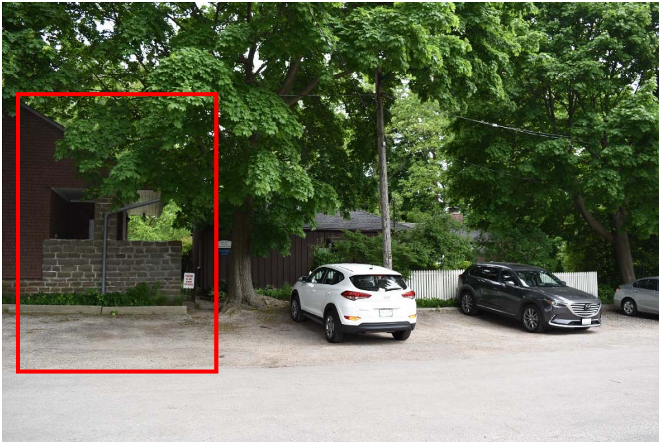
Figure 57: Partial west façade, viewed from the north, including the stone wall of the former manure pit of the Coach House and Gardener's Cottage . The east wall of the Cottage is visible to the right of the Coach House and Gardener's Cottage .
