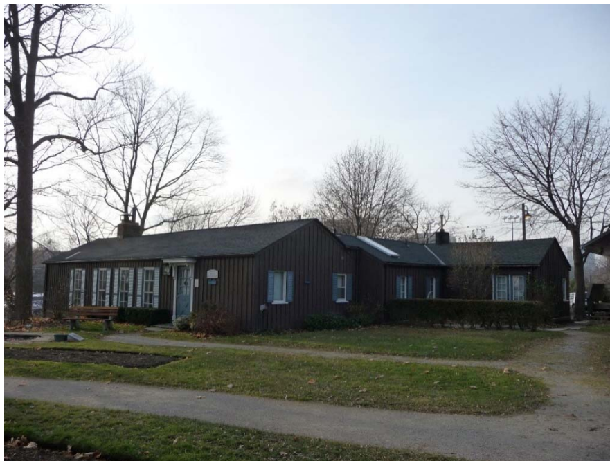
Figure 61: Southeast façade, December 2008
