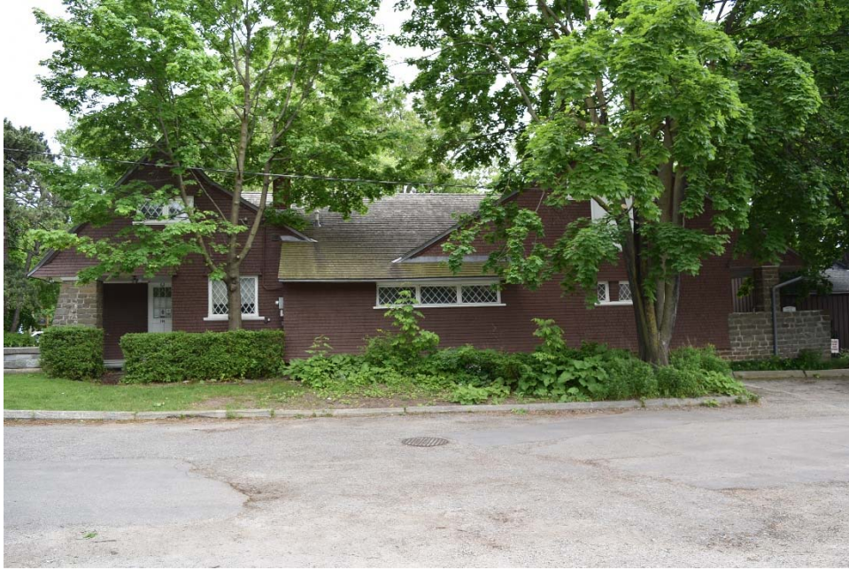
Figure 56: North façade, from King Street.
