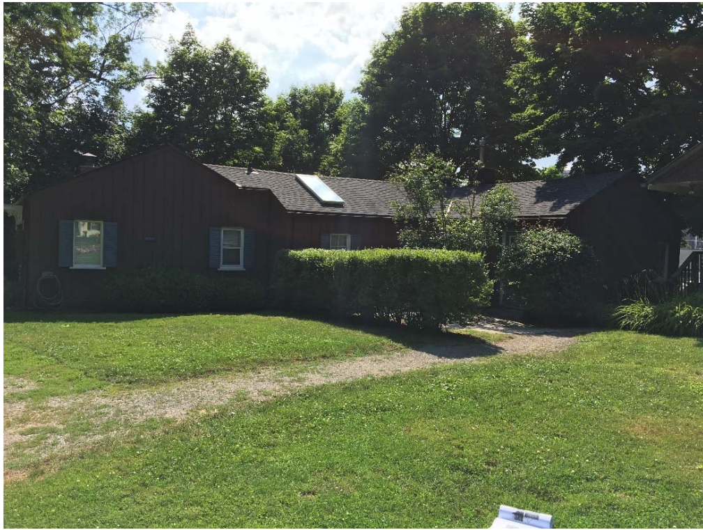
Figure 62: East façade, July 2018
