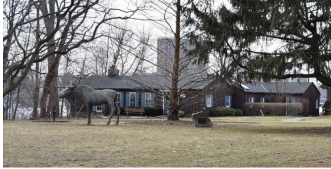
Figure 33: South façade of the 1952 Cottage
