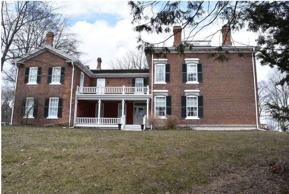
Figure 53: West façade showing (left to right) the c. 1828 Store and 1½ storey addition, and the 1858 2-storey addition.
