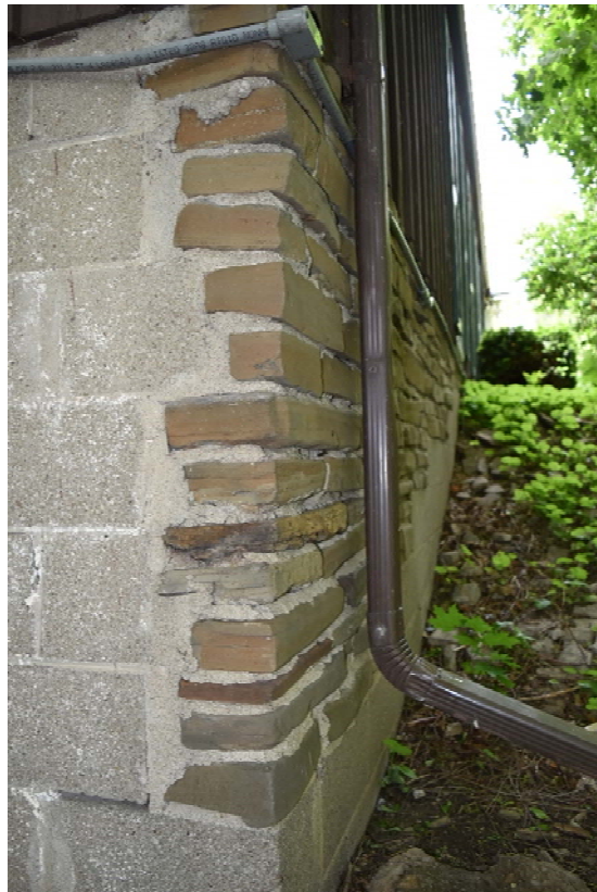
Figure 65: Southwest corner, facing east
