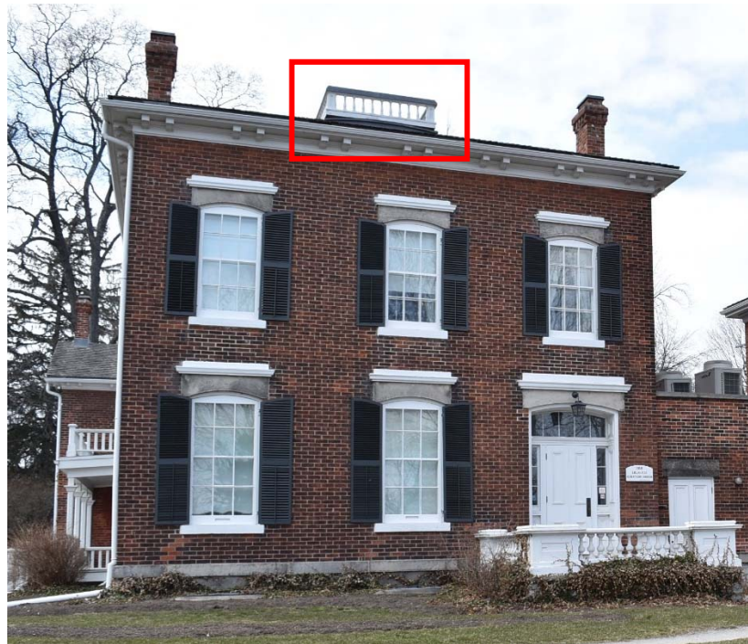
Figure 17: Restored widow's walk on 1858 addition.
