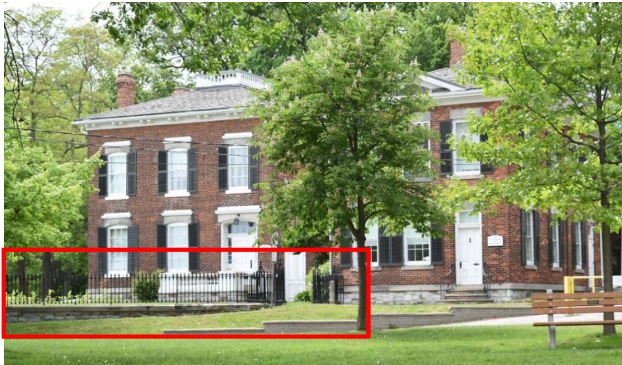
Figure 36: Stone and metal fence detail, June 2018
