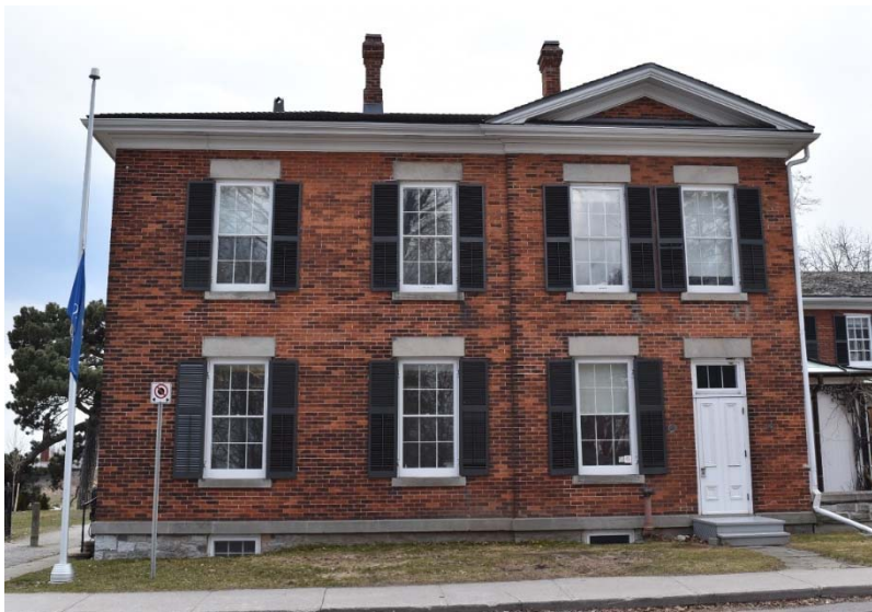
Figure 19: East façade of the Custom House and Bank of Toronto building
