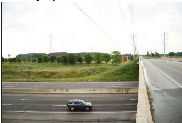
Plate 23: South view along east side of Sixth Line from Highway 407 bridge.
