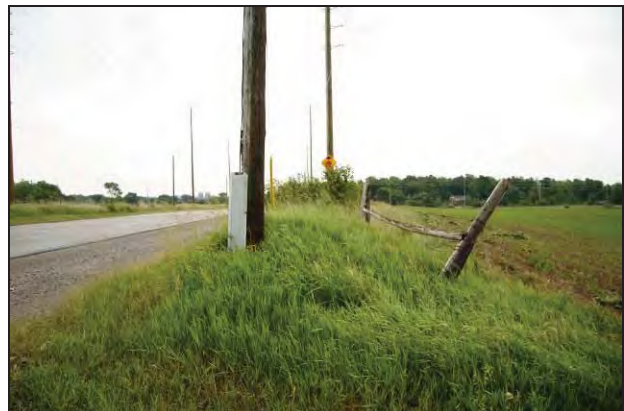
Plate 18: South view along west side of Sixth Line showing communications boxes at edge of ROW.
