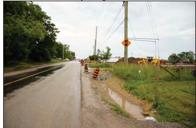
Plate 4: South view of disturbed ditch and ongoing construction beyond ROW.
