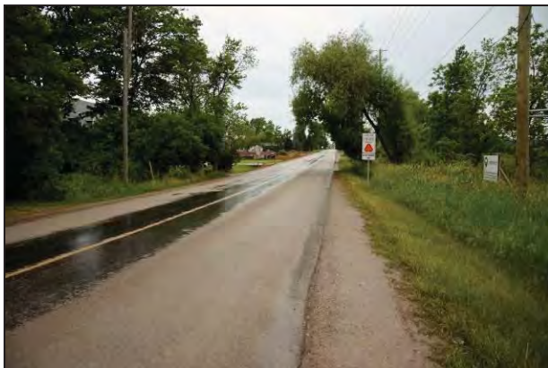
Plate 5: North view along east side of Sixth Line.
