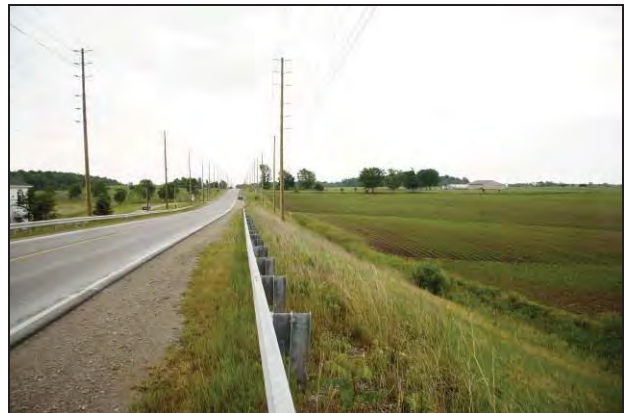
Plate 22: South view along west side of Sixth Line from Highway 407 bridge.
