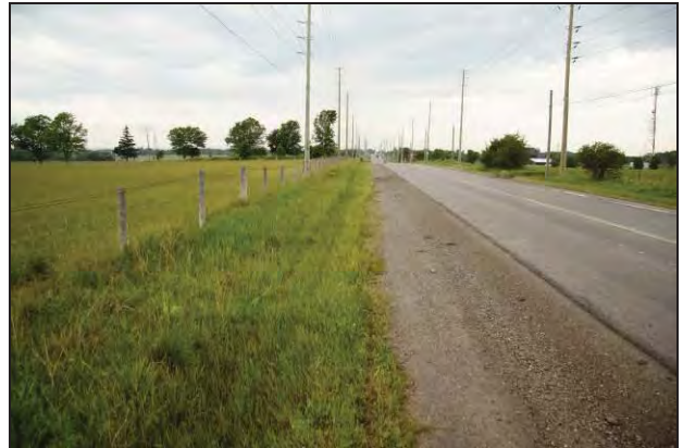
Plate 20: North view along west side of Sixth Line.
