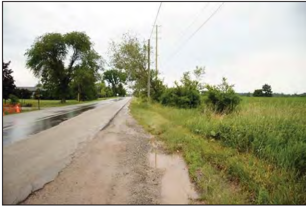
Plate 7: North view along east side of Sixth Line.
