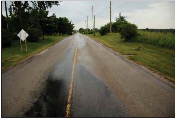
Plate 9: North view along Sixth Line showing ditching and road cut within ROW.
