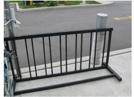
Wheel-only supportive bicycle racks are not permitted.
