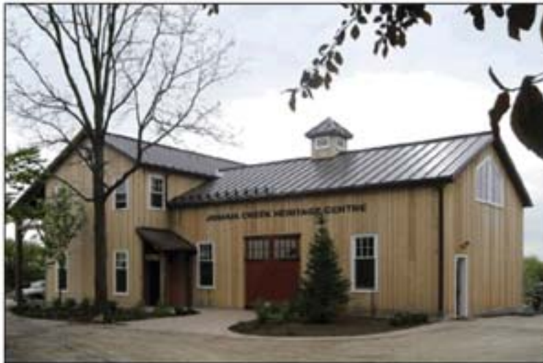
Barn adapted and expanded for use as an art gallery and cultural centre, Oakville, Ontario. Source: www.joshuacreekheritagecentre.ca
