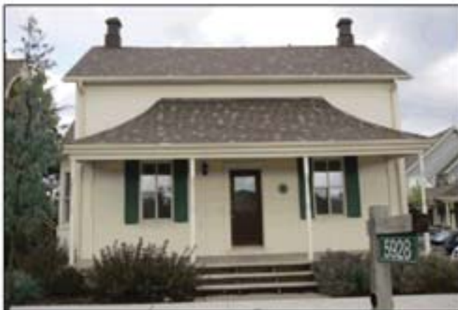
House Relocated within Site and Restored.
