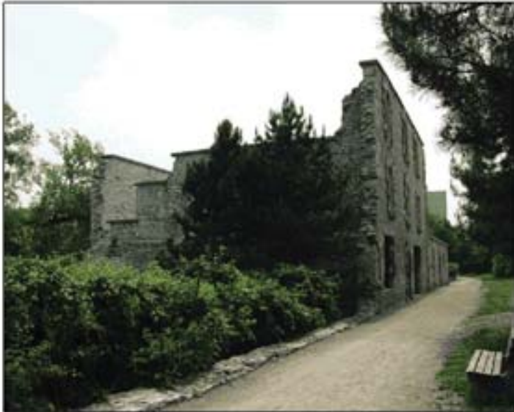
Mill ruins preserved within new public park, Guelph, Ontario. Source: www.flickr.com
