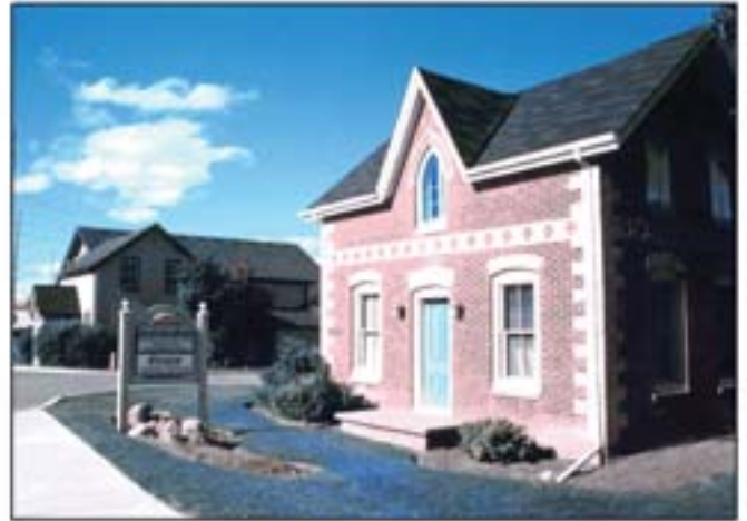
Farmhouse used as medical offices on a main street.
