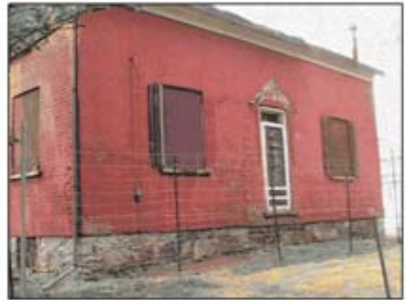
2) High fence erected close to the structure
