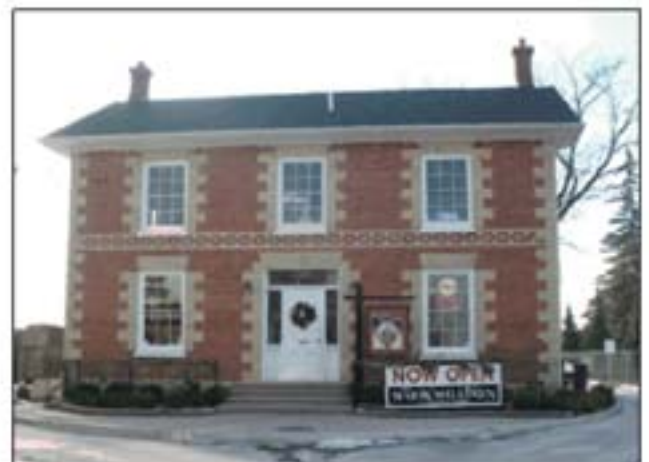
Farmhouse used as restaurant in a new commercial development.
