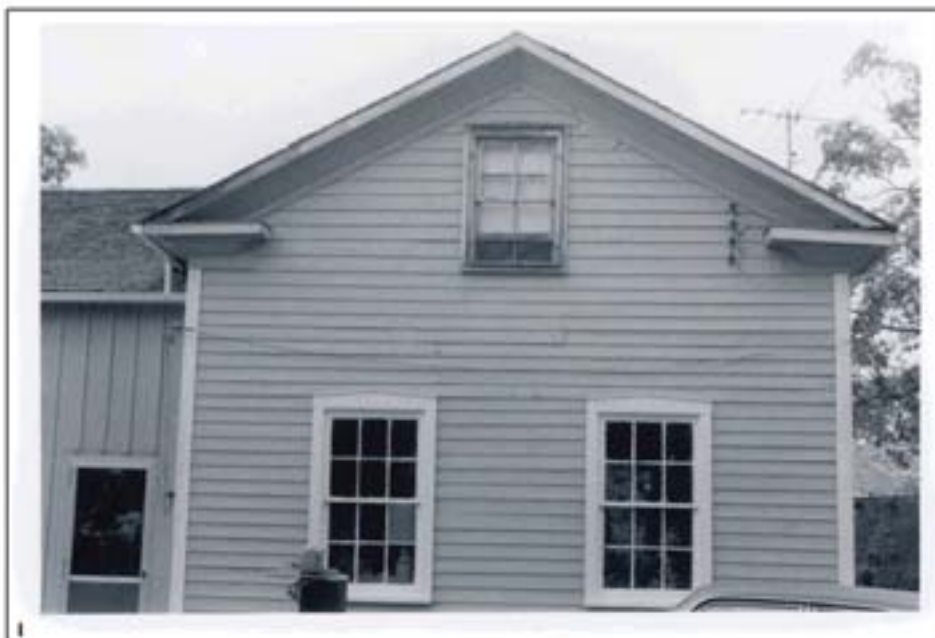
Former farmhouse at 4116 Fourth Line, 1977. The house was demolished for the construction of the 407 West extension.
