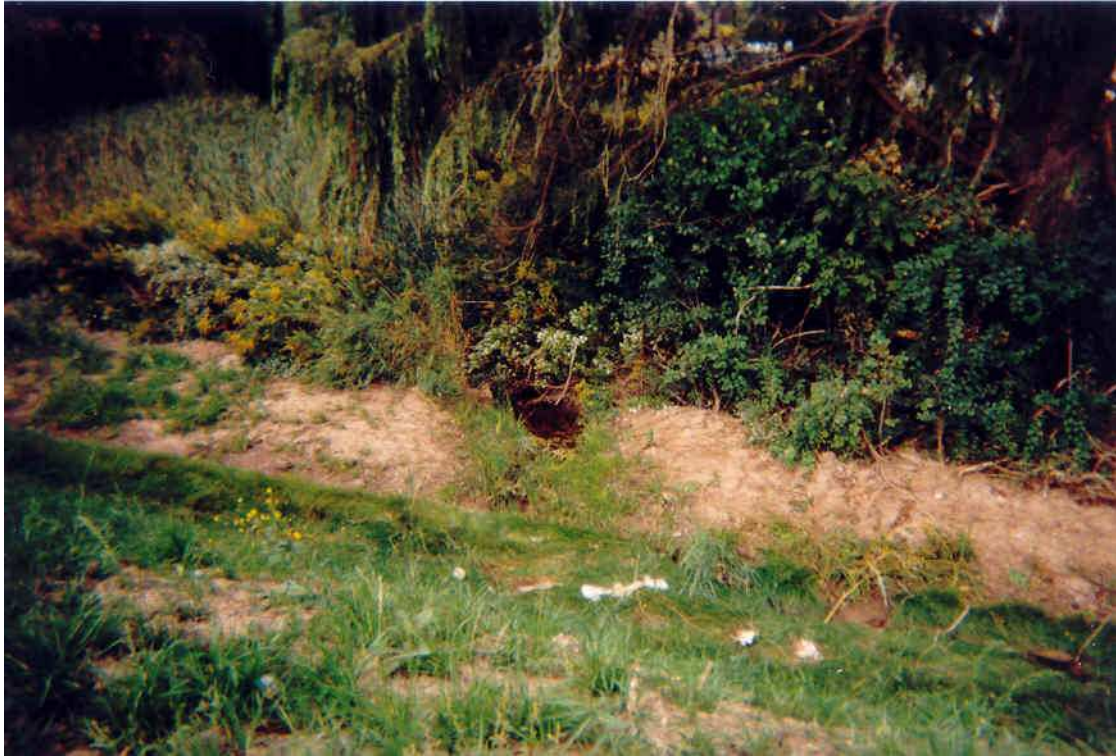
Photo 1. Reach JC-31 looking upstream from Dundas ditch.
