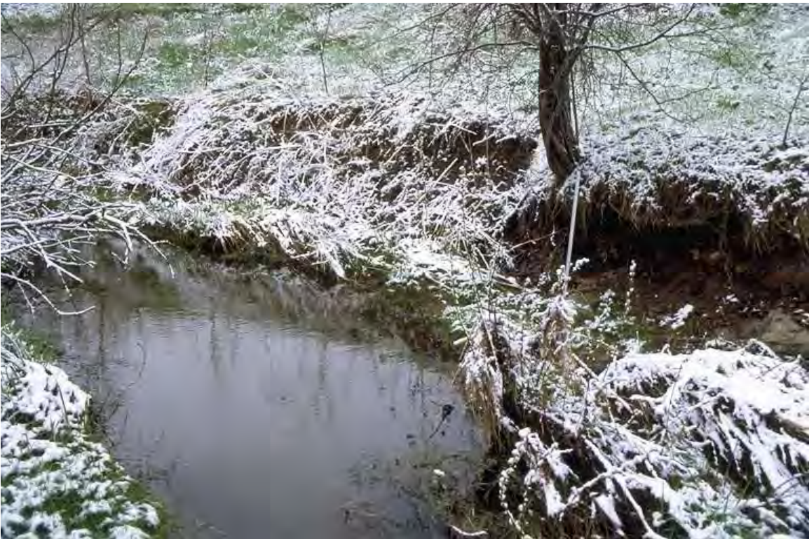
Photo 2. Reach JC-1 at bank erosion.
