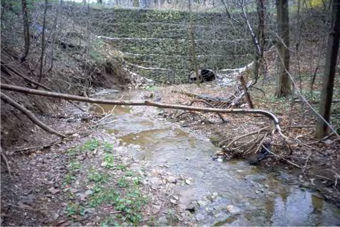
Photo 3. Reach SMA-2 at culvert.
