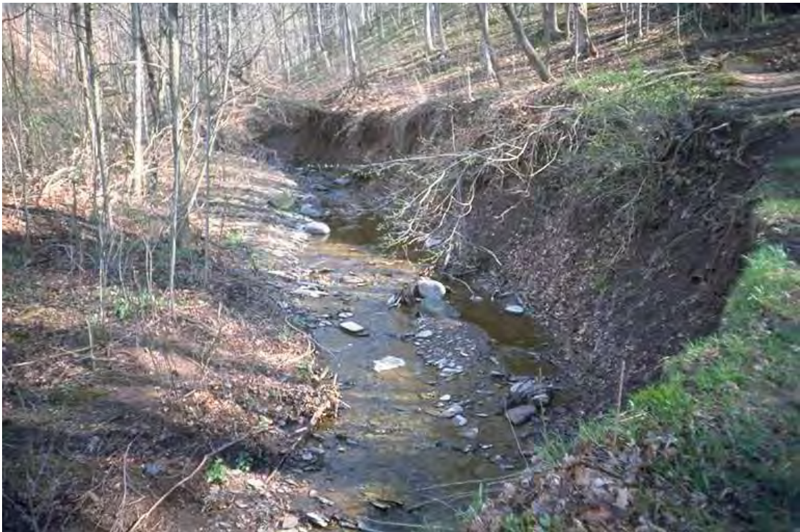
Photo 2. Reach SMA-1 valley wall contact.
