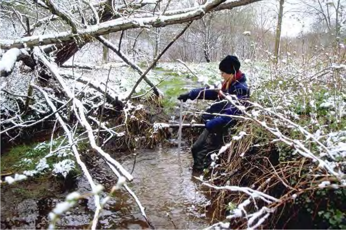
Photo 1. Reach JC-3 at bank erosion.
