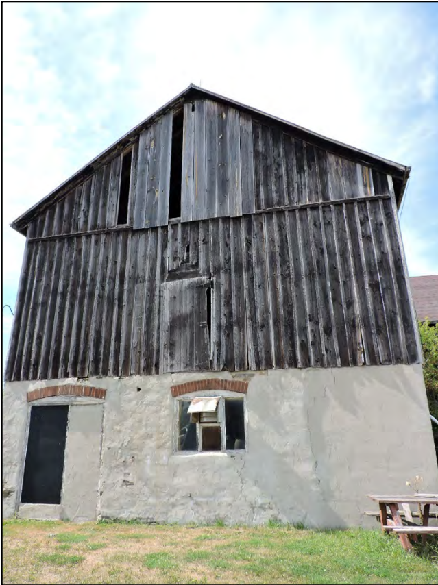
Figure 19: Bank barn, south façade (AB, 2016).
