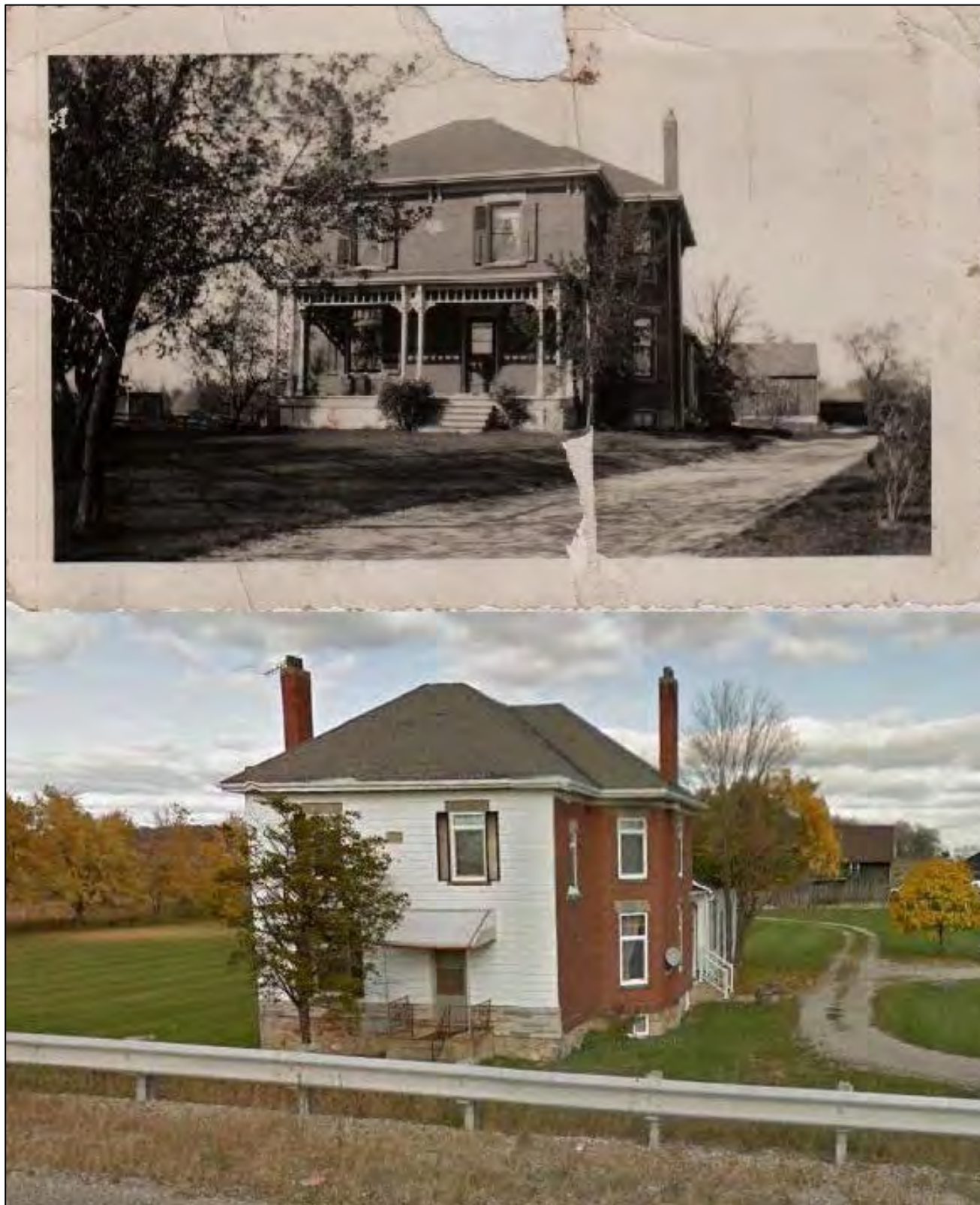
Figure 38: Alterations to the front façade of the residence Top: photograph found in attic at 4243 Sixth Line likely taken mid-20 th century (Provided by C. Schulz, 2016), bottom: Google Streetview, 2016.
