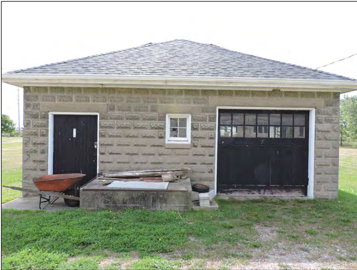
Figure 27: Workshop (former milk house) showing the garage door and rusticated stone exterior, east façade (AB, 2016).
