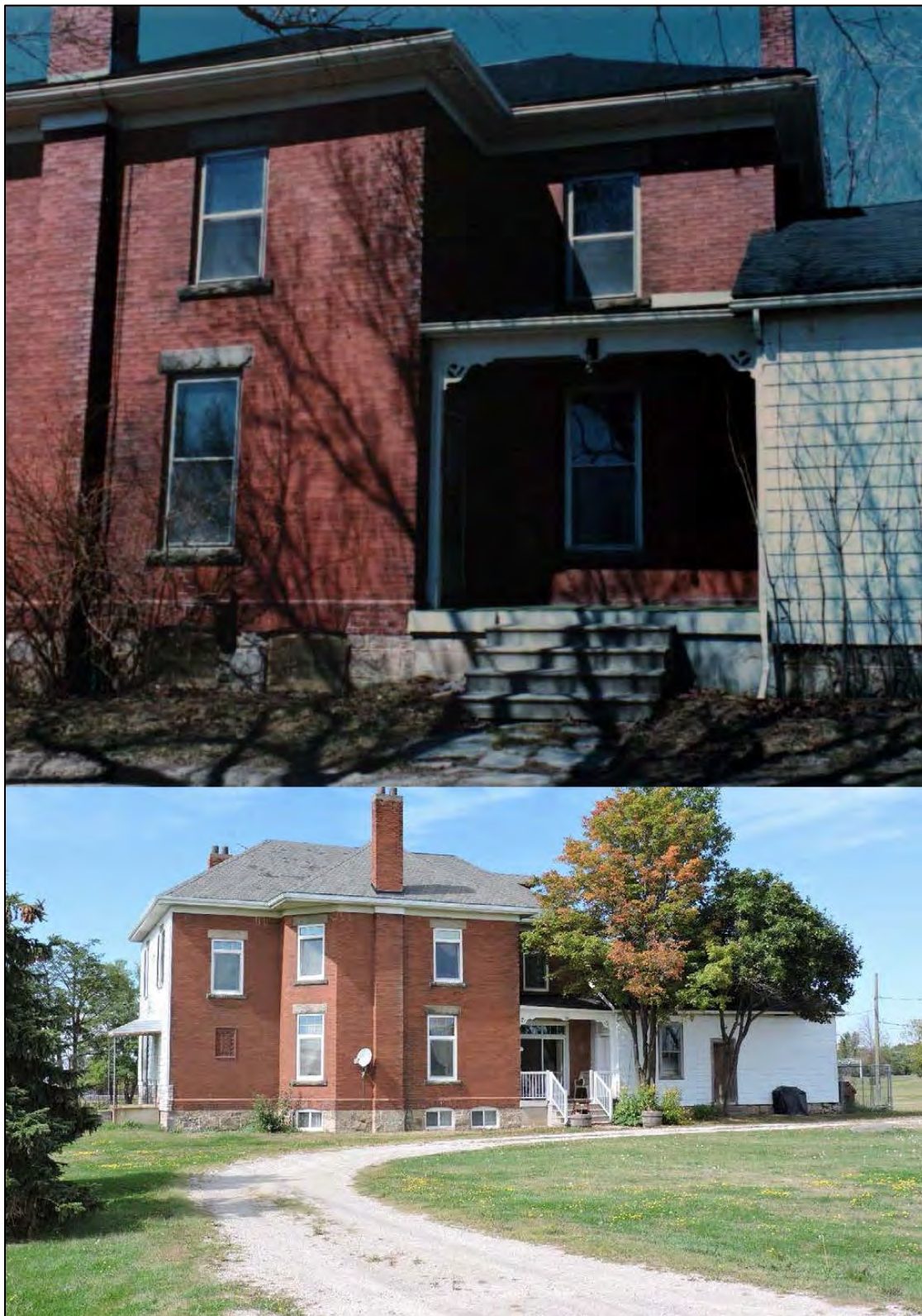
Figure 39: Images of side (south) façade of residence. Top: Schultz family c.1980 (Provided by C. Schulz, 2016); bottom: photograph showing current sliding door entrance along south façade and ghosting from cornice brackets below eaves (AB, 2015).
