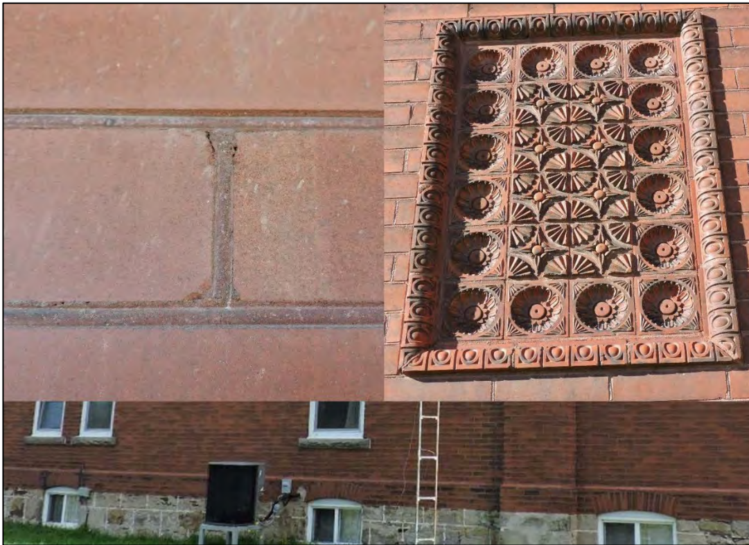
Figure 13: Detail of decorative brick elements (AB, 2016).
