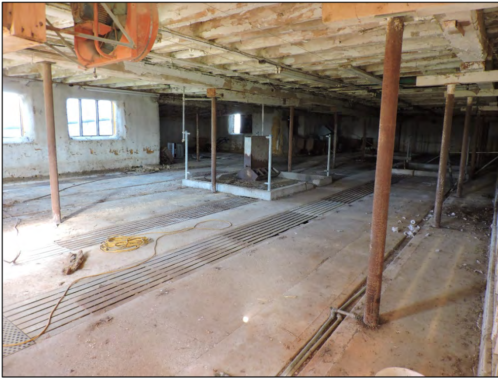
Figure 21: Interior of the lower level of the bank barn tail (AB, 2016).
