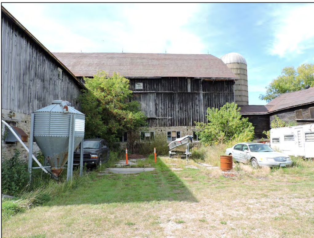
Figure 18: Bank barn, south façade (AB, 2016).
