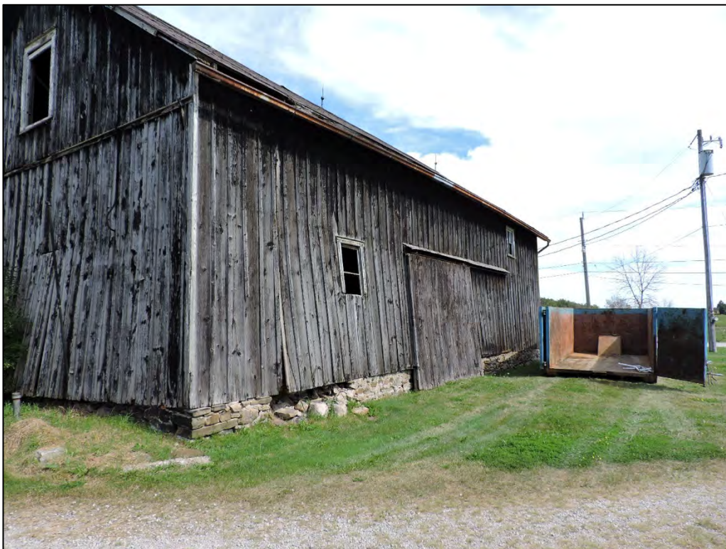
Figure 25: Drive shed, west façade (AB, 2016).
