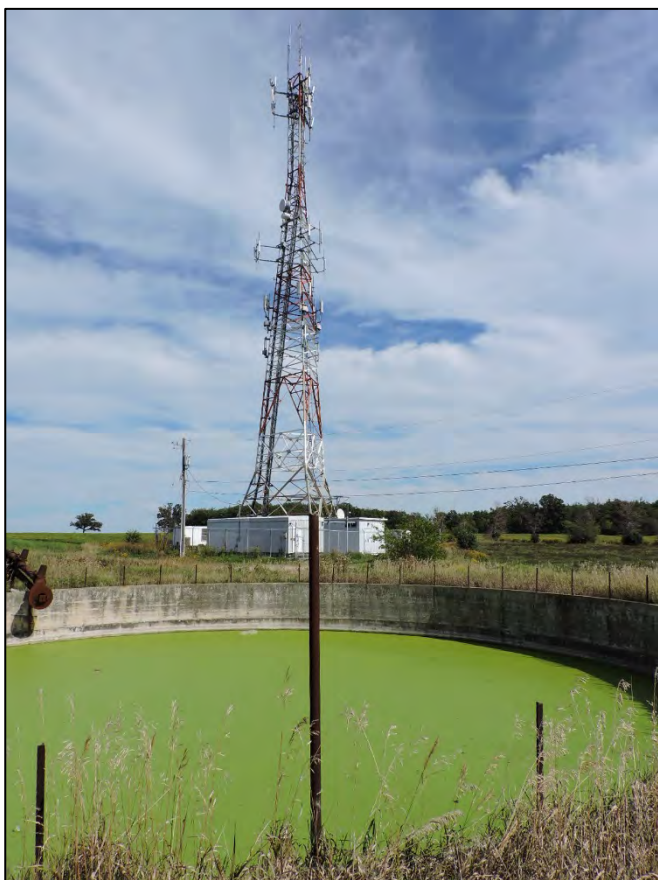
Figure 9: Cell tower and concrete waste holding area (AB, 2016).
