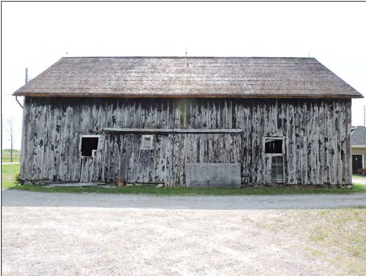
Figure 23: Drive shed, east façade (AB, 2016).
