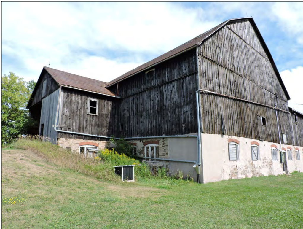
Figure 15: Bank barn, north and west facades of the barn (AB, 2016).
