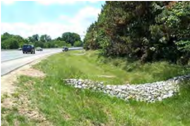
Figure 5.2 Enhanced Grass Swale (Low Impact Development Stormwater Management Planning and Design Guide, Version 1.0, CVC and TRCA, 2010)
