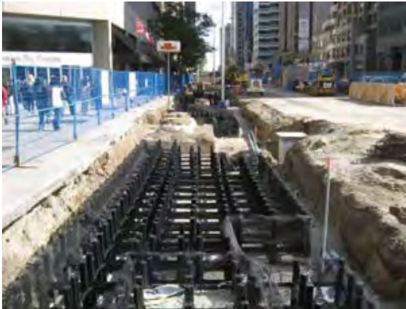
Figure 5.6 Silva Cell Construction (www.smartcitiesdive.com, 2020)
