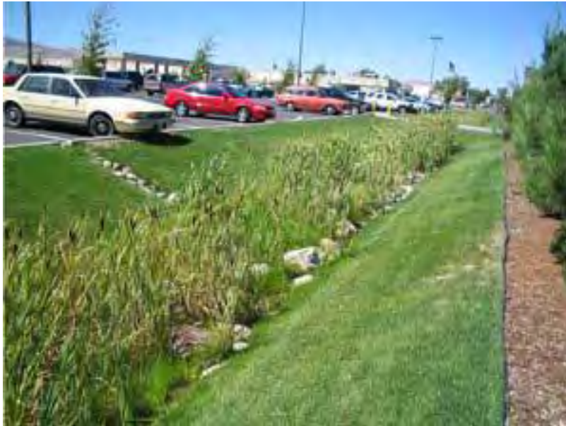
Figure 5.1 Enhanced Grass Swale (Low Impact Development Stormwater Management Planning and Design Guide, Version 1.0, CVC and TRCA, 2010)
