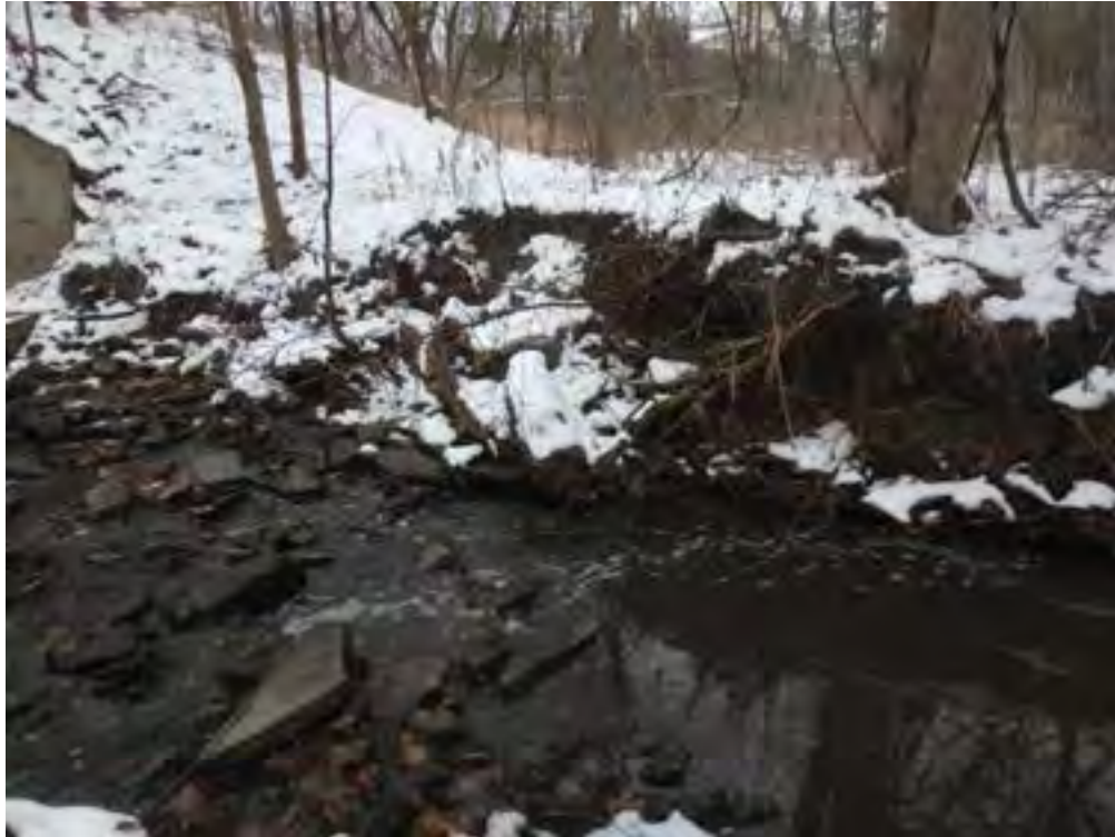
Photo 5: Erosion evident at east bank immediately downstream of Rebecca Street retaining wall. Area spans approximately 10.3 m in length. Height of erosion averages at 1 meter.
