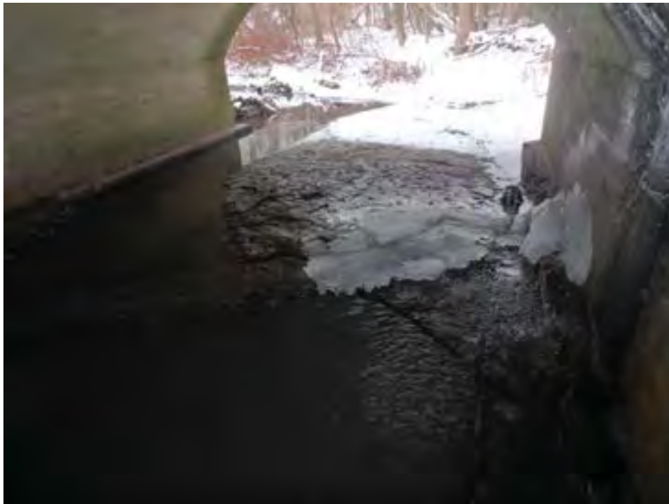
Photo 14: Standing within Lakeshore Road ROW facing upstream. Note large area of limestone present to right (east) of structure inlet. Cement slab located at left may pose a potential barrier to smaller-bodied fish during periods of high flow.
