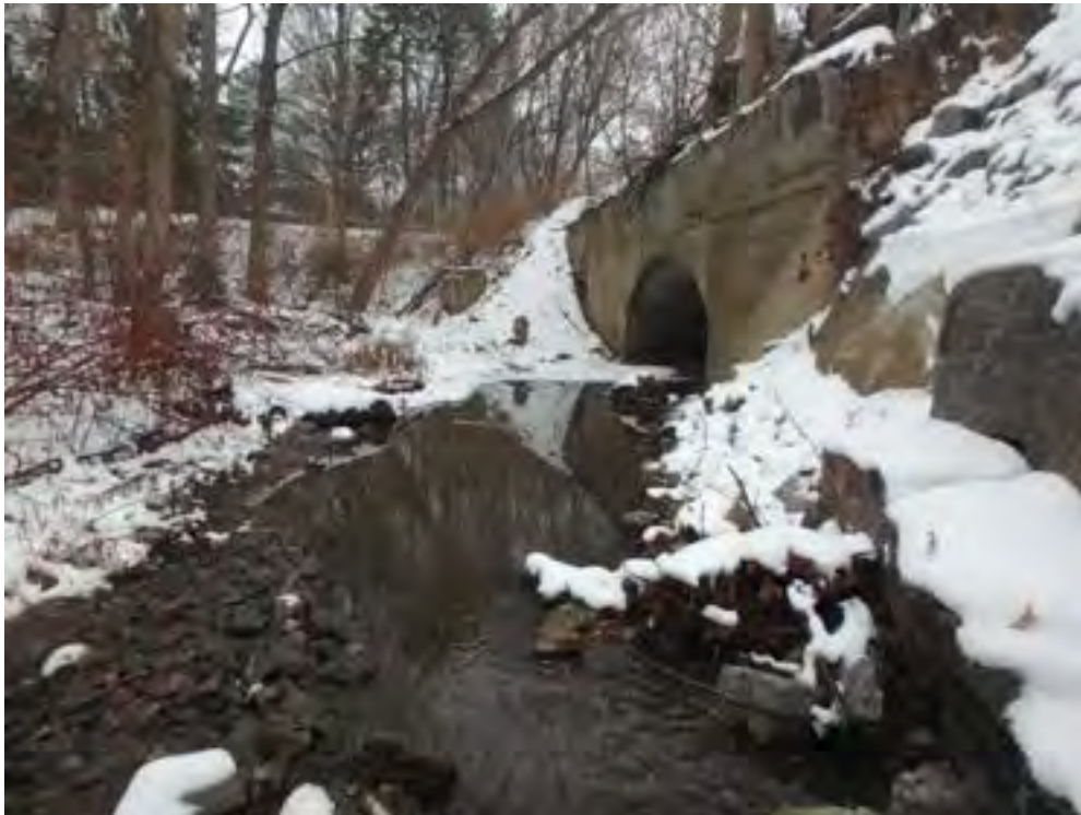
Photo 13: Upstream end of Lakeshore Road crossing. Note some erosion is also evident at northeast bank, where exposed sandy soils are present.
