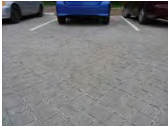
Figure 5.8 Permeable Pavers (Low Impact Development Stormwater Management Planning and Design Guide, Version 1.0, CVC and TRCA, 2010)
