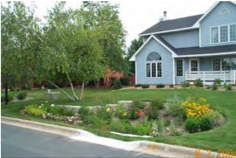
Figure 5.4 Bioretention Facility (Low Impact Development Stormwater Management Planning and Design Guide, Version 1.0, CVC and TRCA, 2010)
