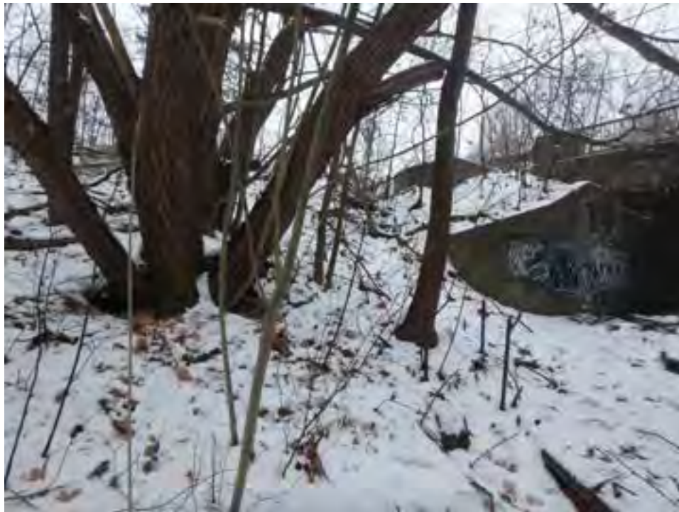
Photo 3: Photo of stable west bank at Rebecca Street.
